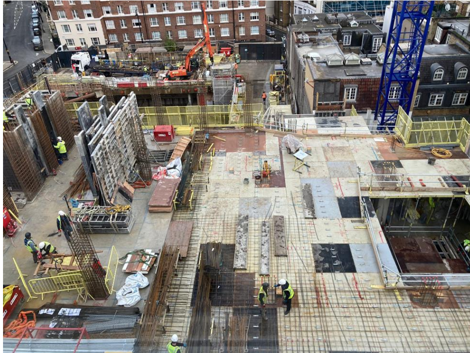
ZONE 1 LEVEL 2 SUPERSTRUCTURE
