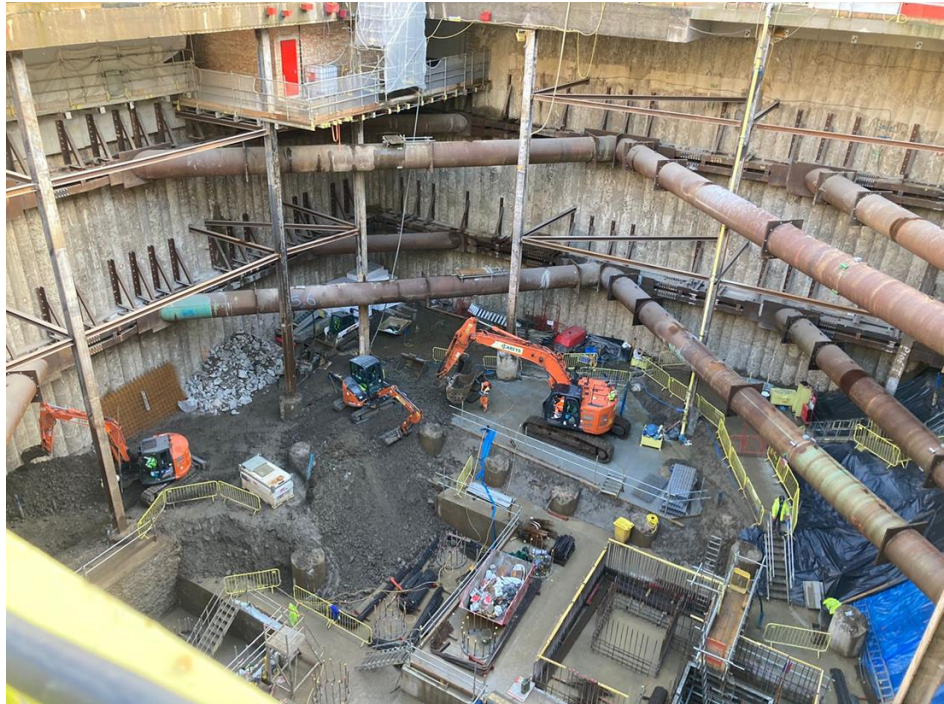
ZONE 2 LEVEL 2 BASEMENT SUBSTRUCTURE
