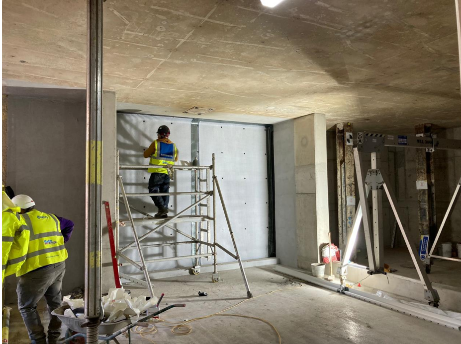
ZONE 1 BASEMENT WATERPROOFING
