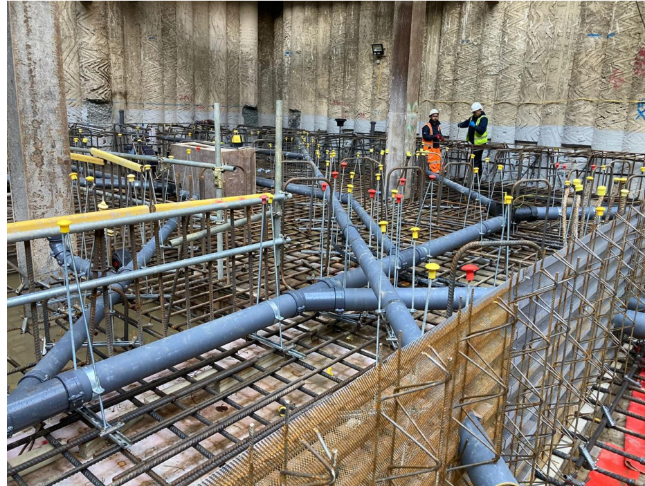
ZONE 2 LEVEL 2 BASEMENT DRAINAGE
