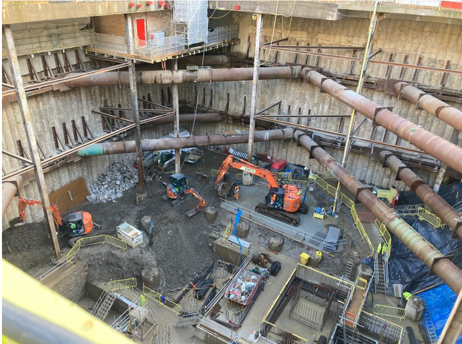
ZONE 2 LEVEL 2 BASEMENT SUBSTRUCTURE
