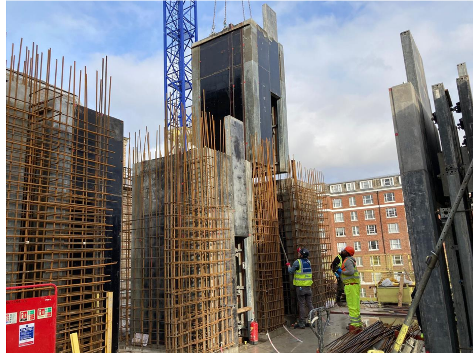
ZONE 1 LEVEL 2 SUPERSTRUCTURE VERTICALS
