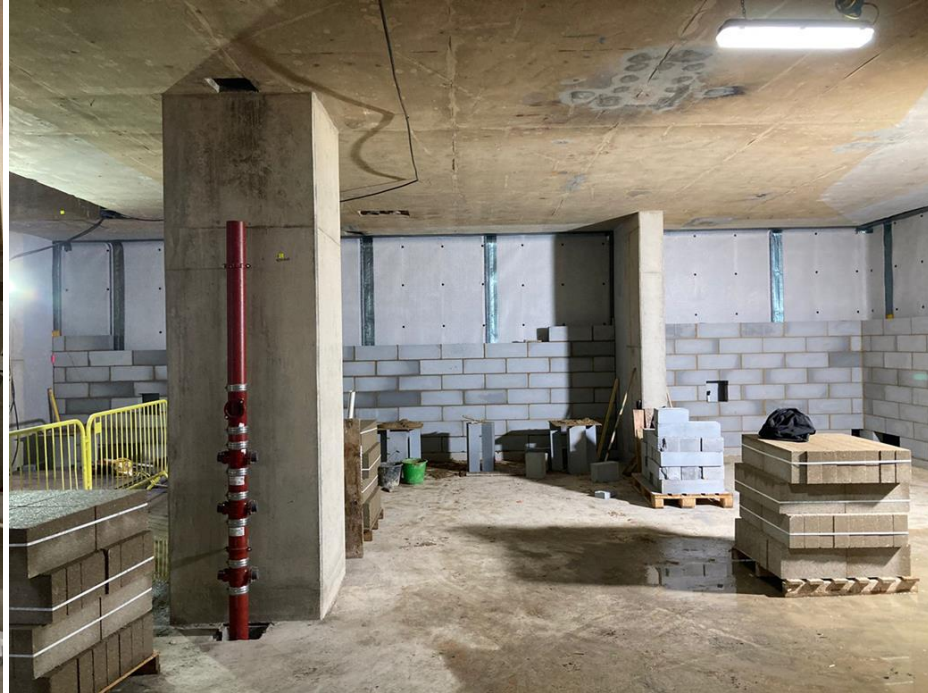
ZONE 1 BASEMENT BLOCKWORK
