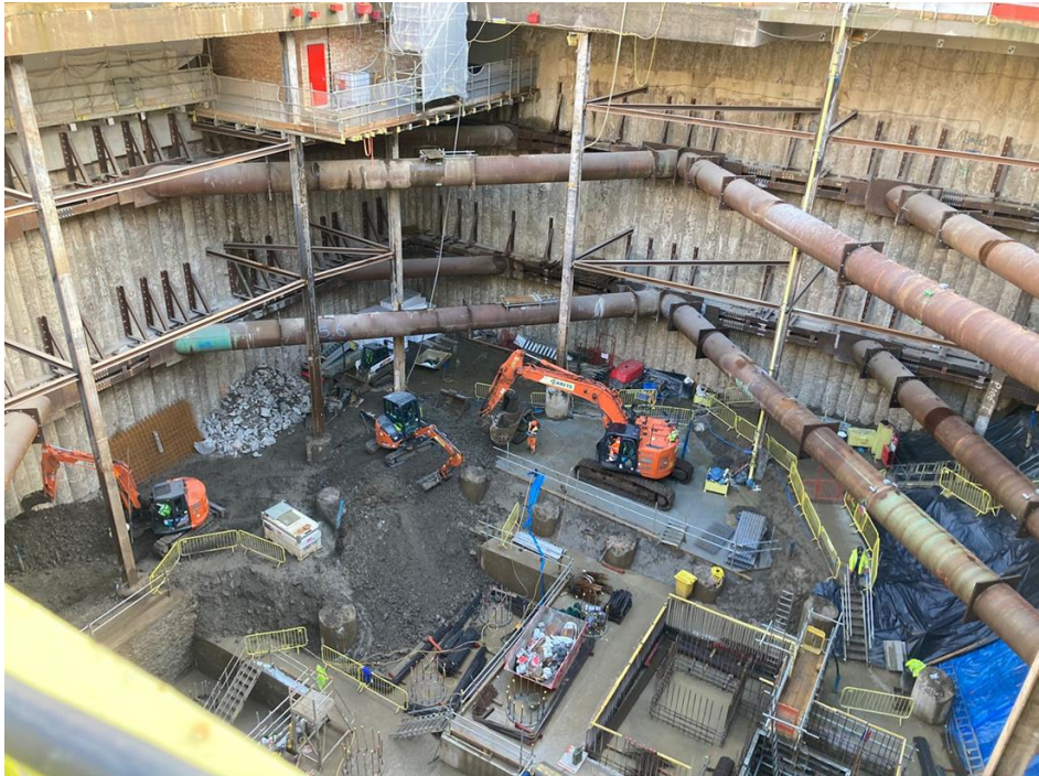
ZONE 2 LEVEL 2 BASEMENT SUBSTRUCTURE
