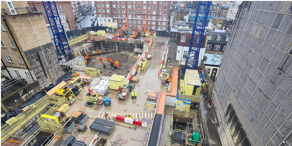
Zones 1 & 2 garden level slab works Looking east from Audley Square
