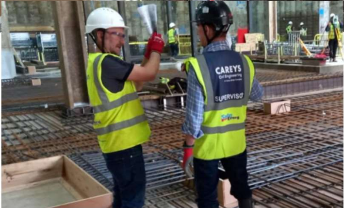
Zone 1 top down B2 substructure works
