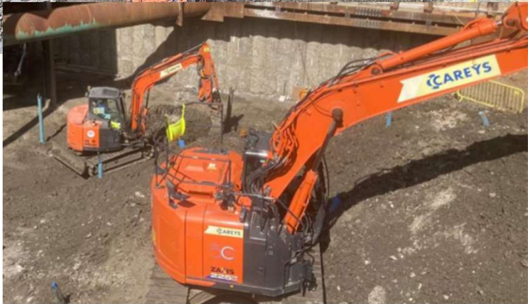
Zone 2 open cut excavation
