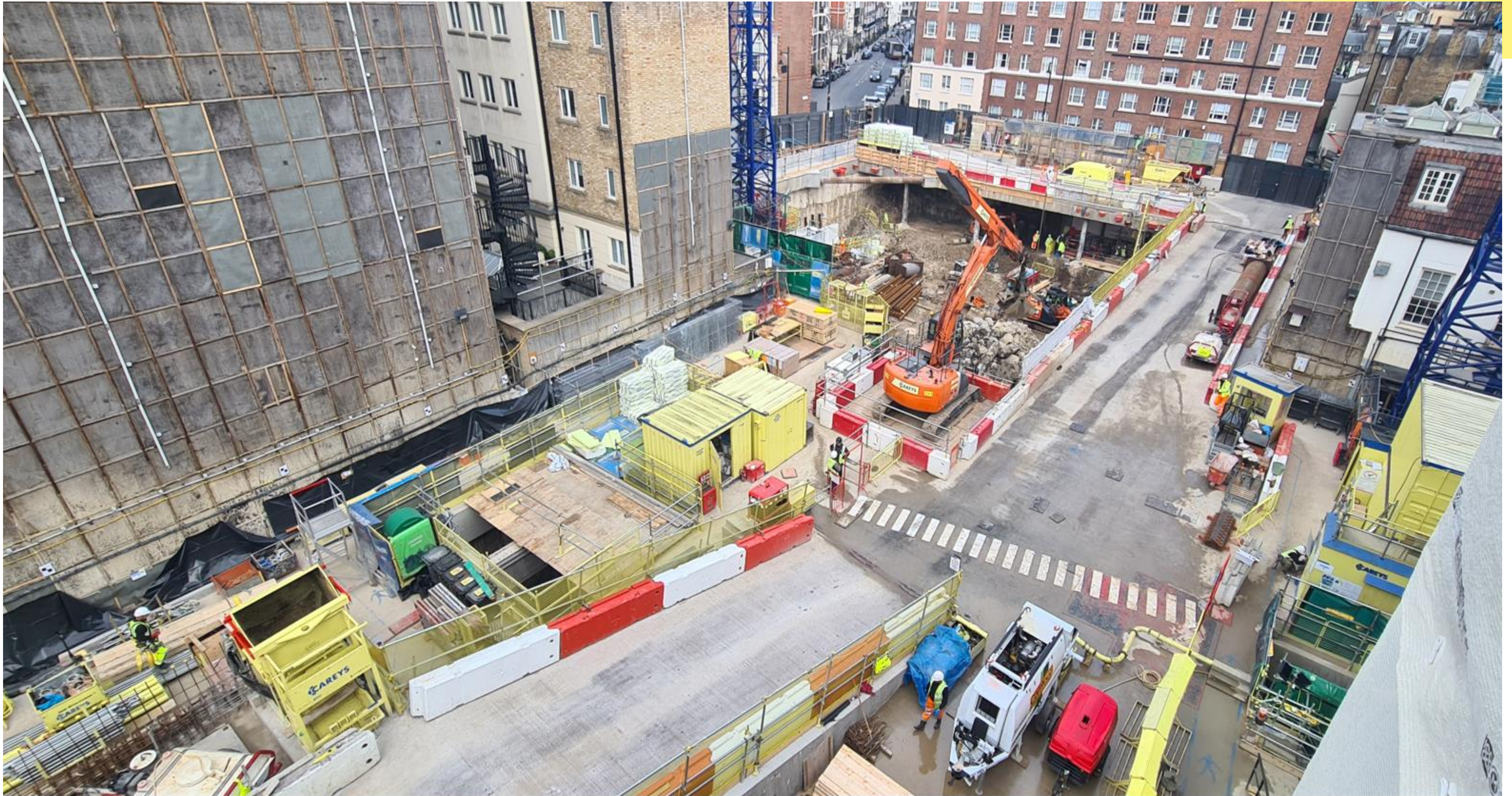
General Site Overview
