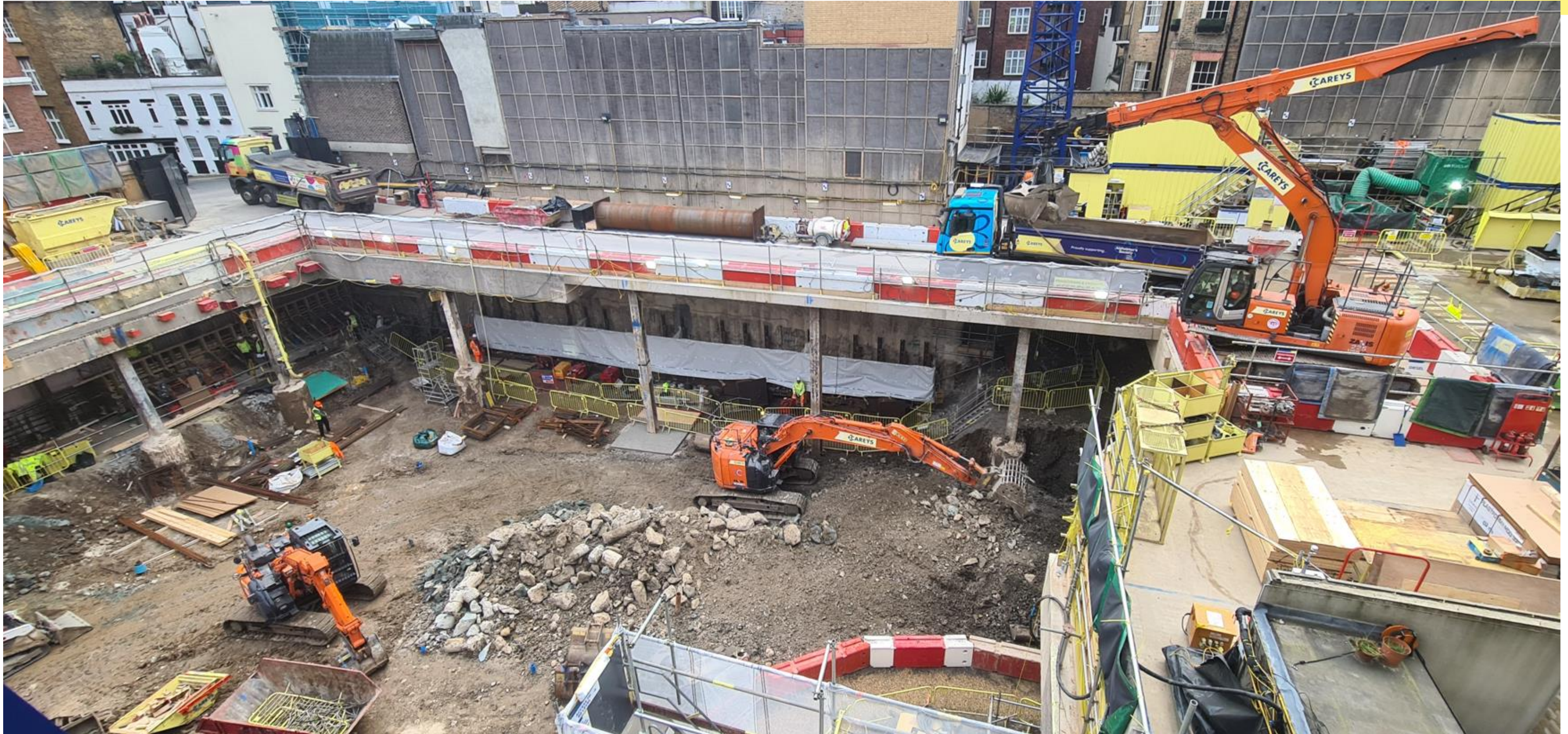
General Overview – Zone 2 Basement Works
