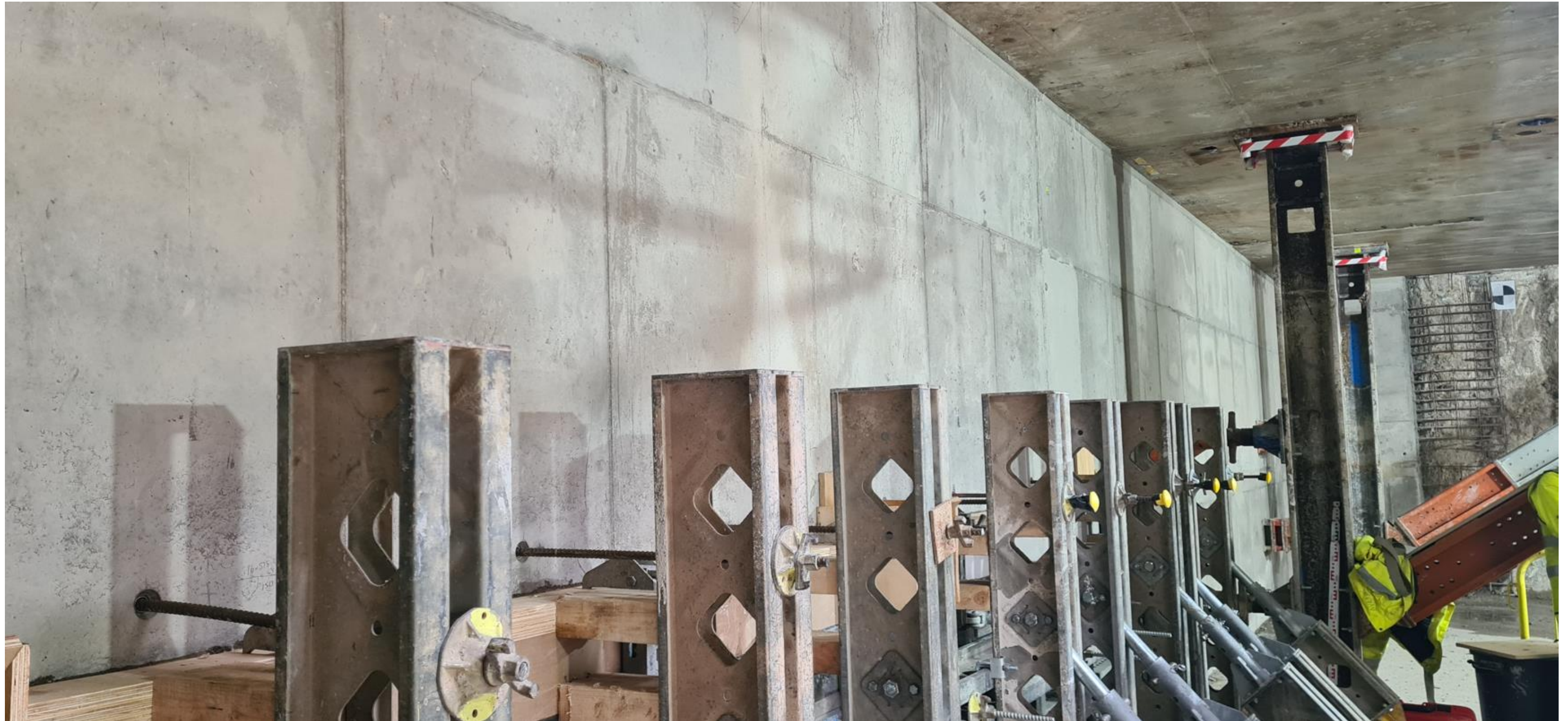
Basement Liner Wall Construction Progress – Along 3 Audley Square Elevation
