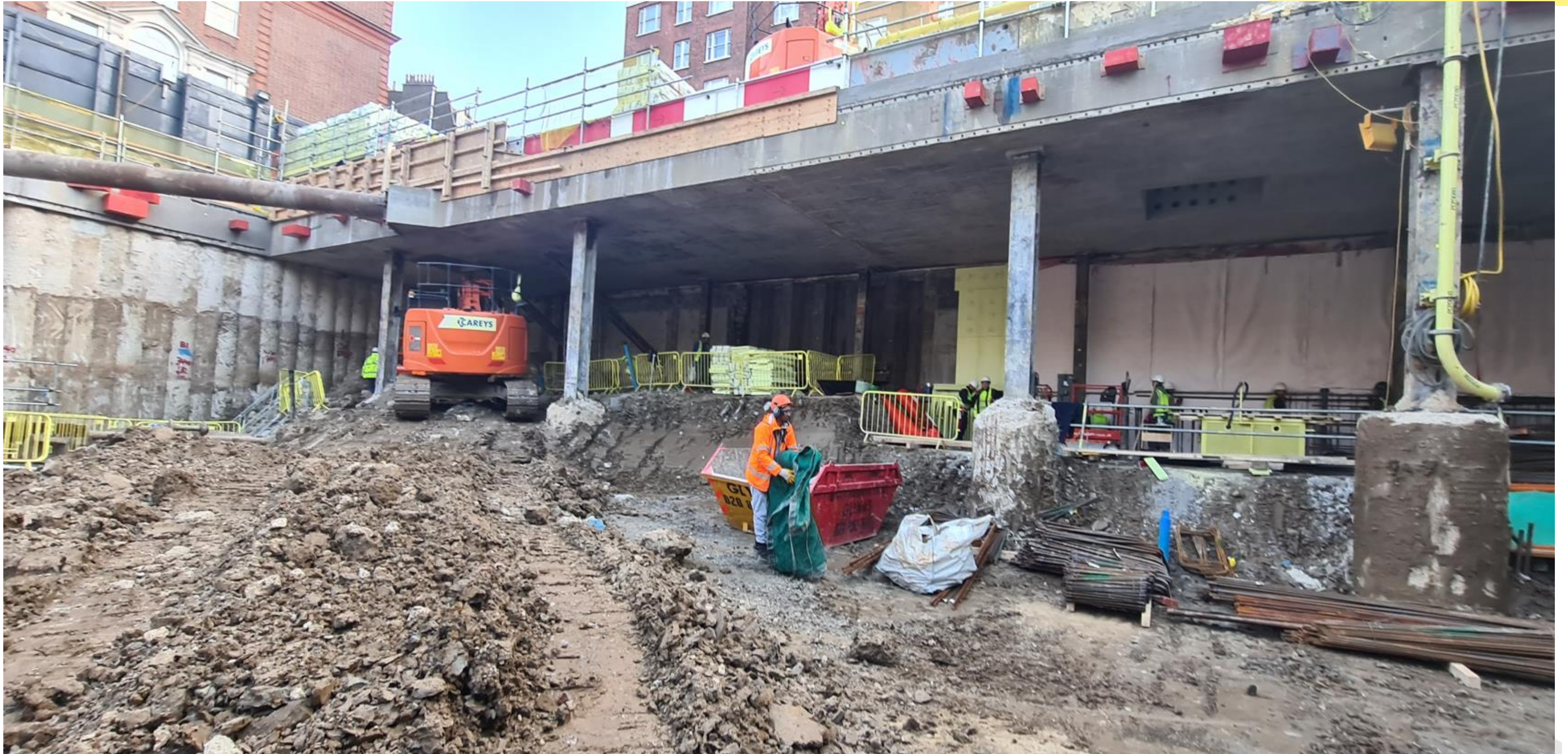
Typical View – Waverton Street – B2 Excavation Ongoing
