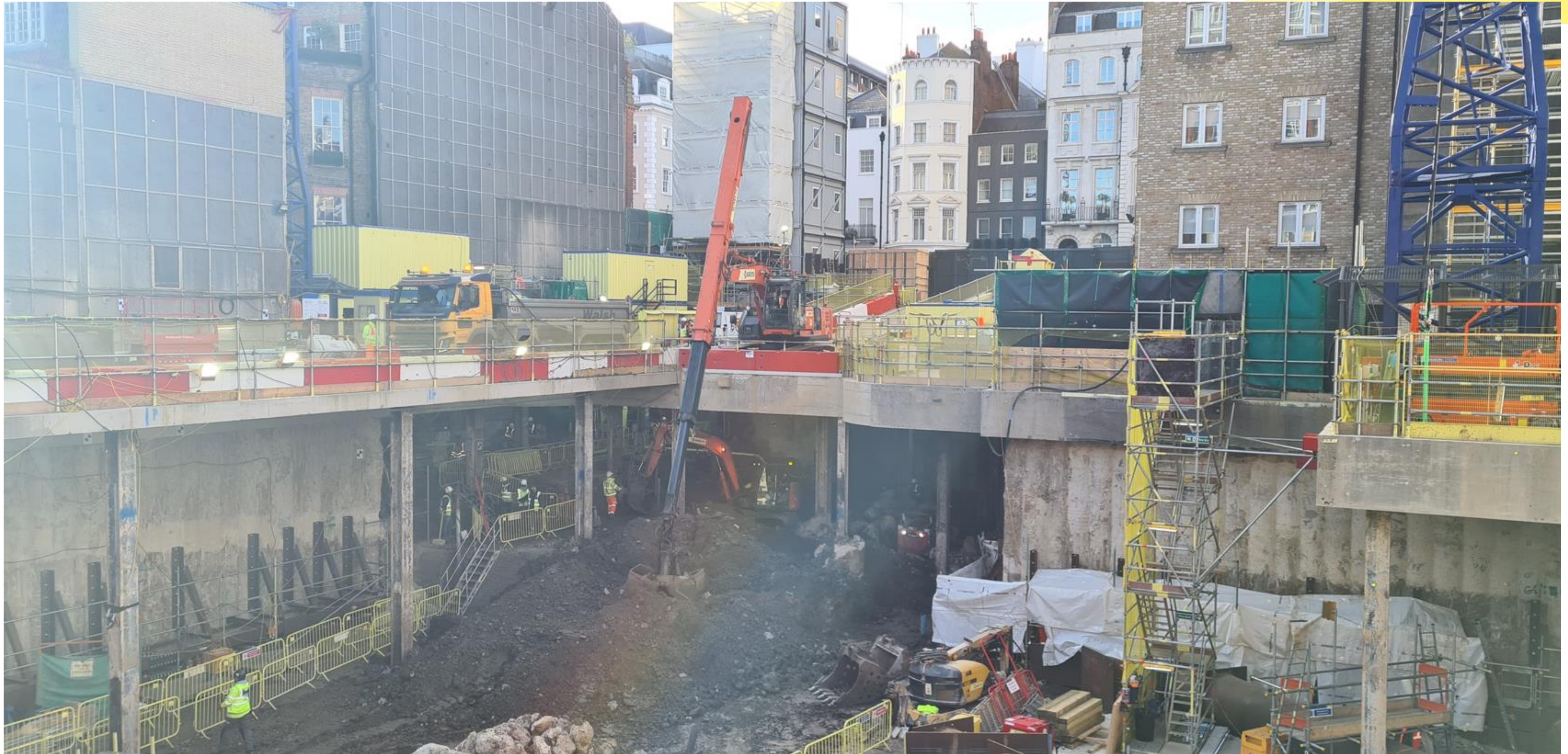
Overview – Long Reach Excavator Removing spoil from basement
