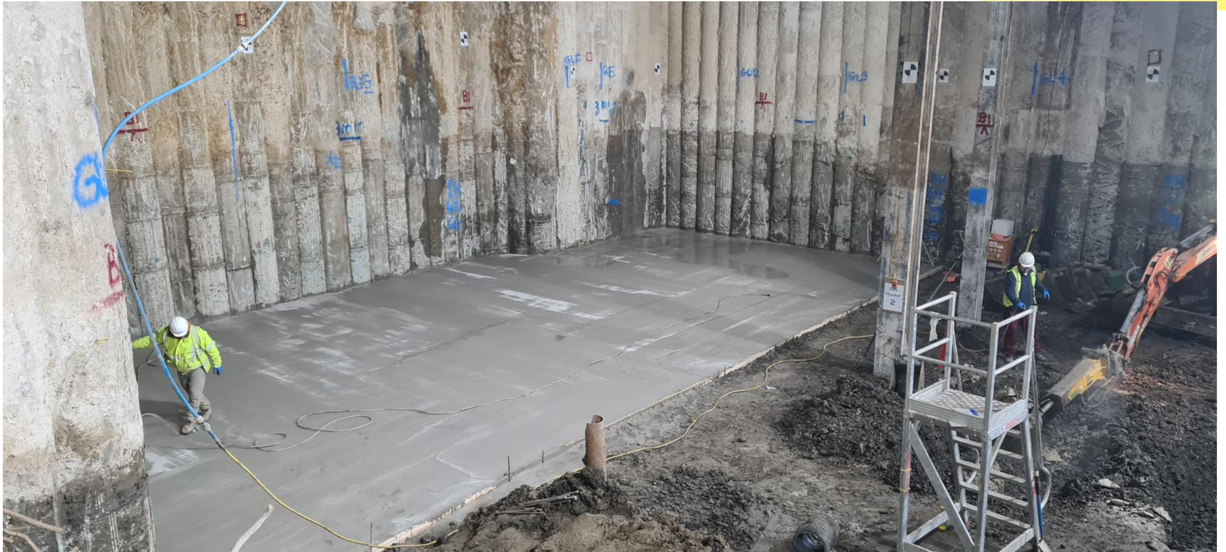
B2 Slab Preparation in the Top Down Zone 1 Work Area
