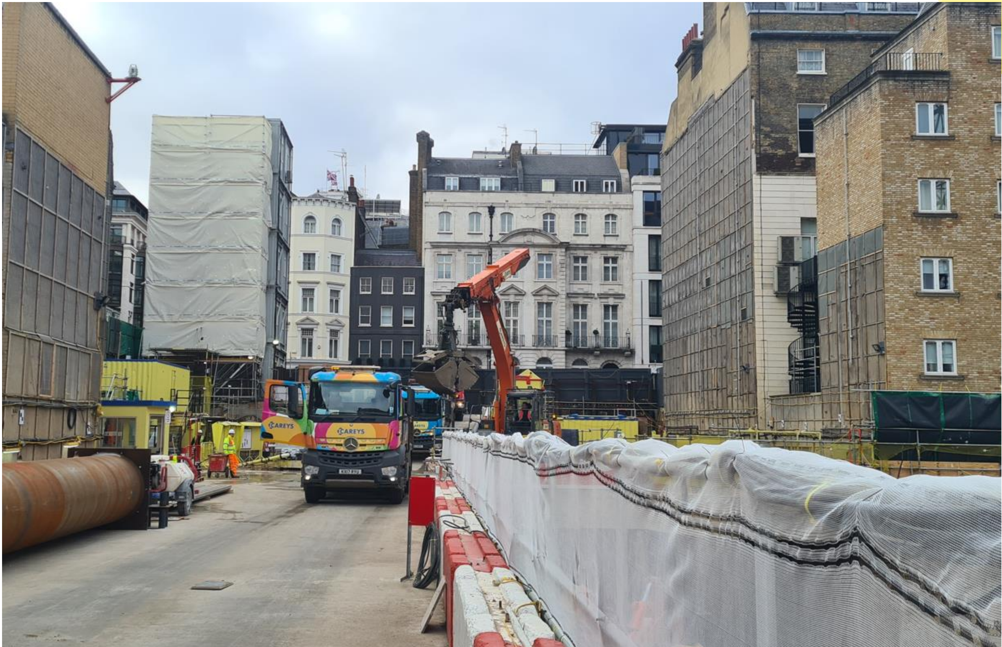
Tipper Trucks – Getting Loaded By Excavator
