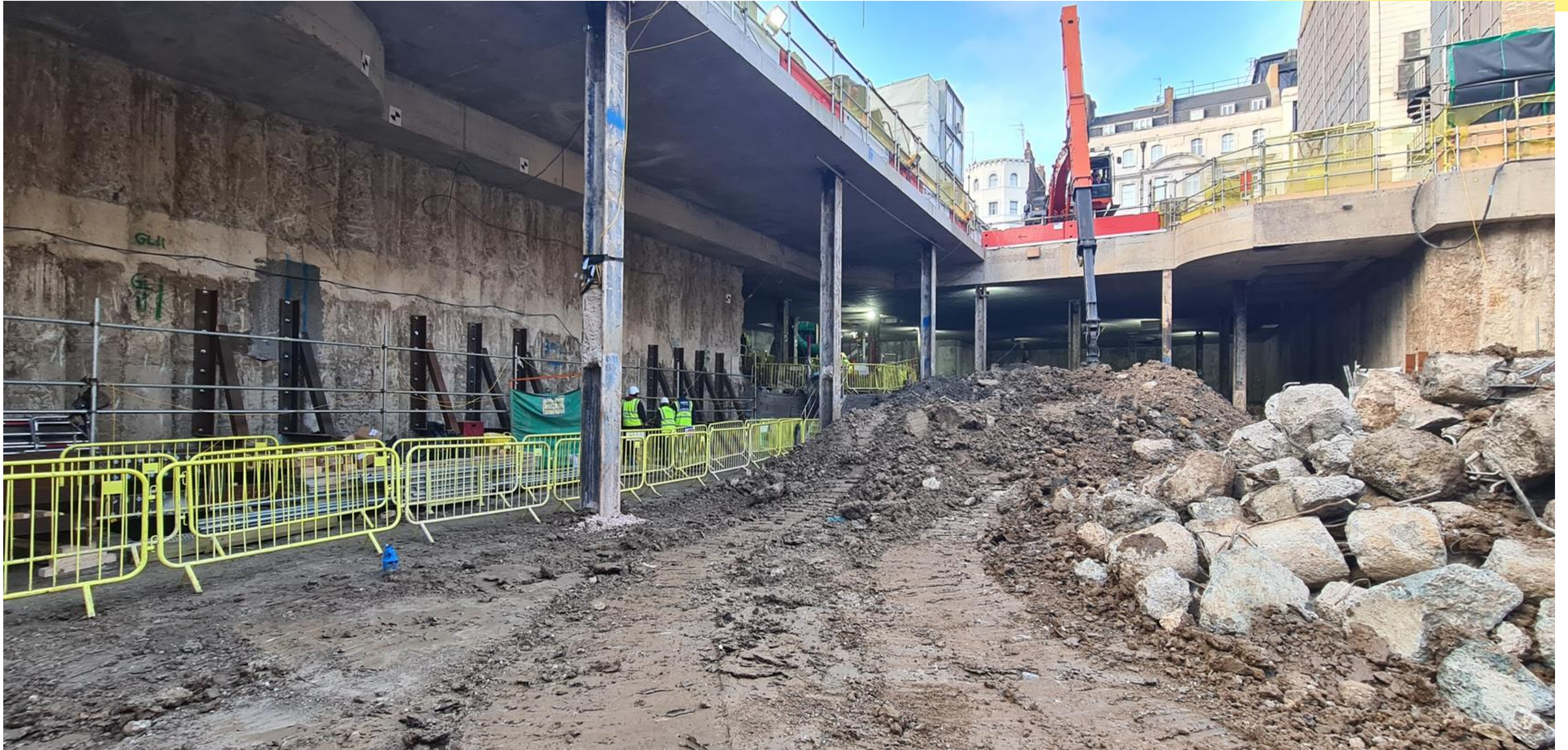
Typical View – Red Lion Yard – B2 Excavation Ongoing
