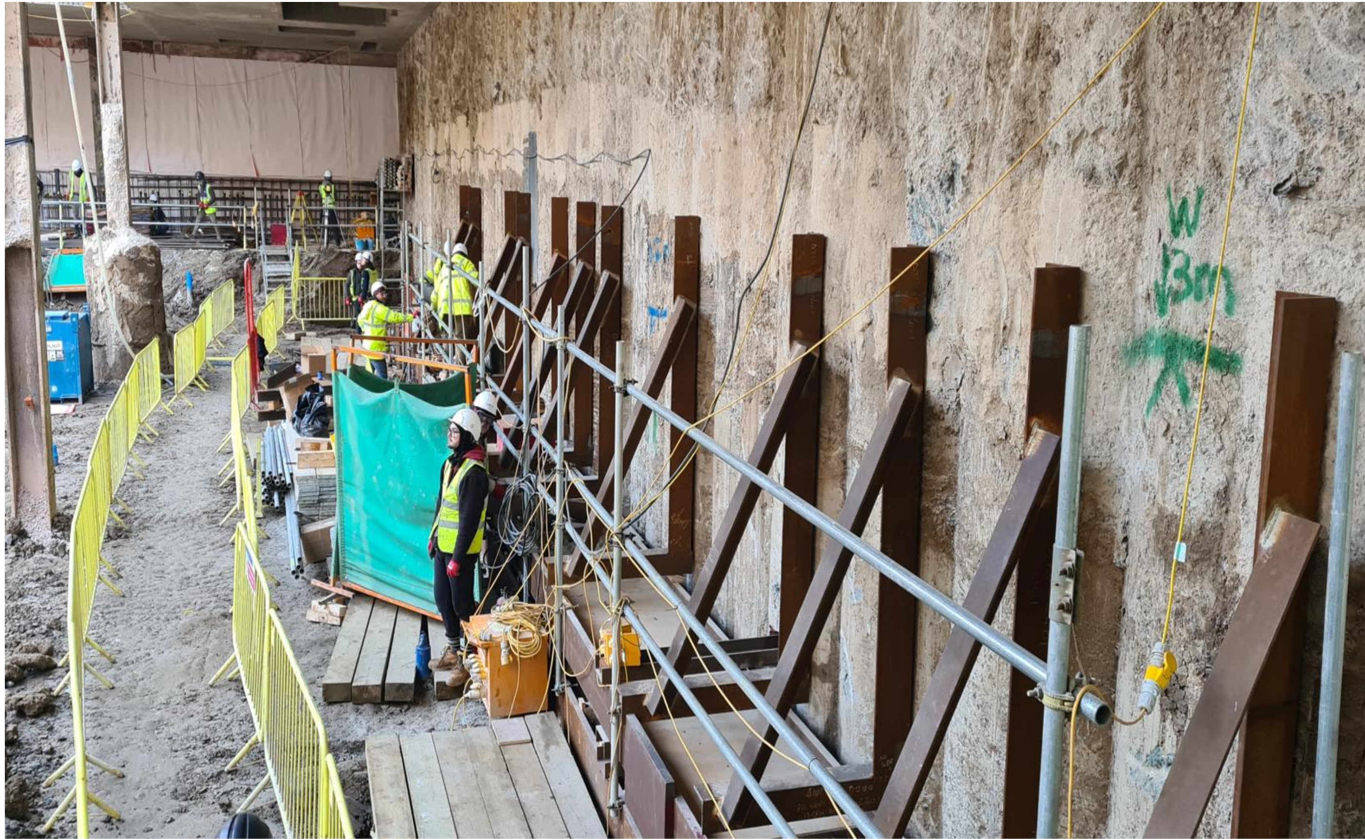
Steel Propping Installation – At B2 Level in Zone 2
