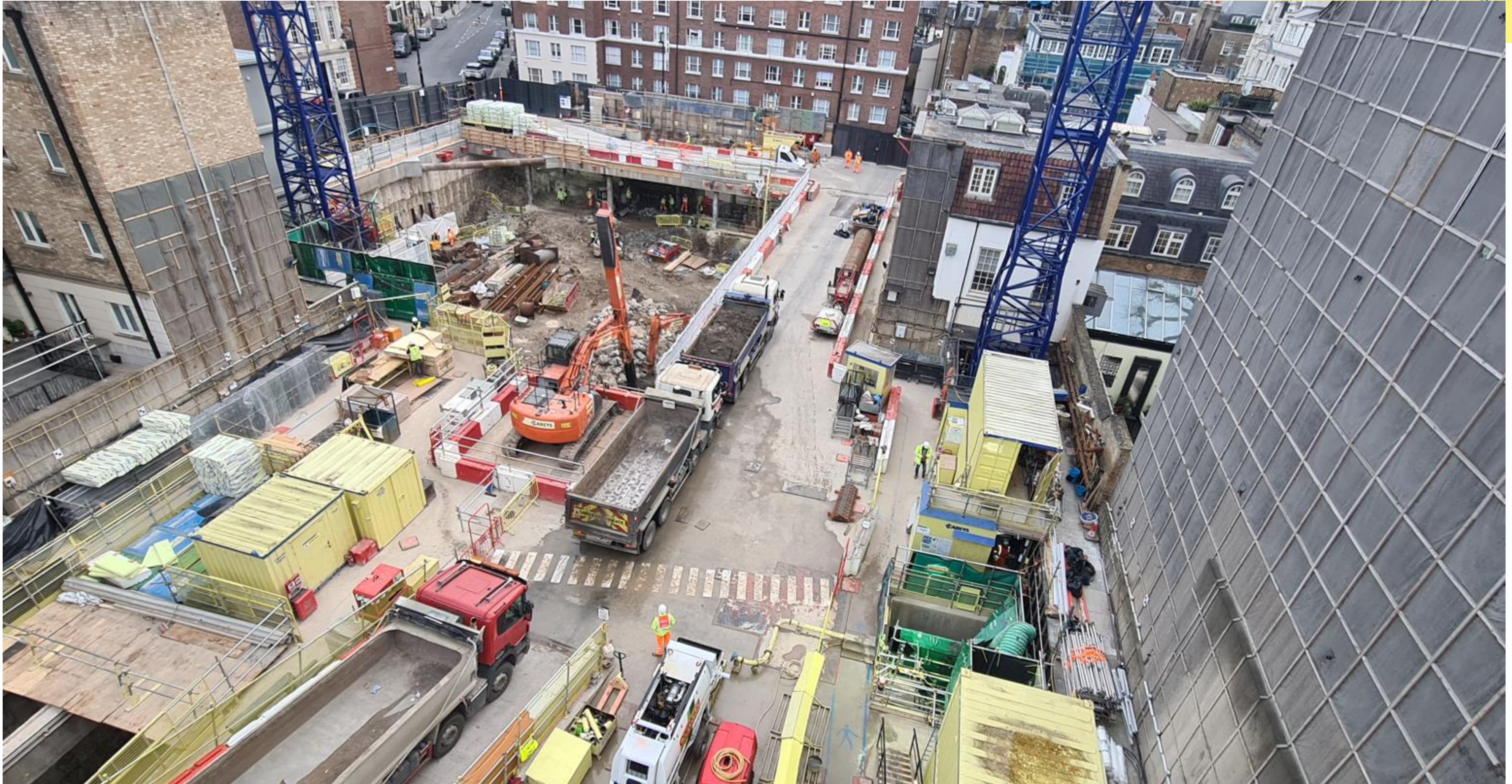
Tipper Trucks – Getting Loaded By Excavator
