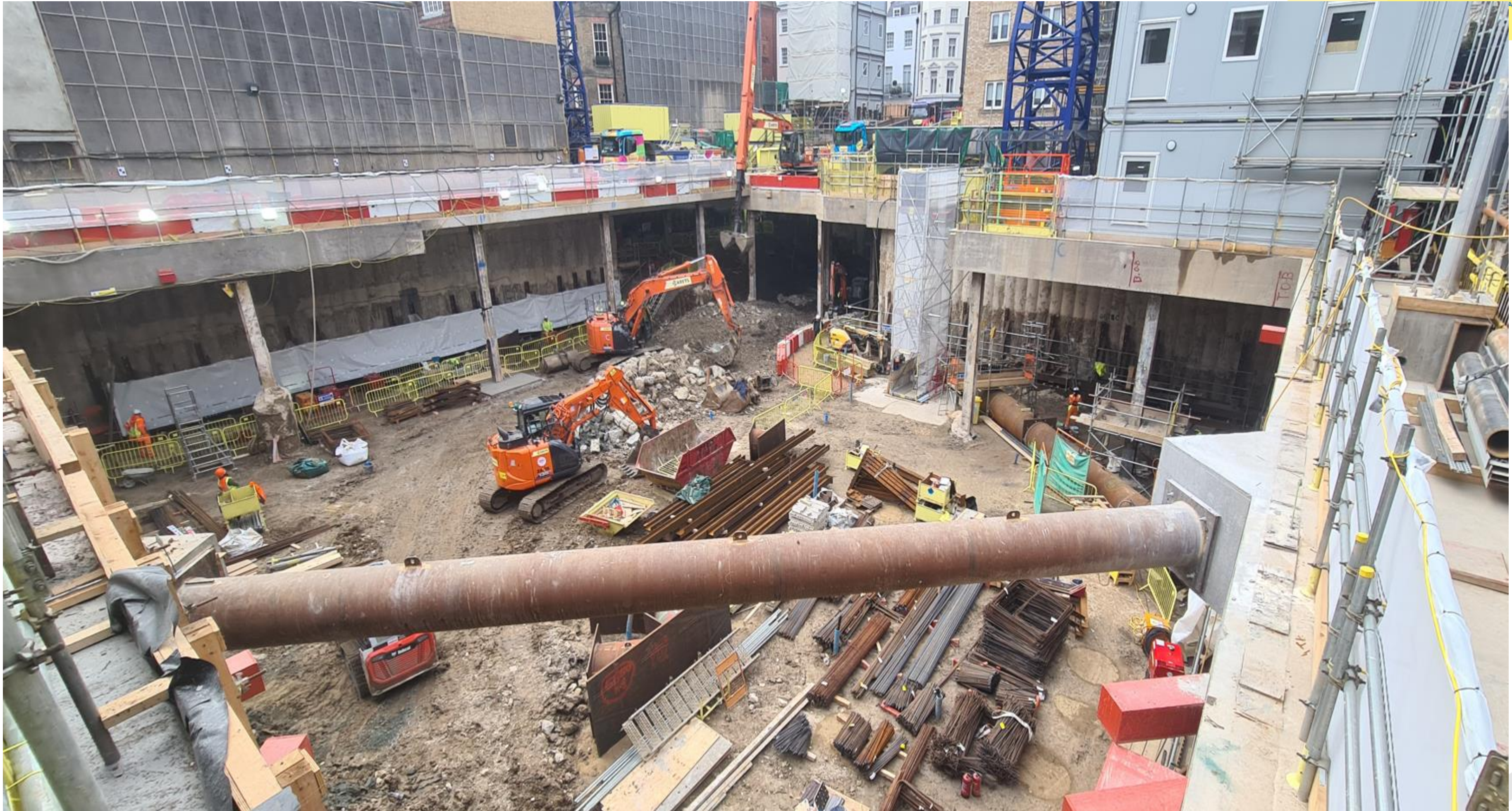
General Overview – Zone 2 Basement Works
