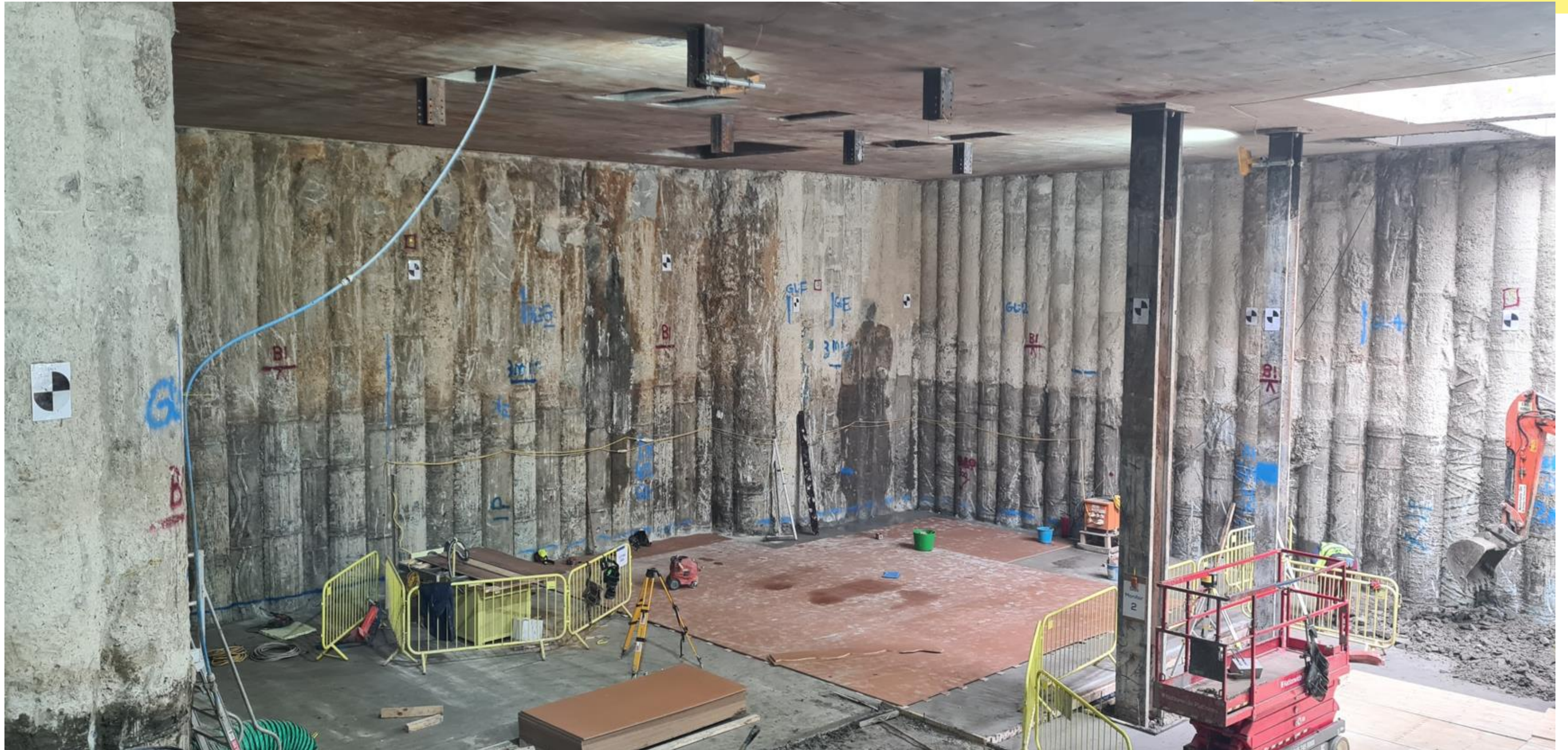
B2 Slab Preparation in the Top Down Zone 1 Work Area
