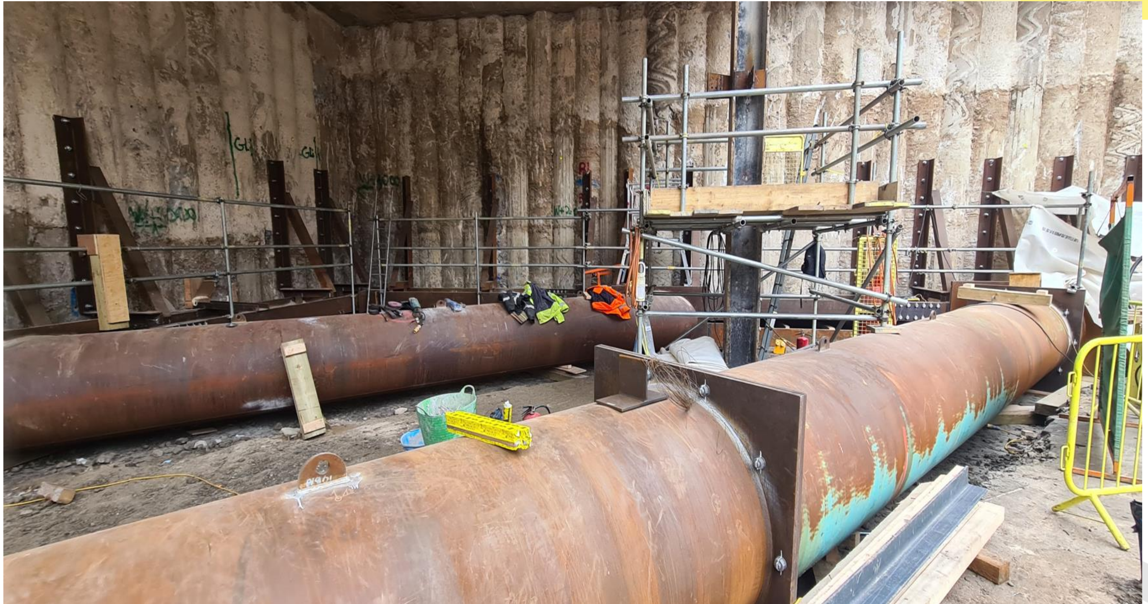
Steel Propping Installation – At B2 Level in Zone 2
