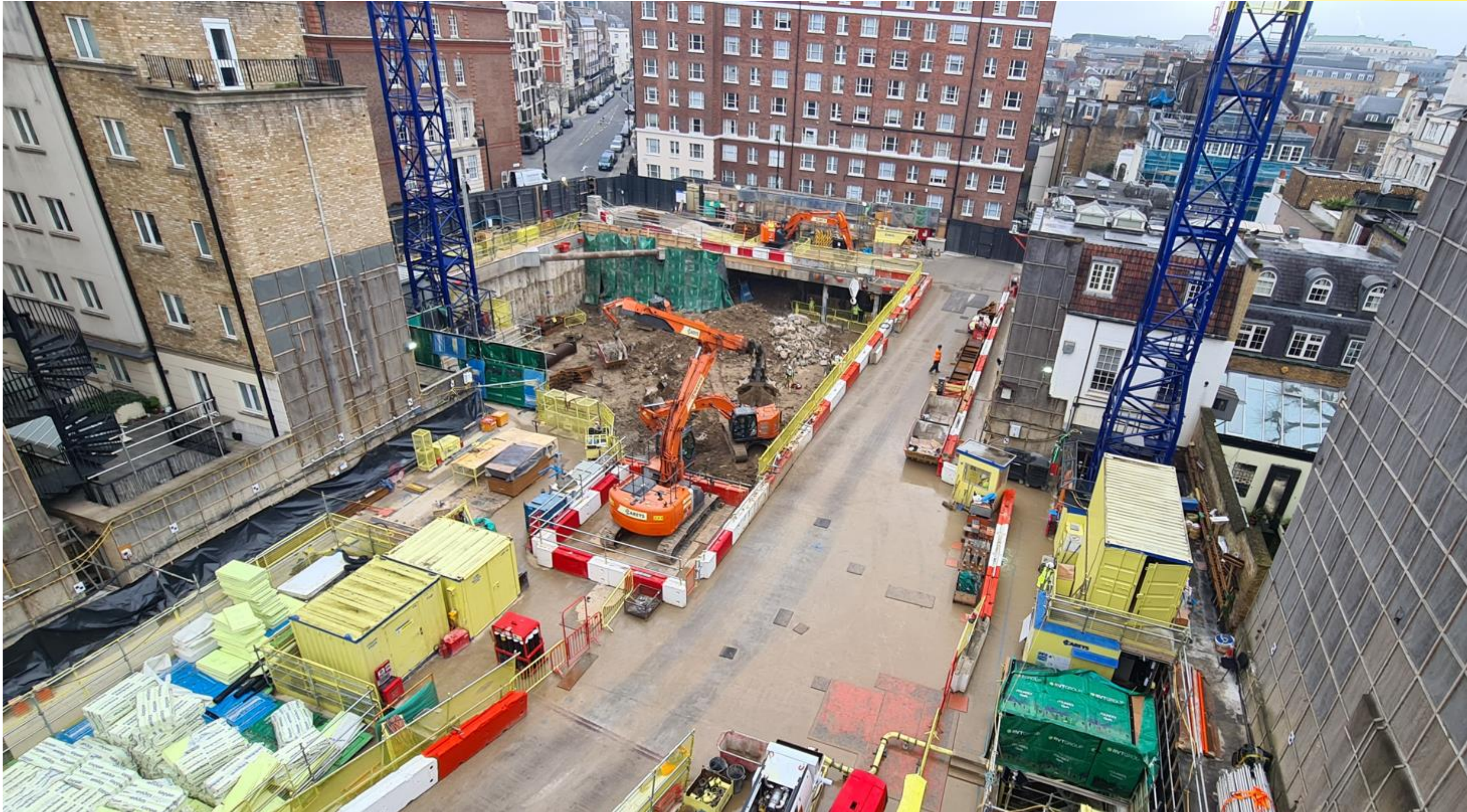
Current Site Overview
