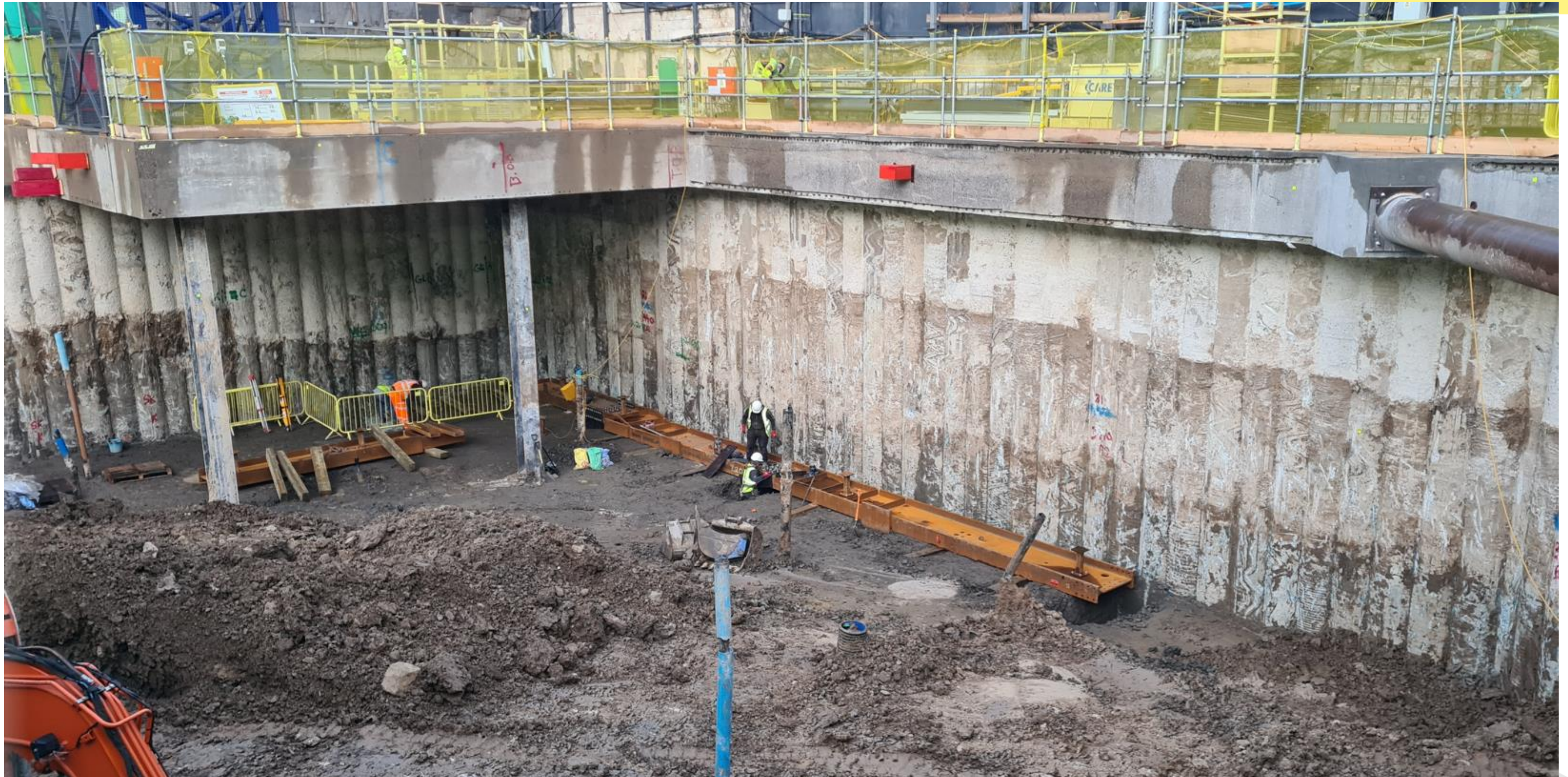
B2 Basement Propping Supports being installed – Hill Street Elevation
