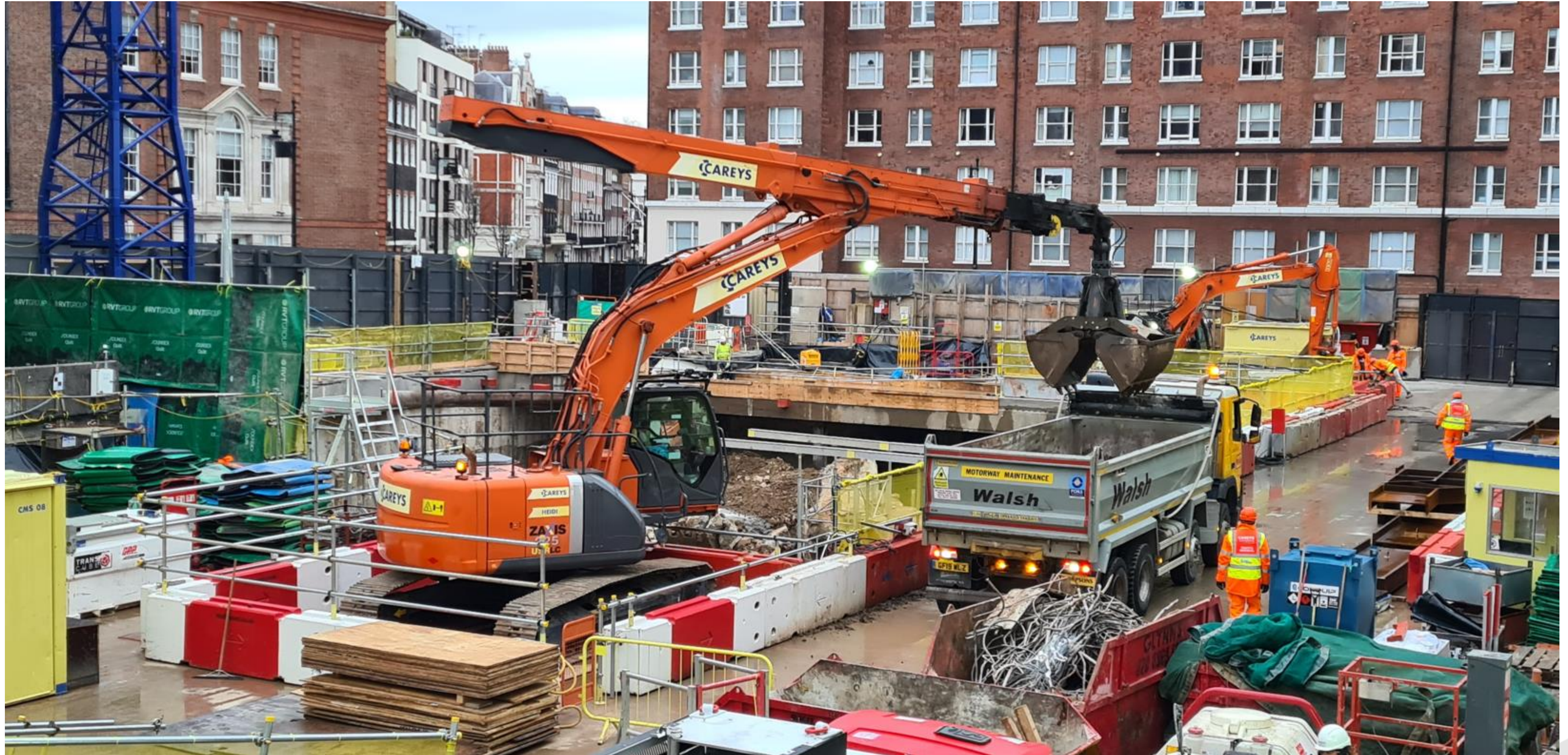
Long Reach Excavator In Action
