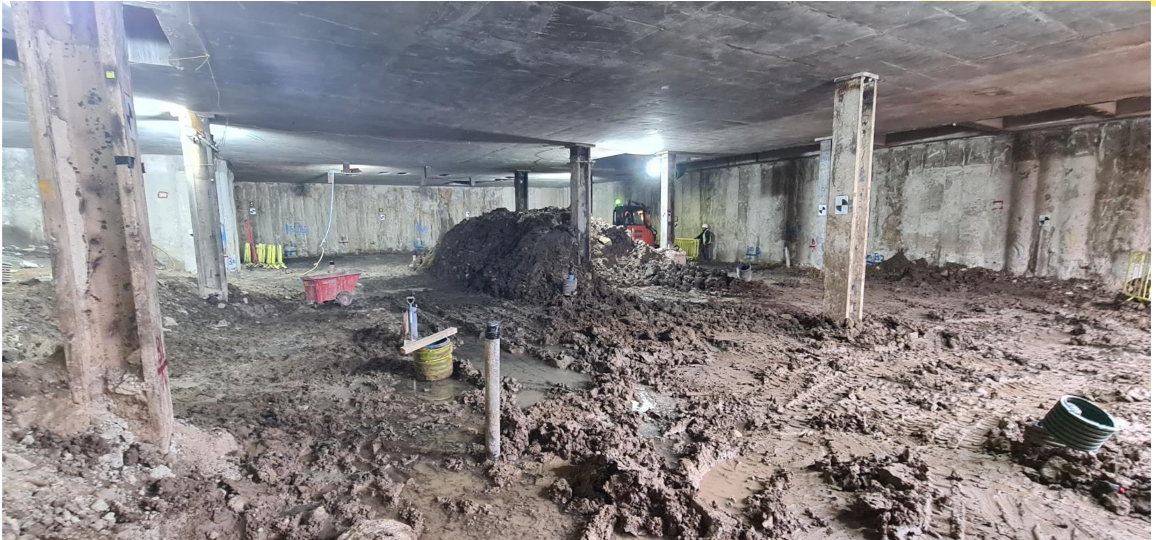
Bulk excavation ongoing in basement area – Zone 1 Top Down
