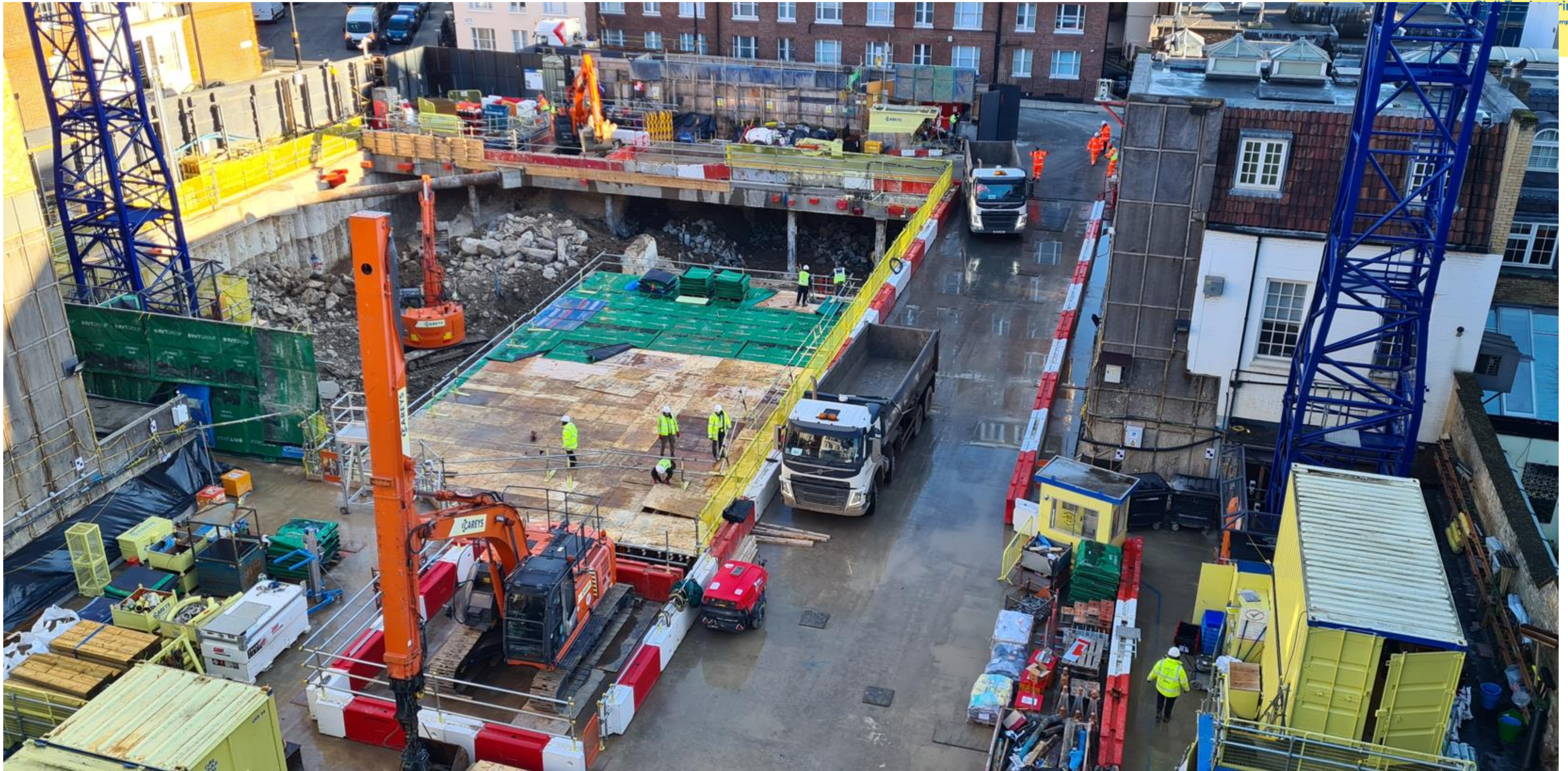
Slab Removal Complete – Removing Acoustic Frame in Zone 2
