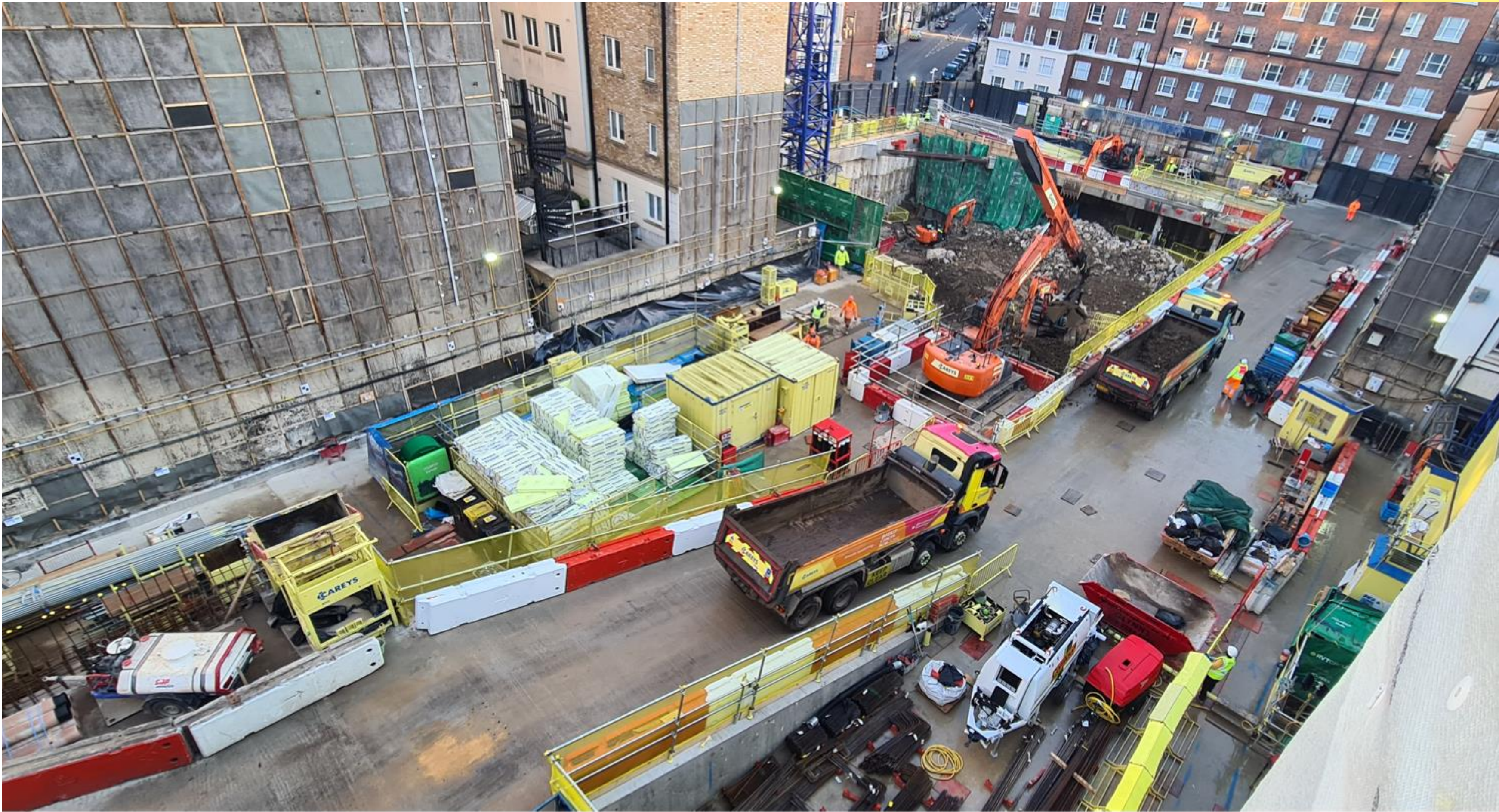
Vehicle Access Ramp In Use – Loading Tipper Trucks
