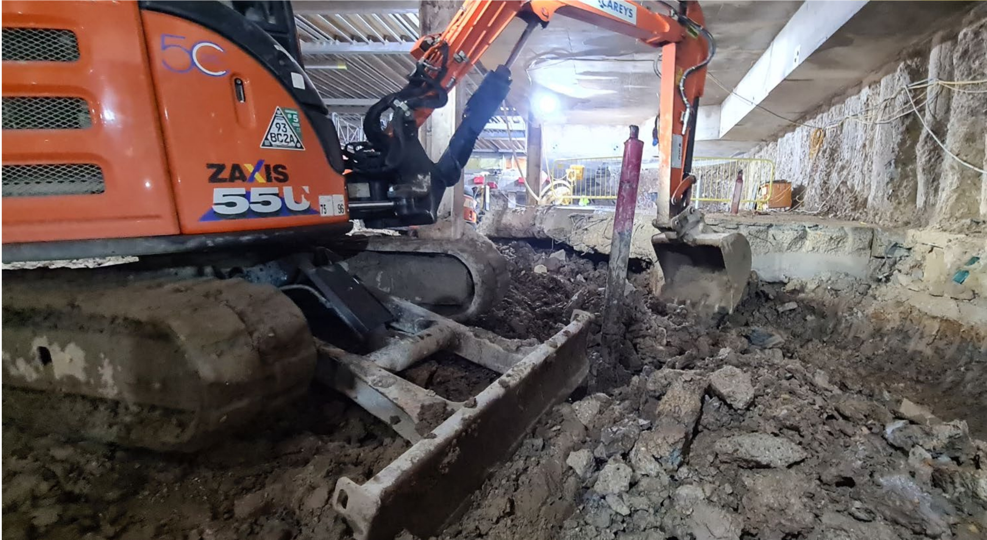
Excavator digging under slab to aid removal
