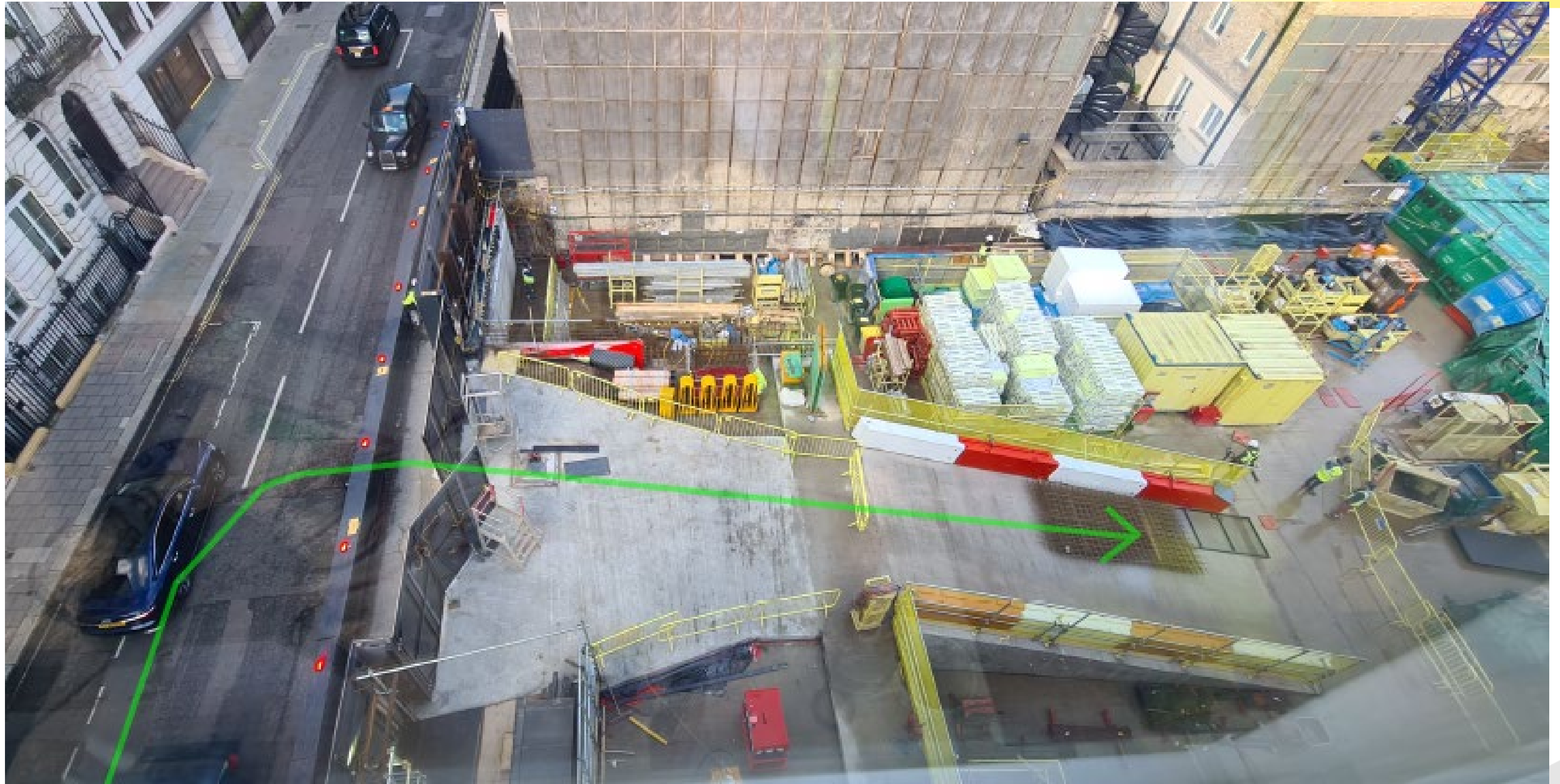
Completed Gate 1 installed on South Audley Street.
