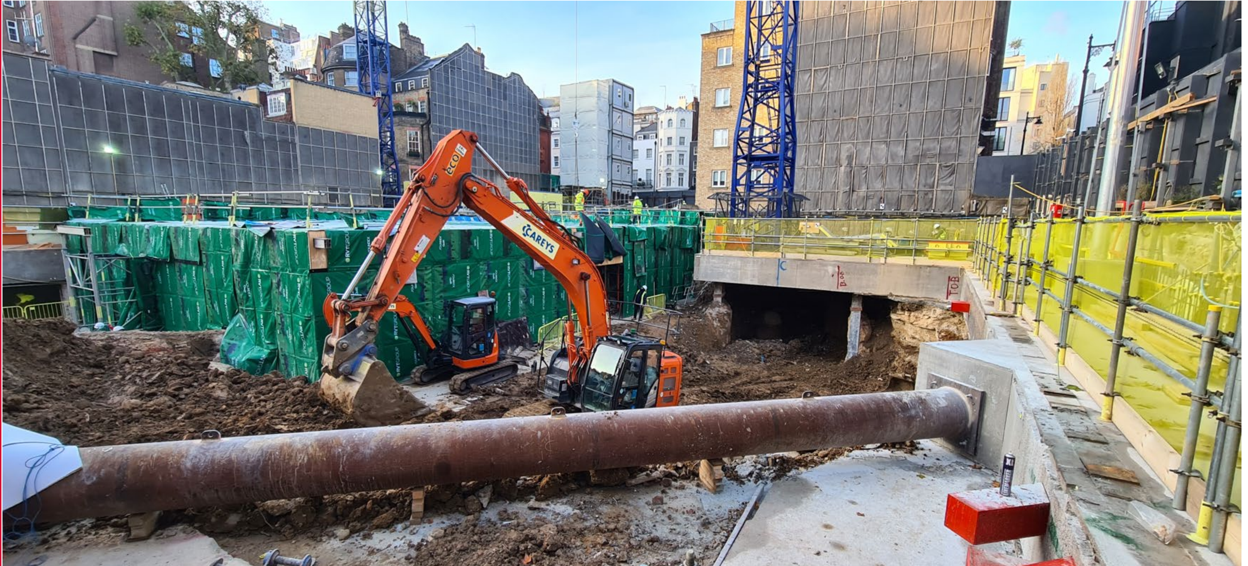
Excavating under Garden Slab along 51 Hill Street elevation.
