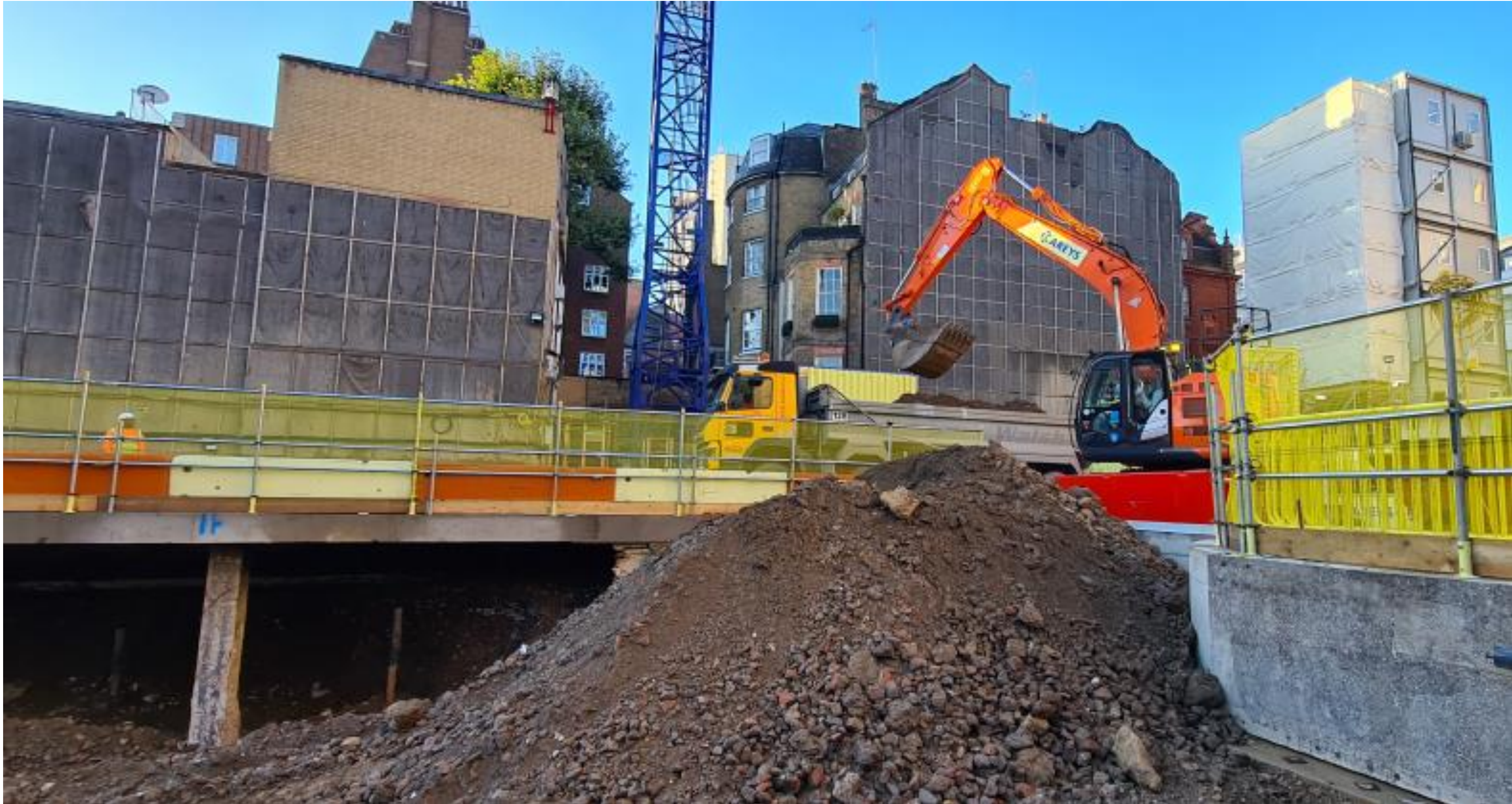
Excavator Loading Tipper Truck On The Traffic Slab
