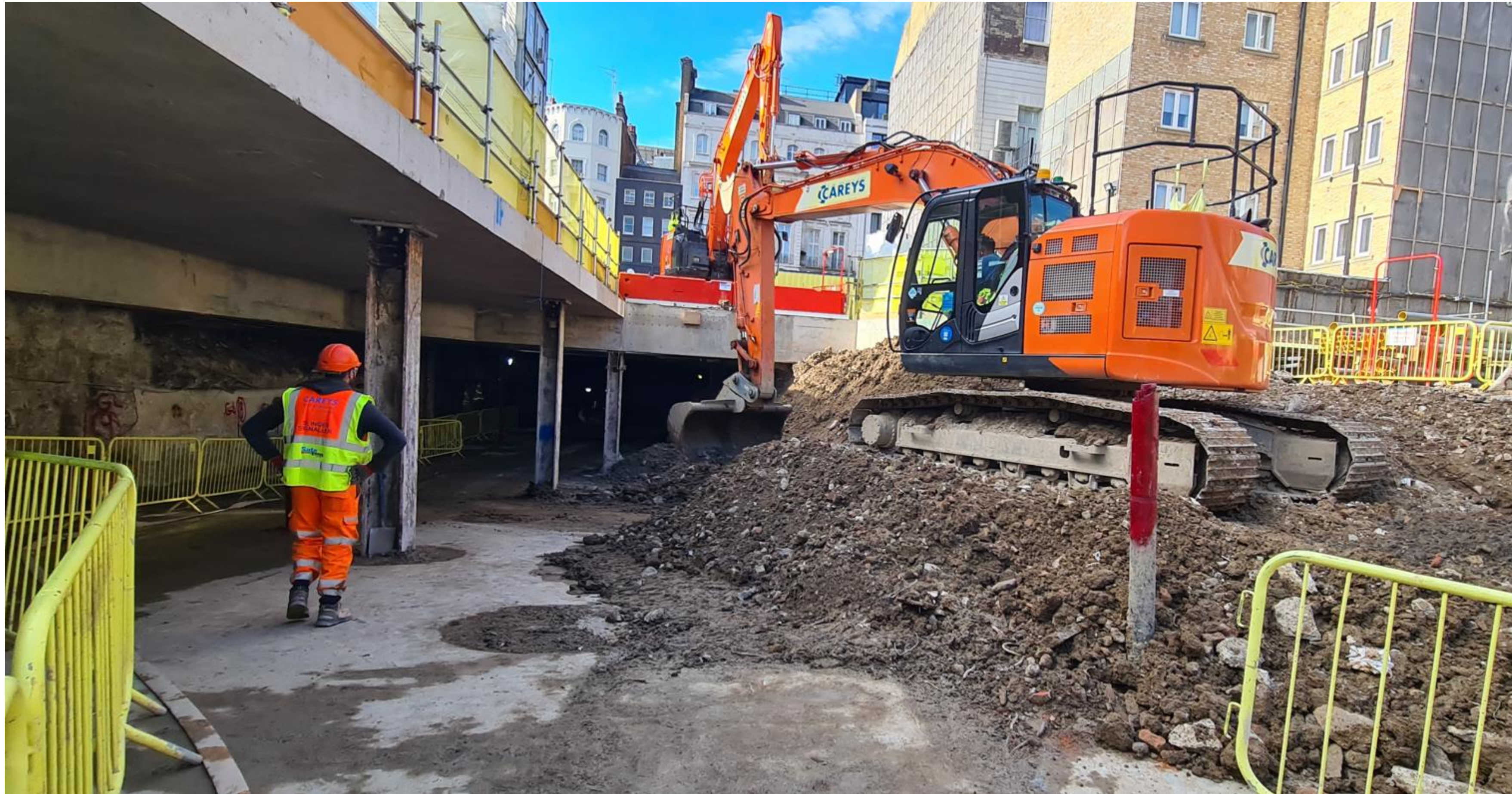
Excavation Progress Under New Garden Level Slab
