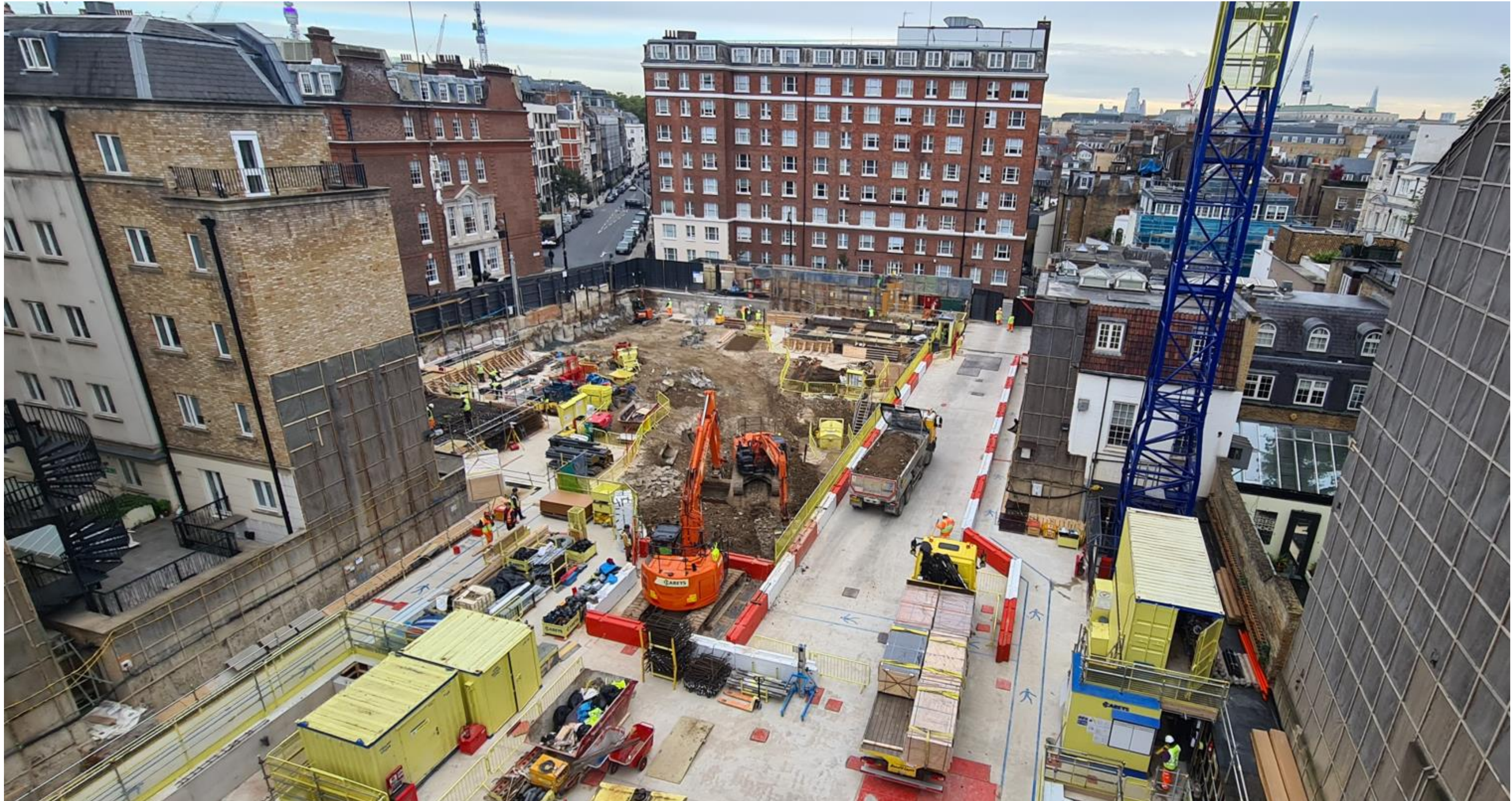
Current Overview of Site
