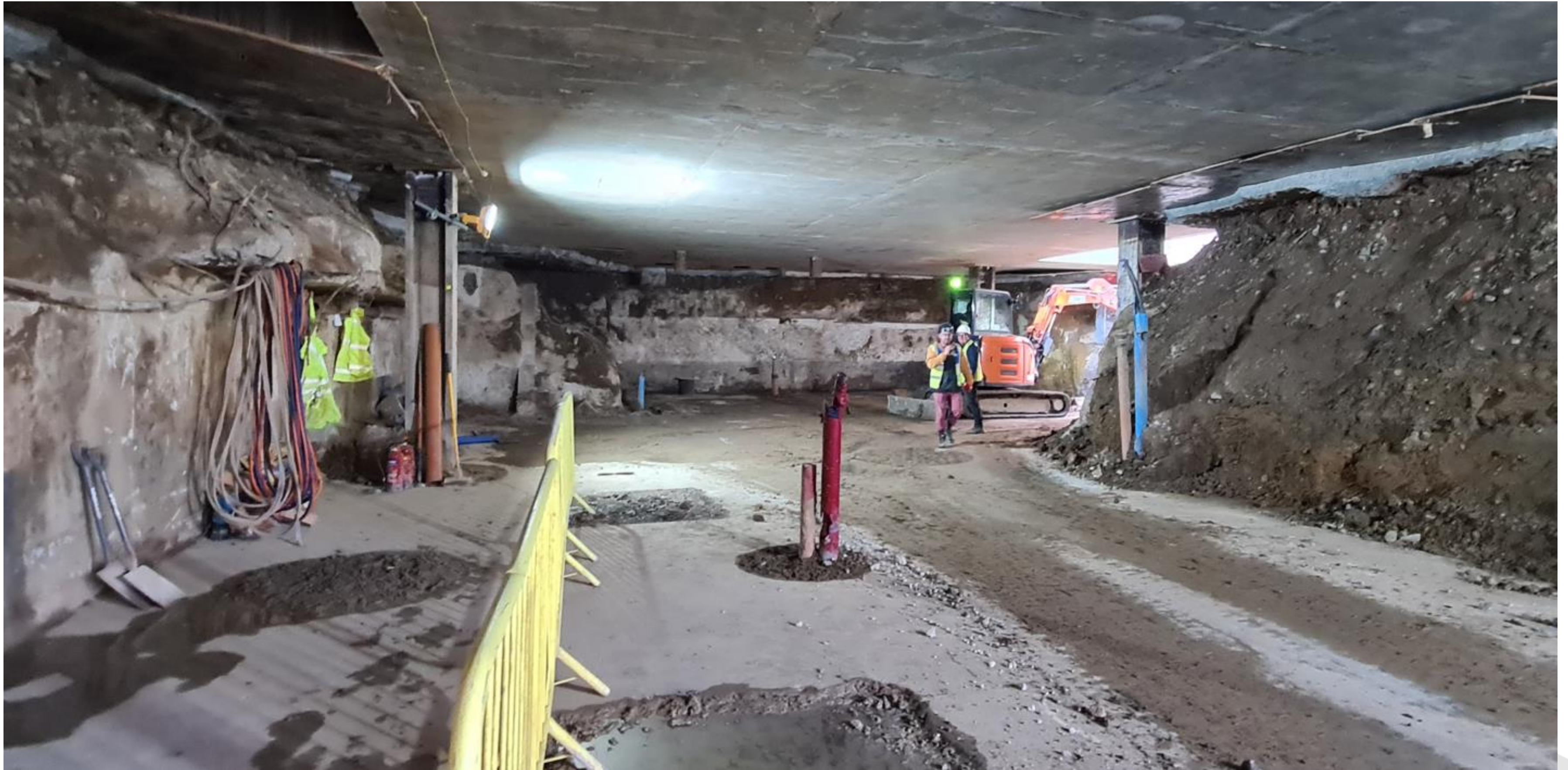
Excavation Progress Under New Garden Level Slab
