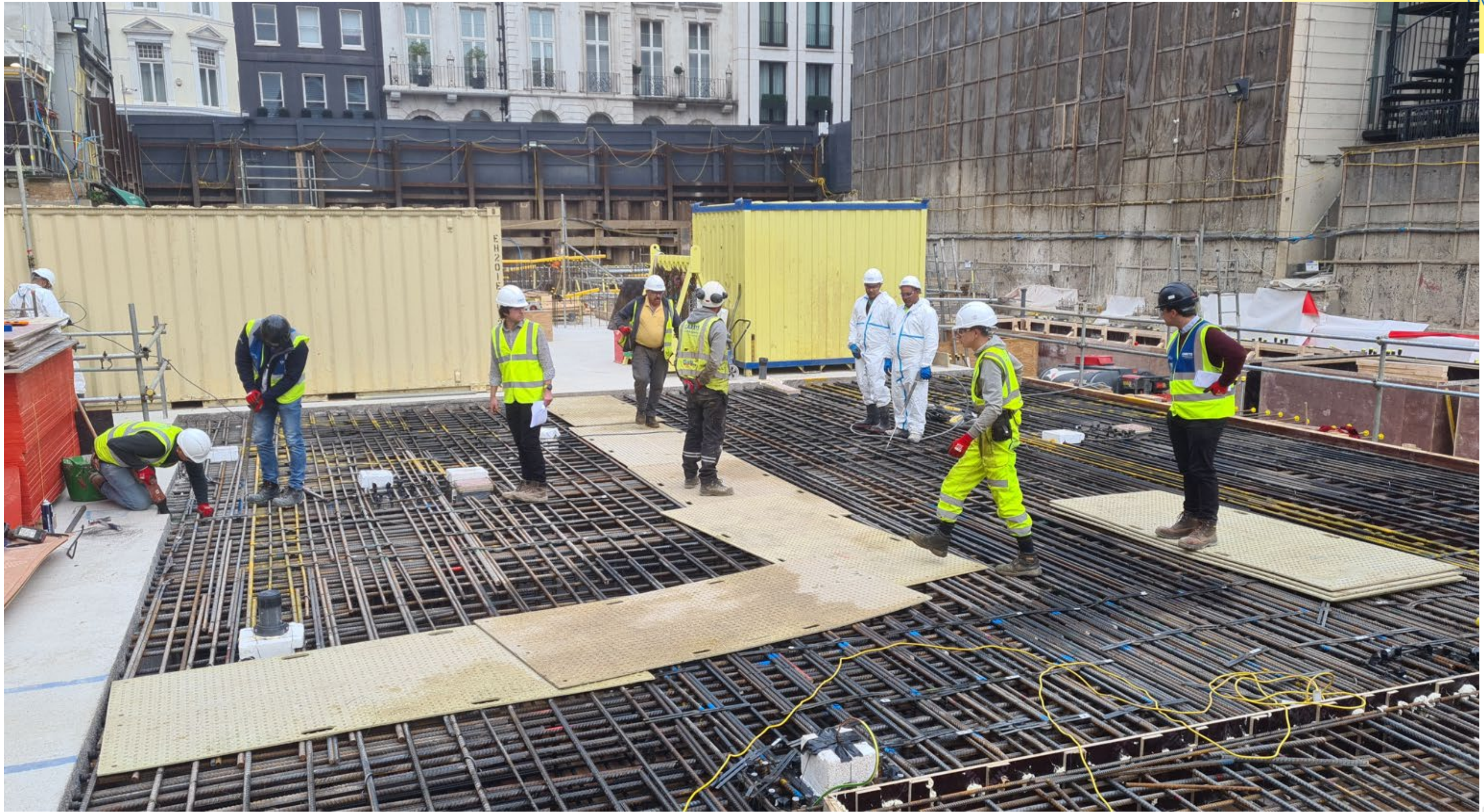
Site team working on typical Ground Floor Slab Construction
