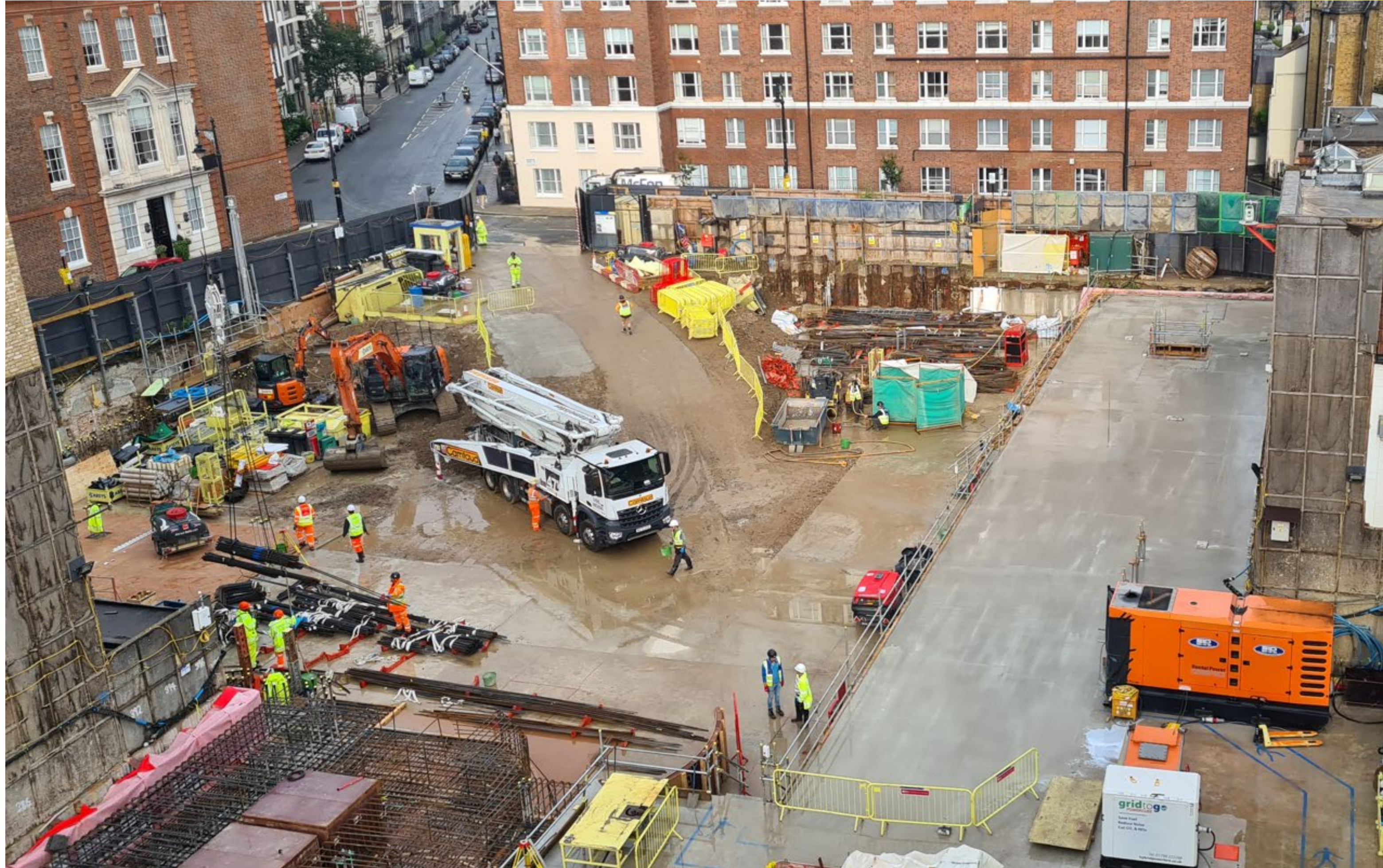
Pour 7 G0 Slab along RLY – Completed 14/09/21 (Today)
