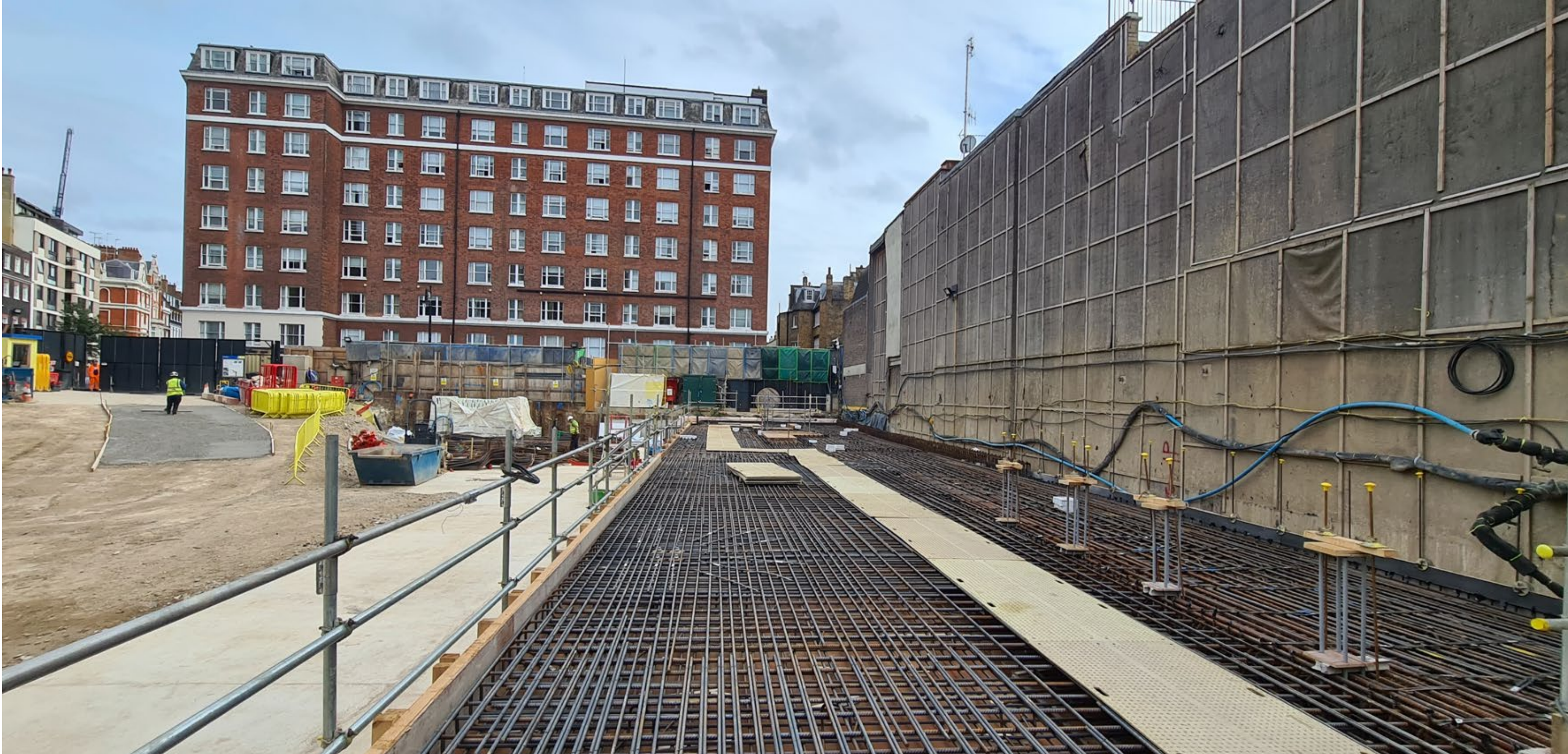
Pour 7 G0 Slab ready to cast along Rey Lion Yard Elevation
