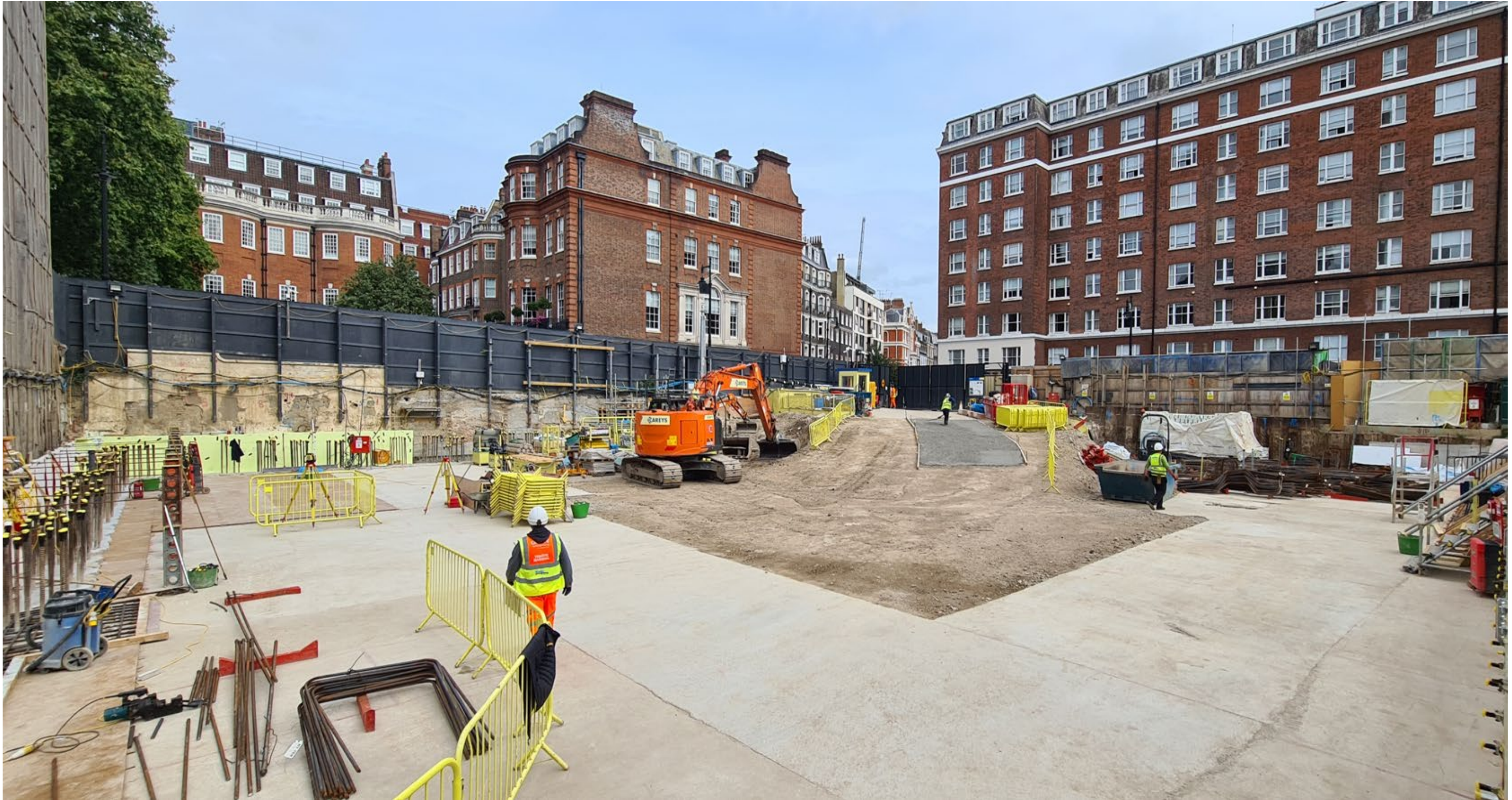
Commencement of Pour 1 G0 Slab along 51 Hill Street Elevation
