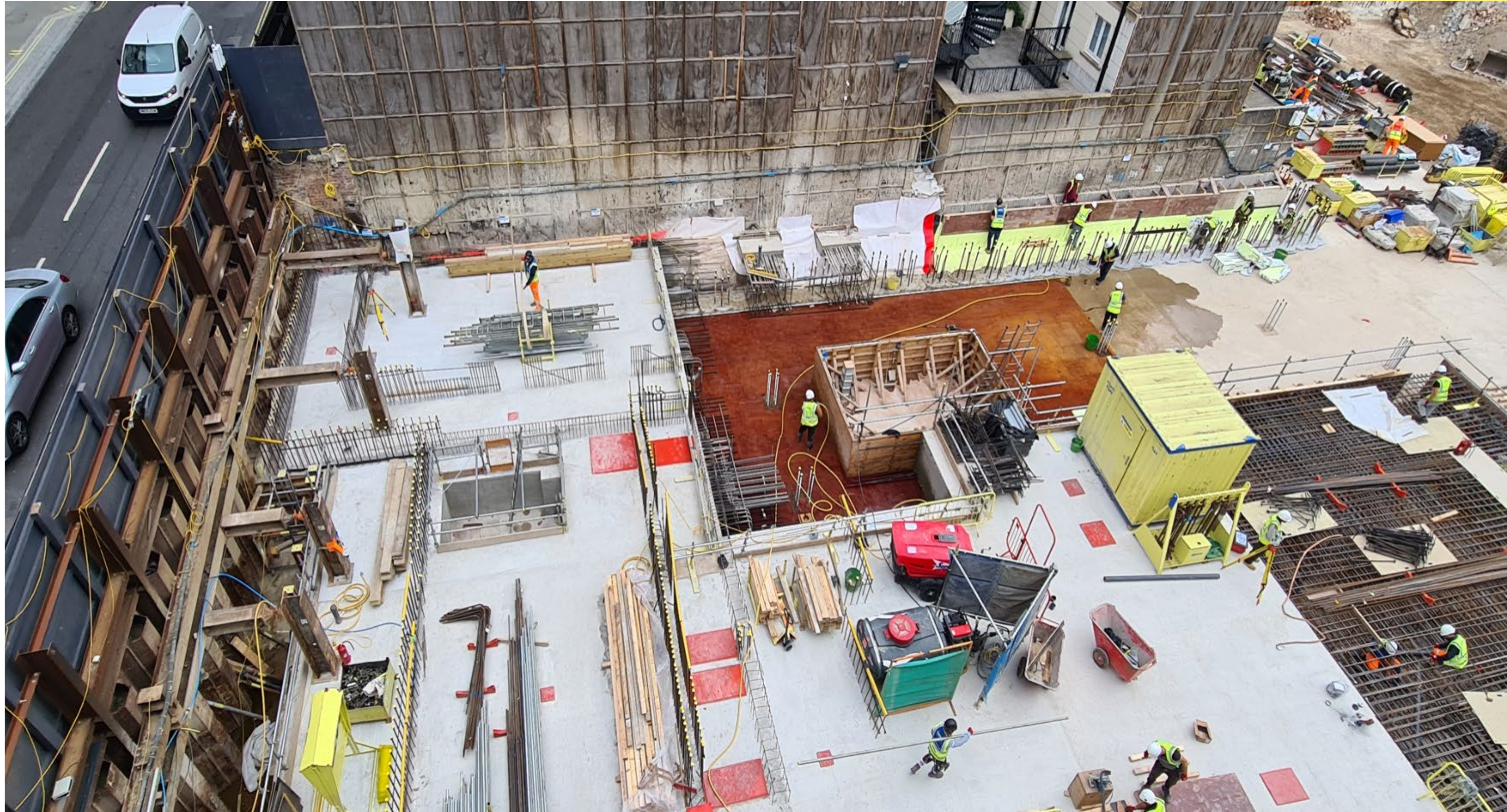
Example of Completed Slabs cast along South Audley Street Elevation
