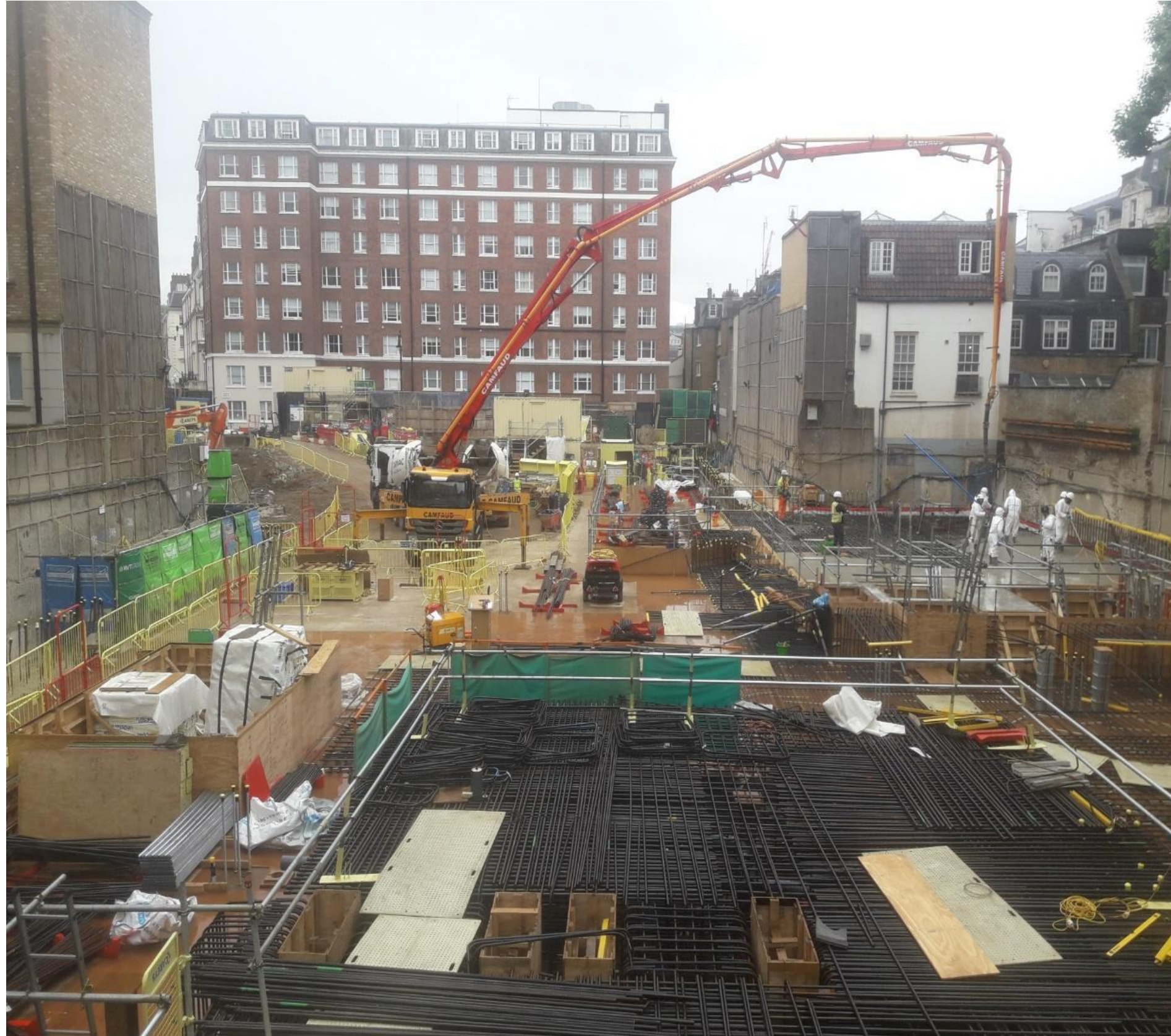
Team placing concrete using mobile concrete pump
