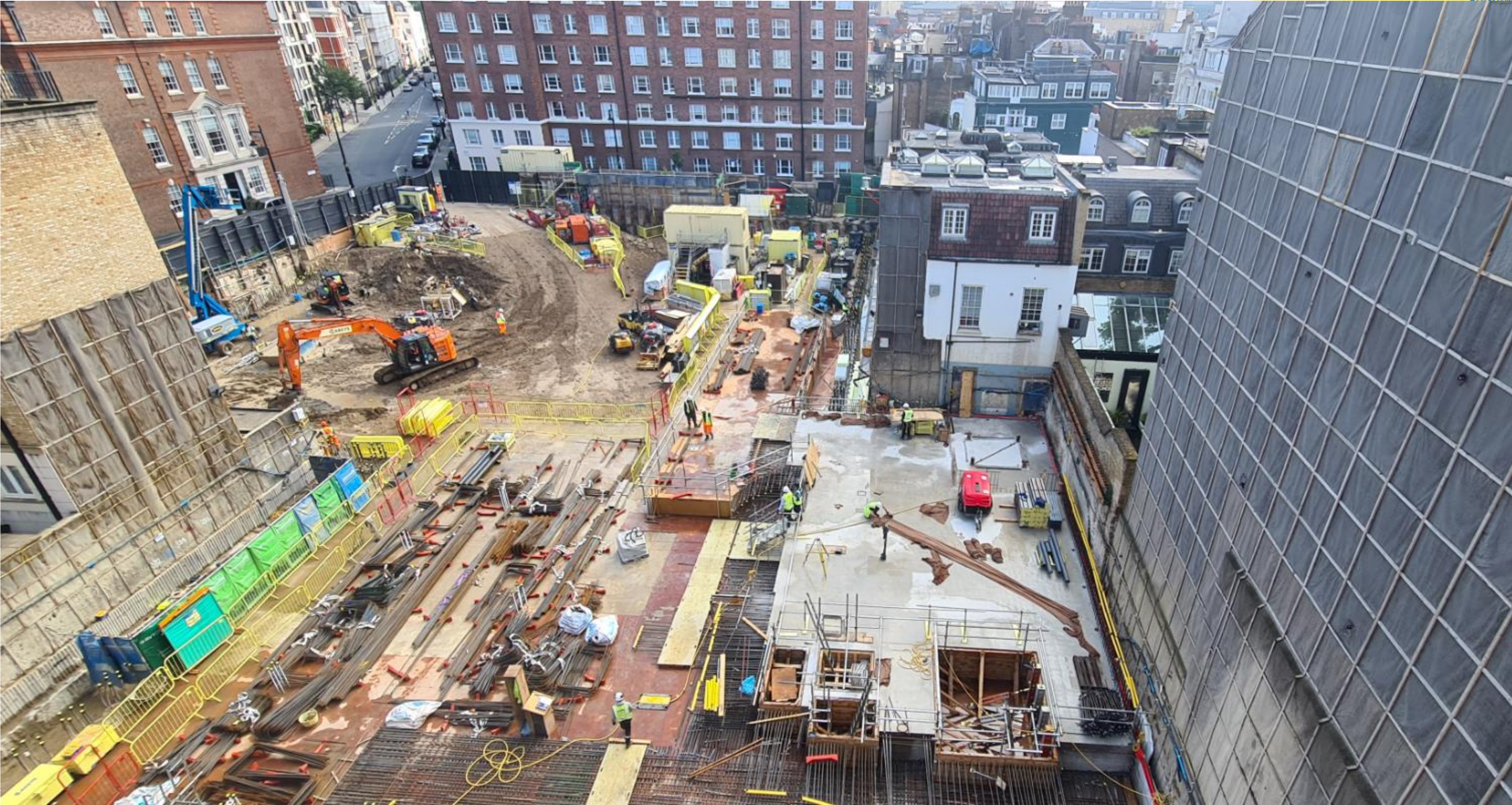
Typical completed concrete slab pour. (Location 3AS elevation)
