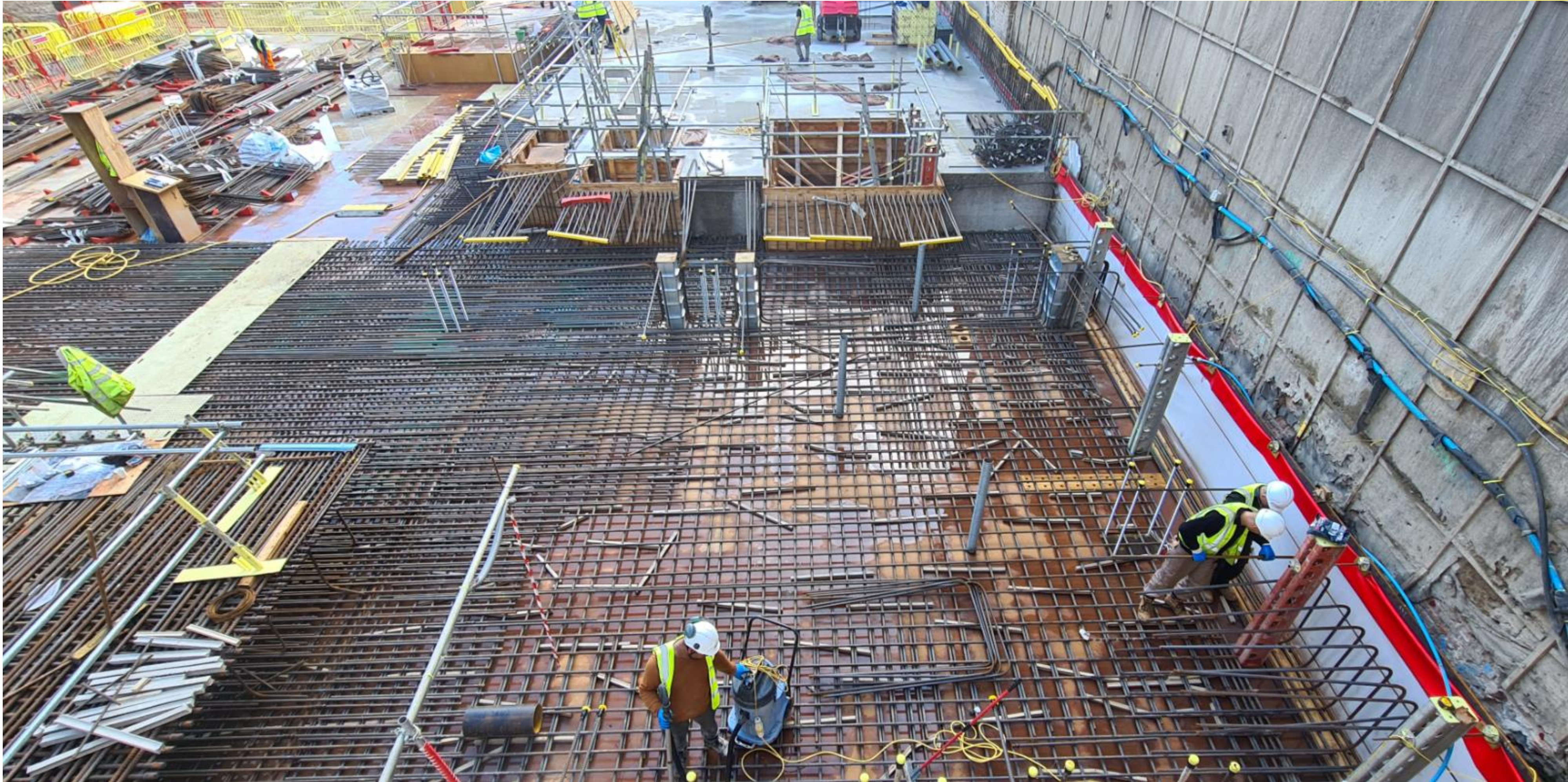
Typical steel fixing for slab construction along South Audley Square elevation.
