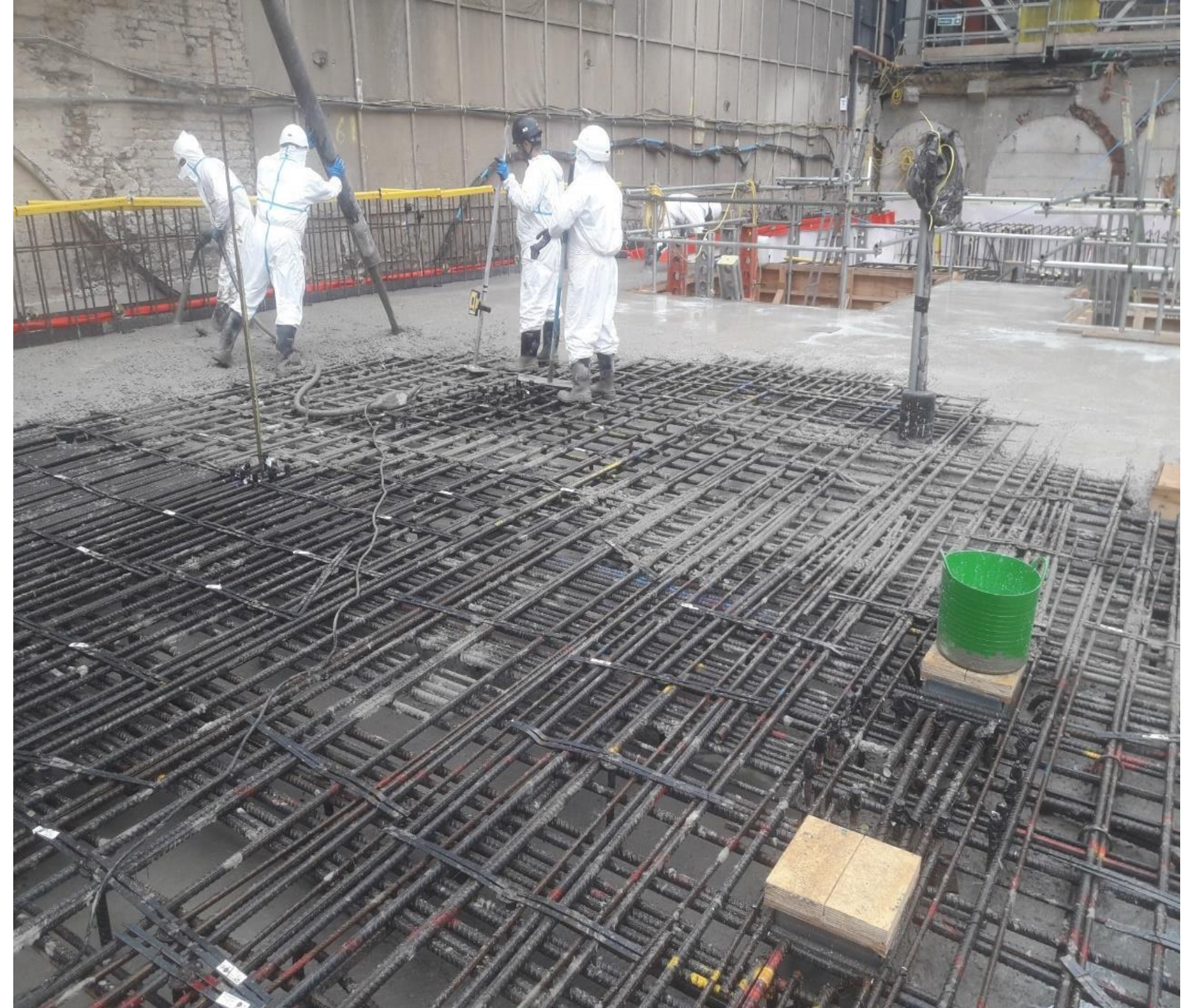
Team placing concrete using mobile concrete pump
