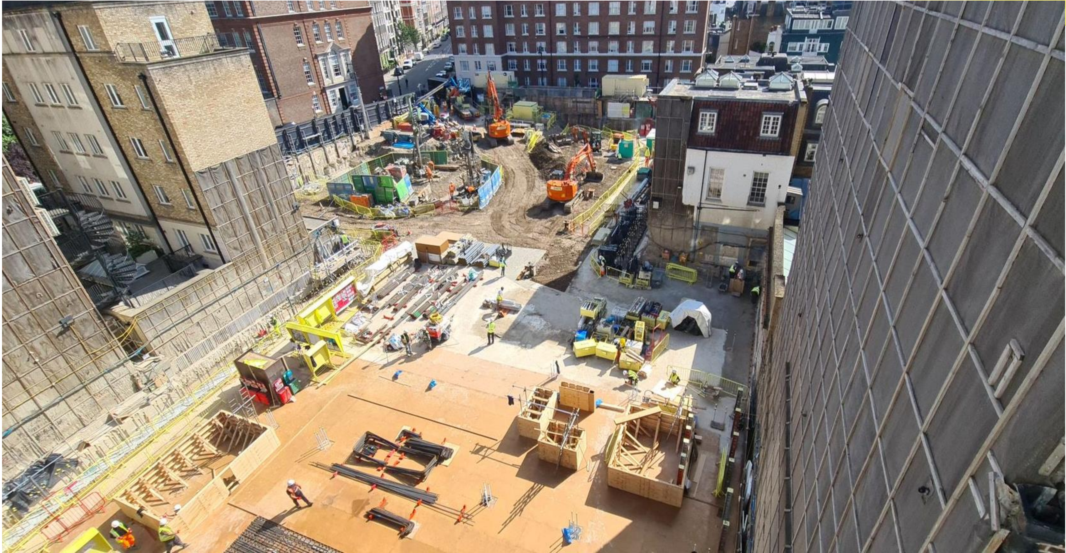
Concrete blinding complete in Zone 1. Slab Plywood installation ongoing.
