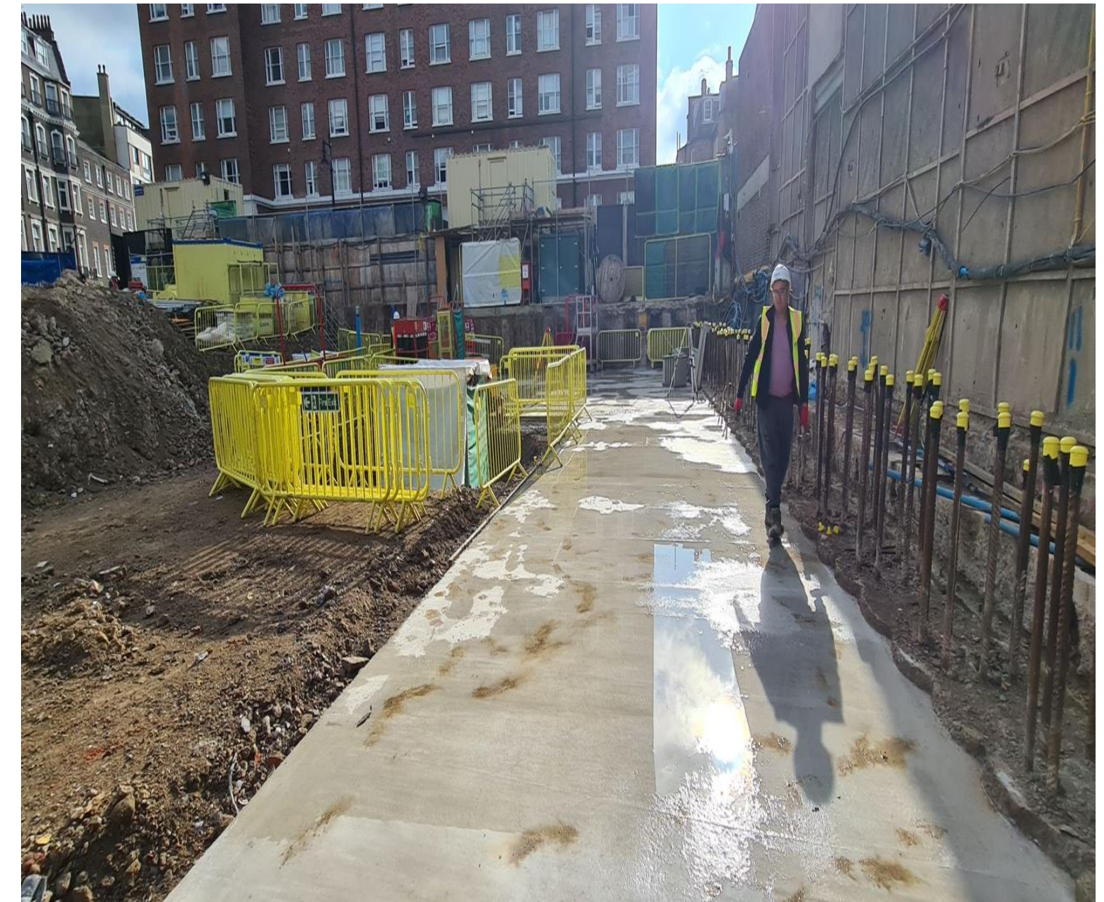
Slab preparation along Red Lion Yard elevation
