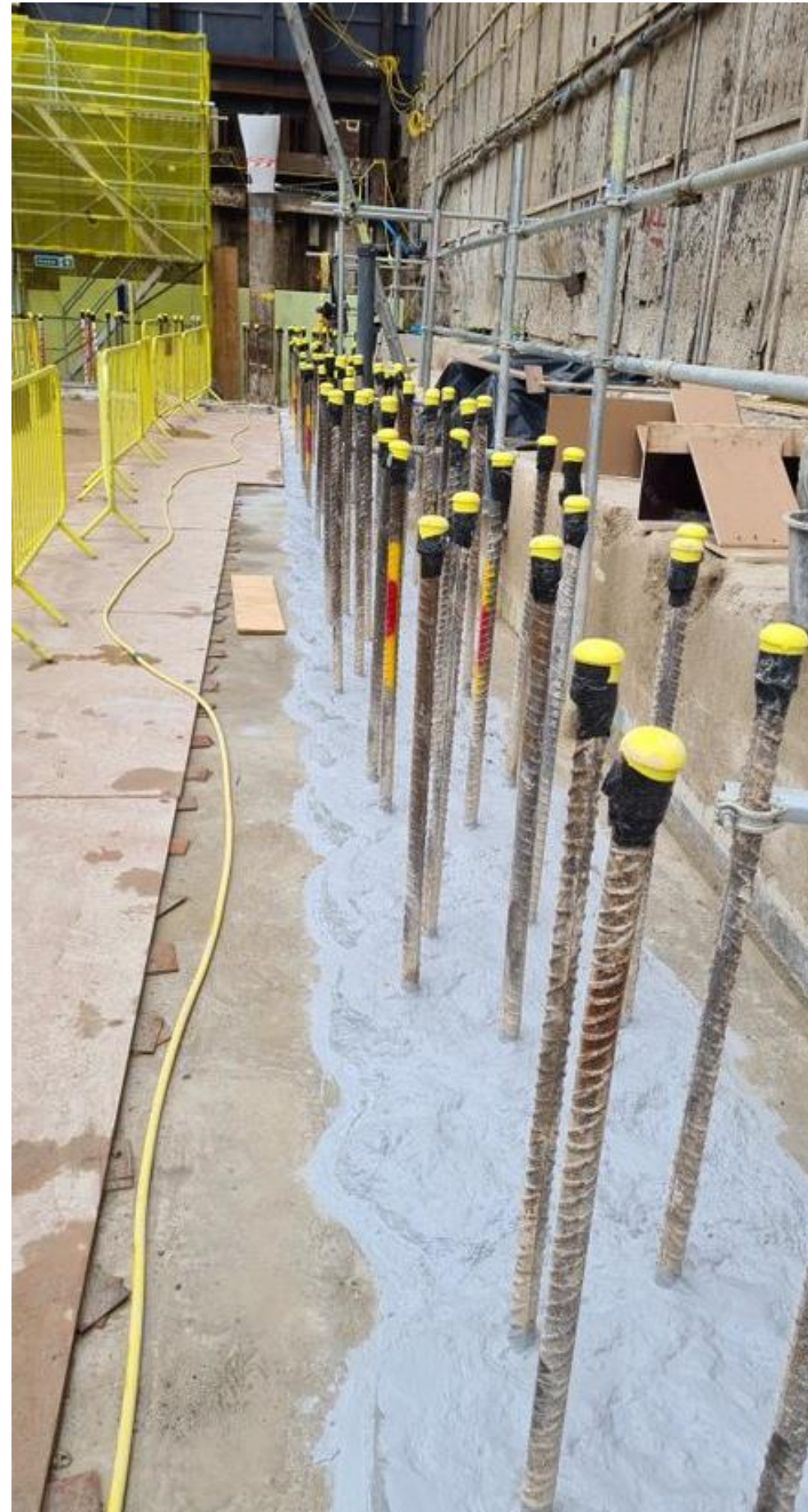
Typical waterproofing installation to piles
