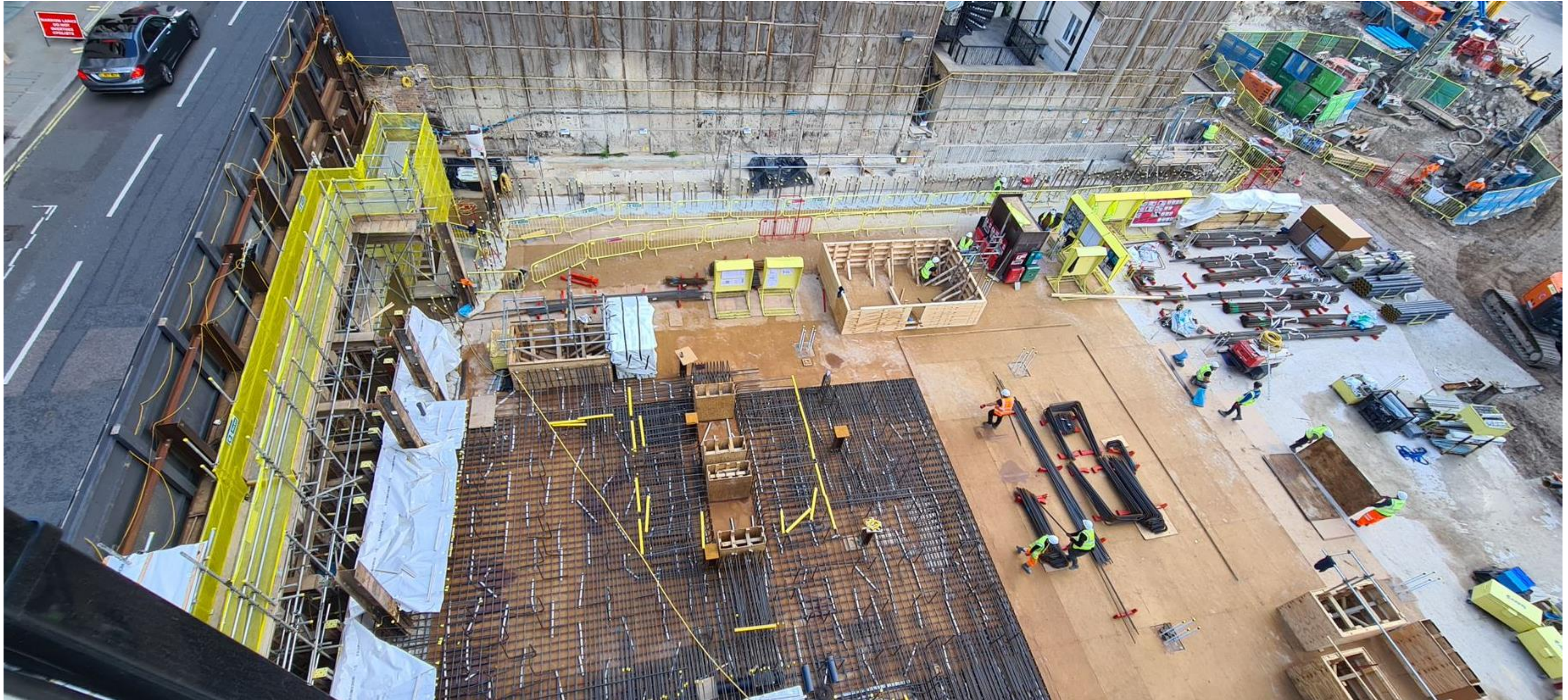
Plan View - Garden Level Slab reinforcement fixing to West of site
