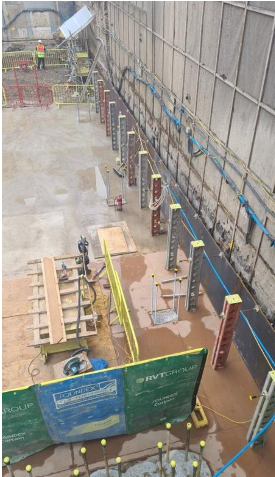
Typical slab formwork installation along 3 Audley Square
