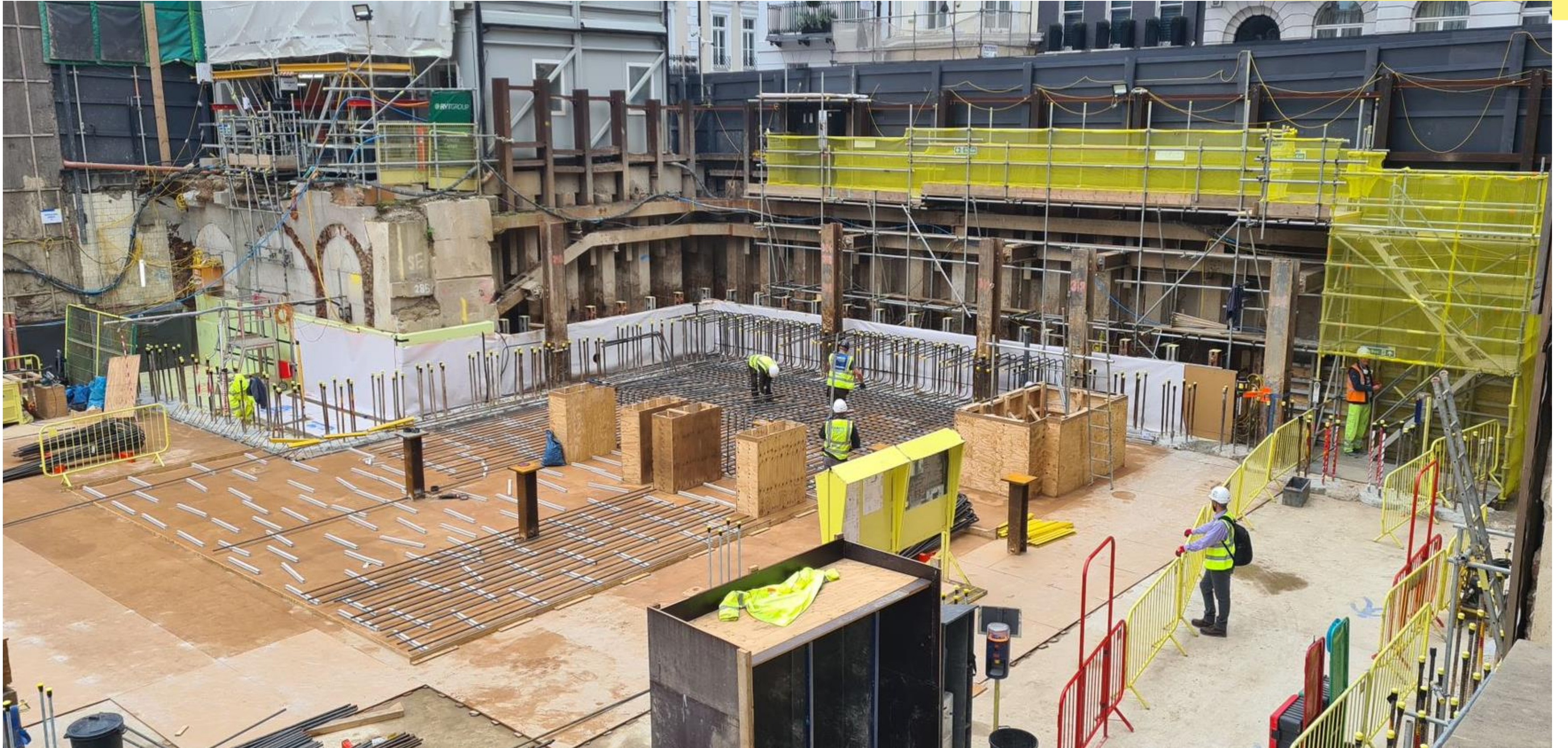
Garden Level Slab reinforcement fixing to West of site
