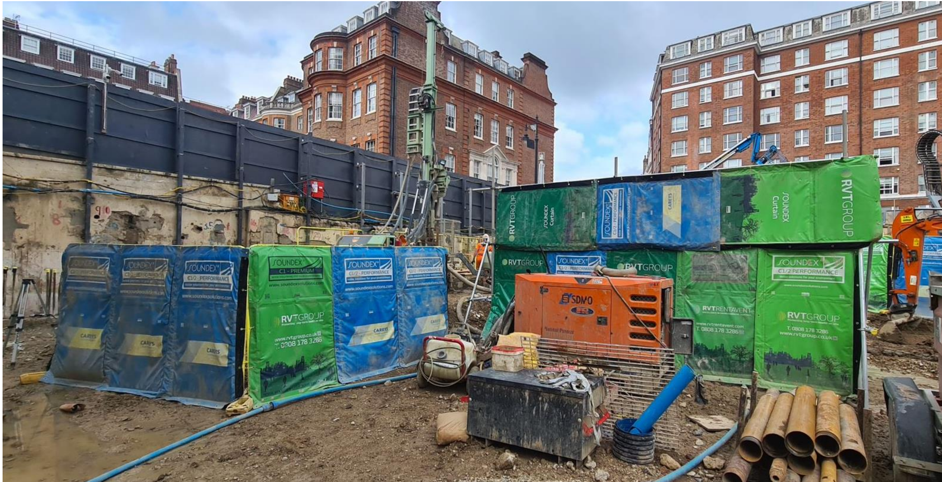
Ground Source Heat Pump Boreholes Ongoing – Surrounded by Acoustic Noise Barriers
