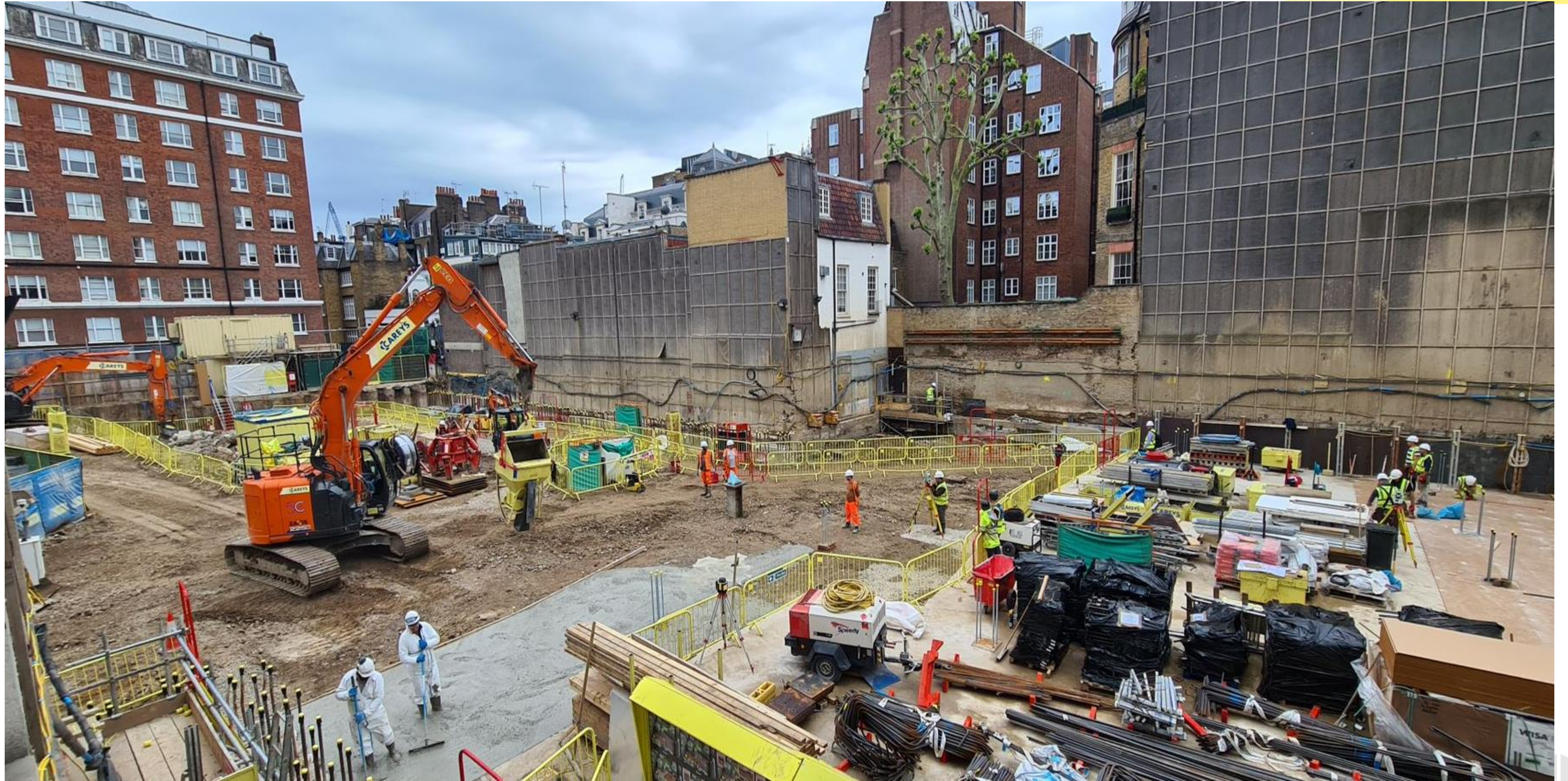
Pouring Concrete blinding for slab preparation
