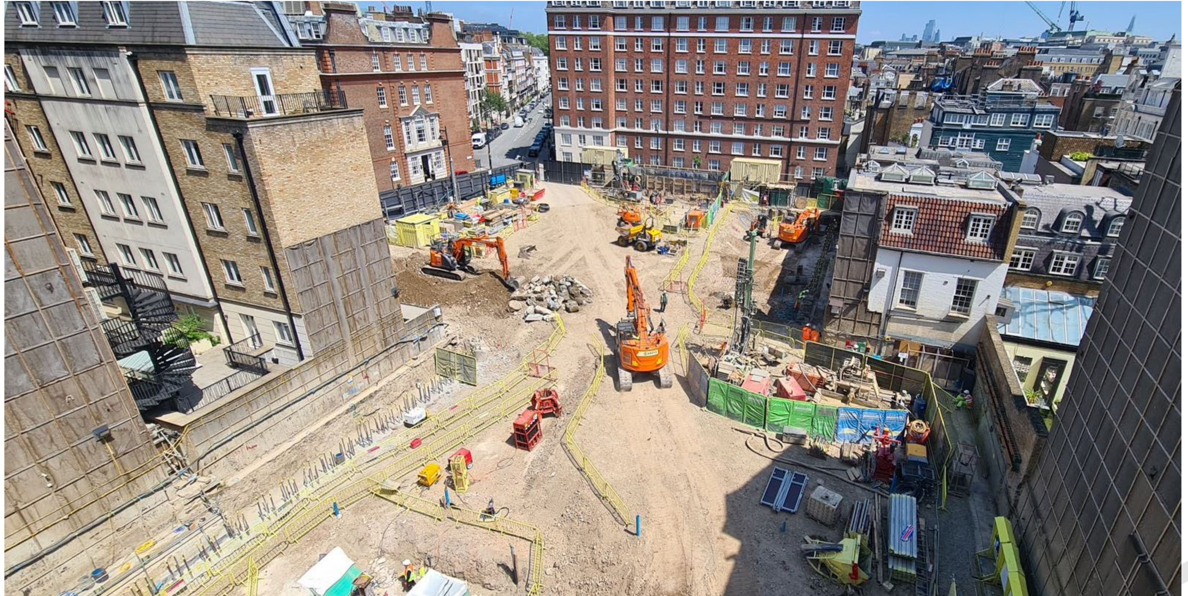
General Overview – Pile Cropping & Excavation
