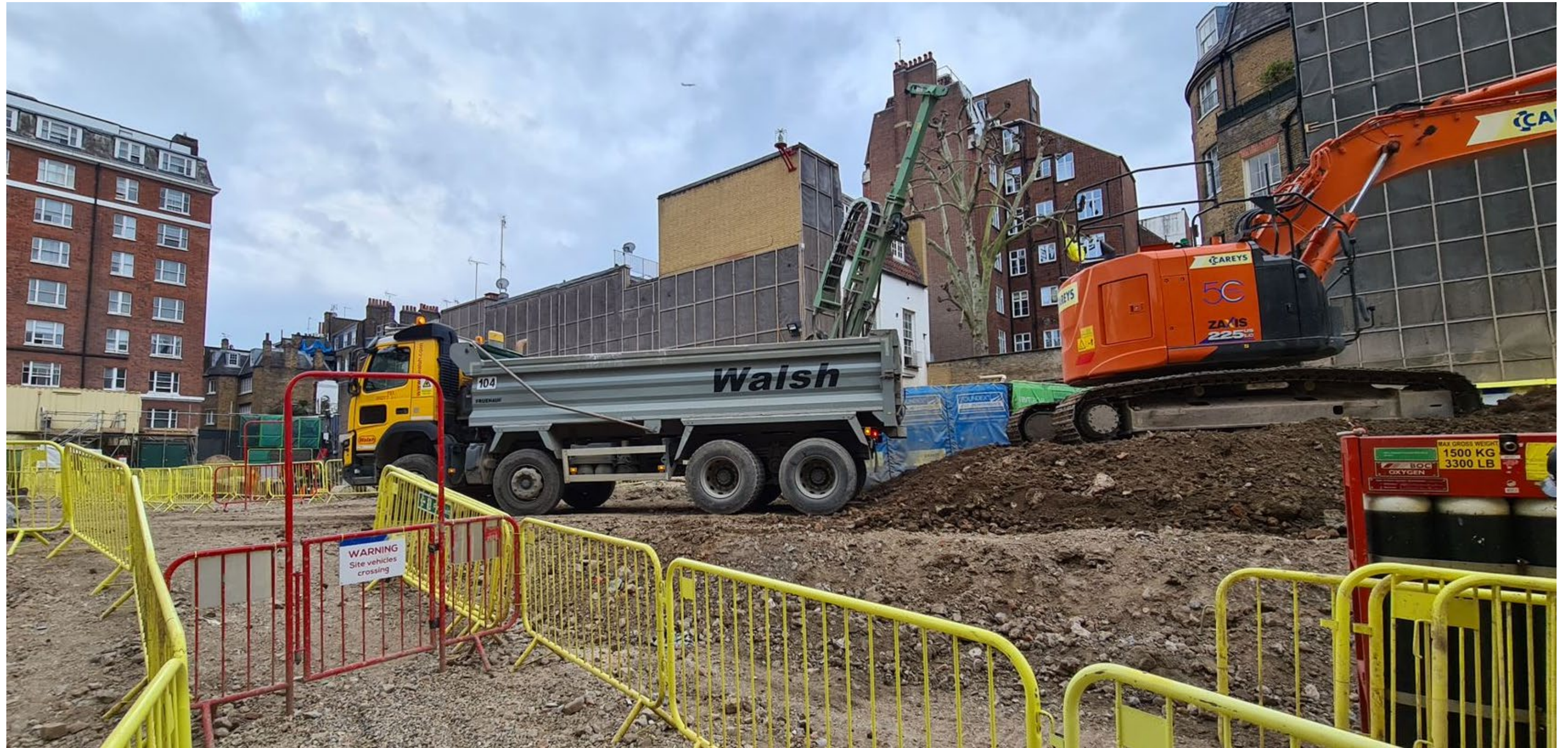
Removal of Spoil in Tipper Trucks
