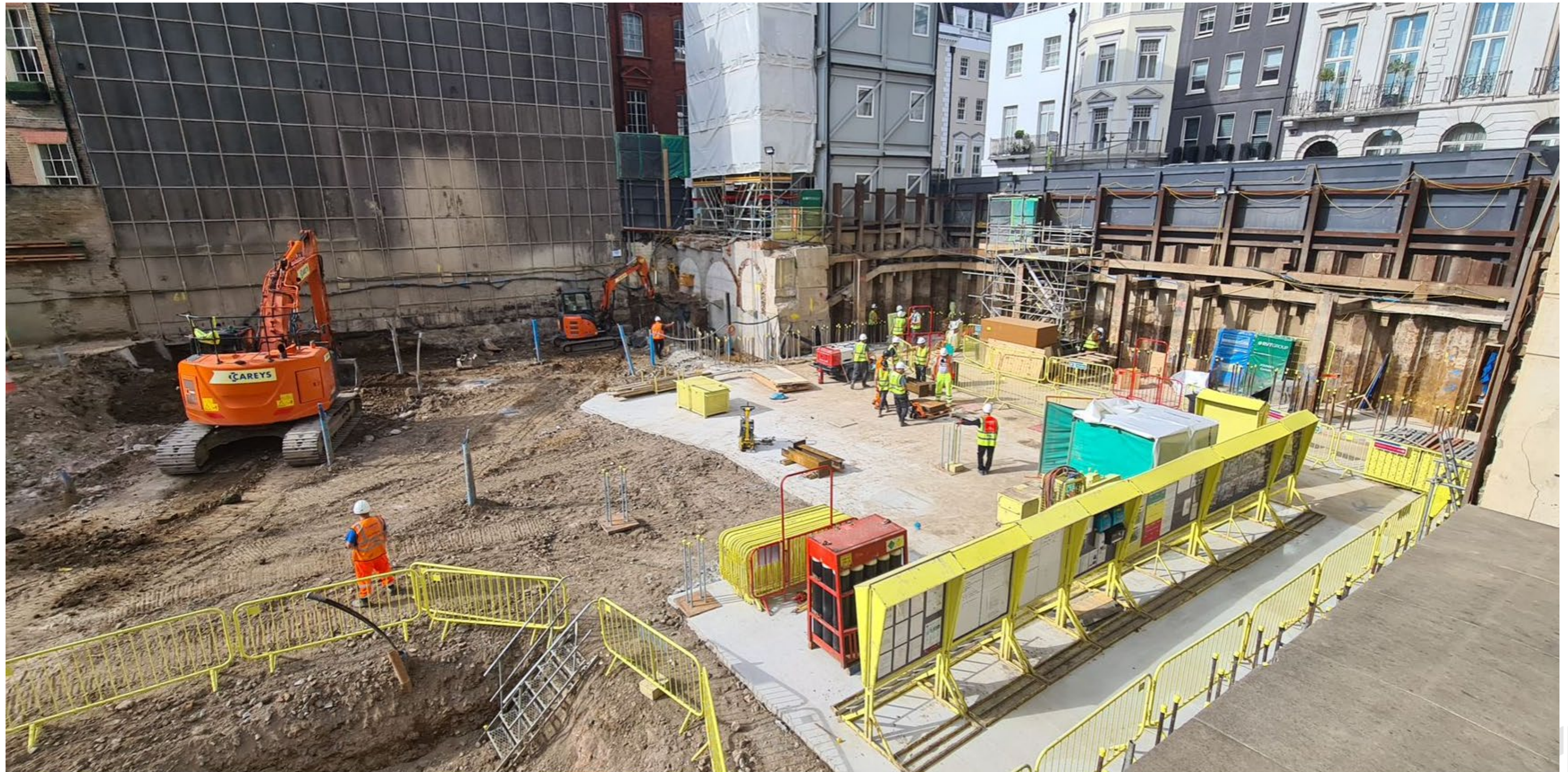
Preparation For Slab Construction
