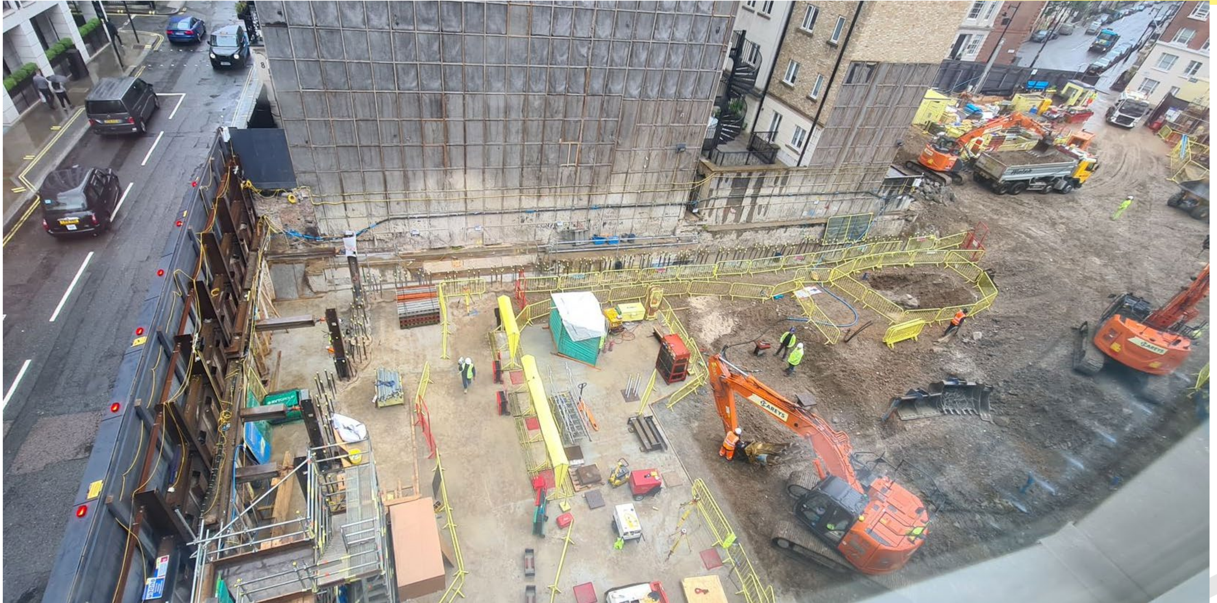
Commencement of GF Slab Construction to West Elevation of Site
