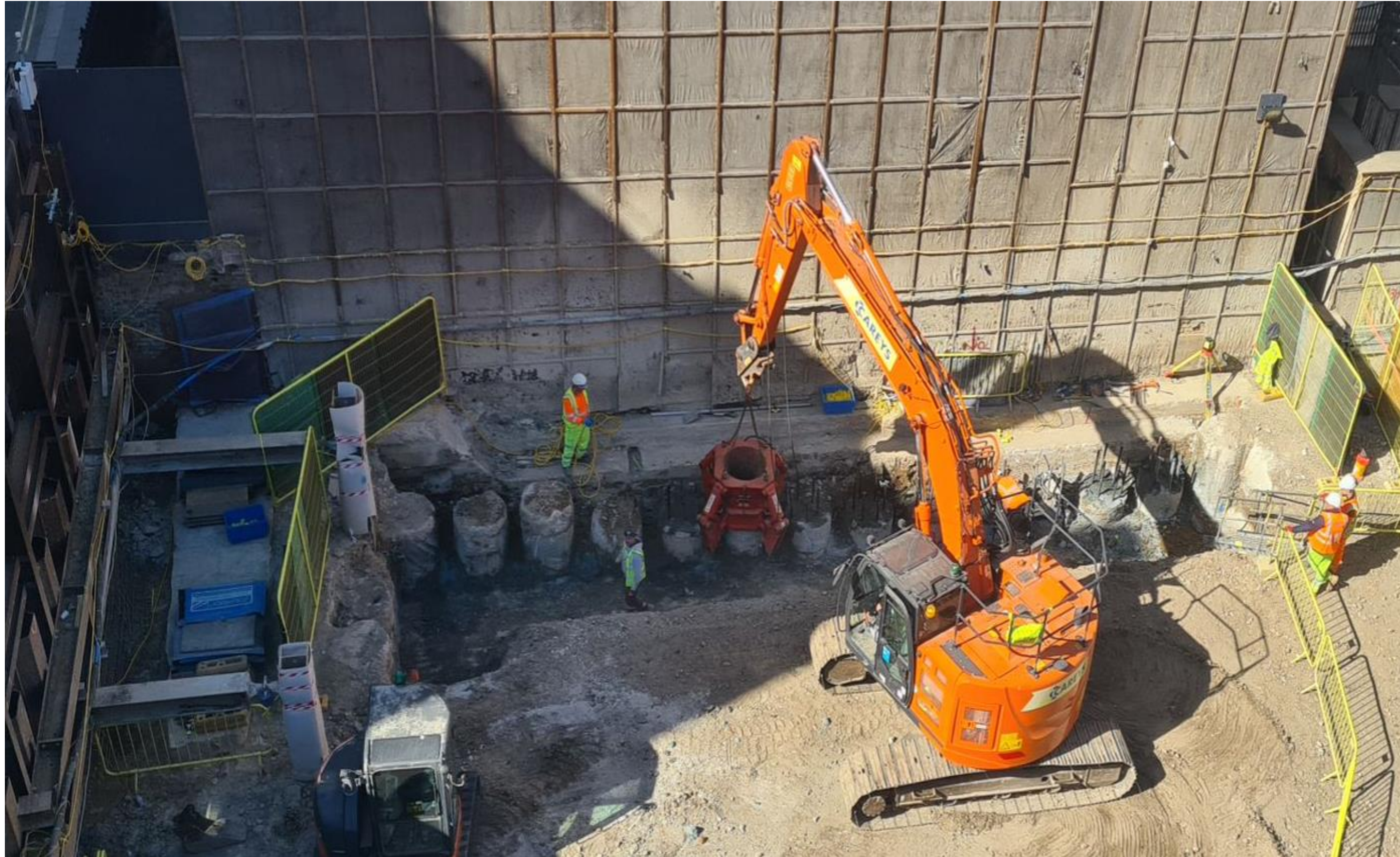
West Elevation of Site – Guidewall Removal & Pile Cropping
