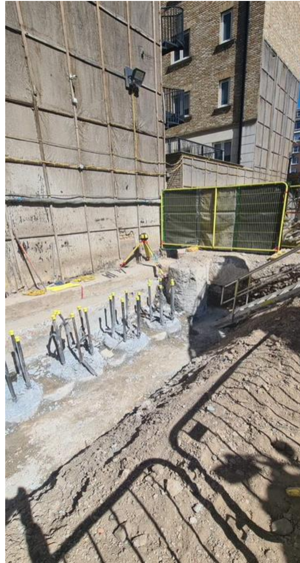
West Elevation of Site – Guidewall Removal & Pile Cropping Close to South Audley Street
