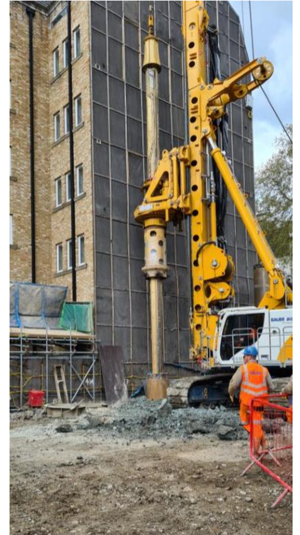
Rig Installing Last Remaining Secant Piles at 51 Hill Street
