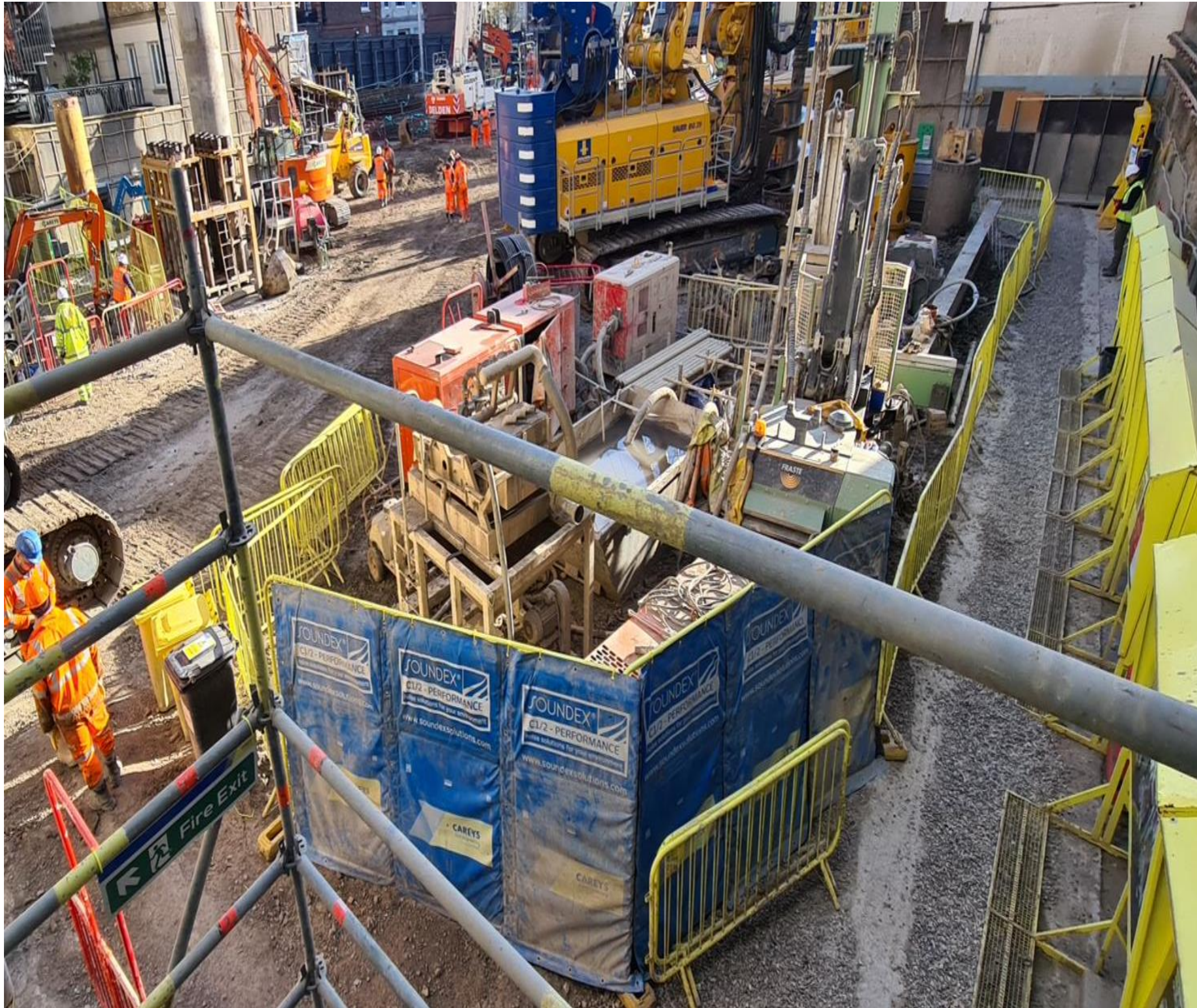
Typical GSHP Mini Piles – With Noise Barriers
