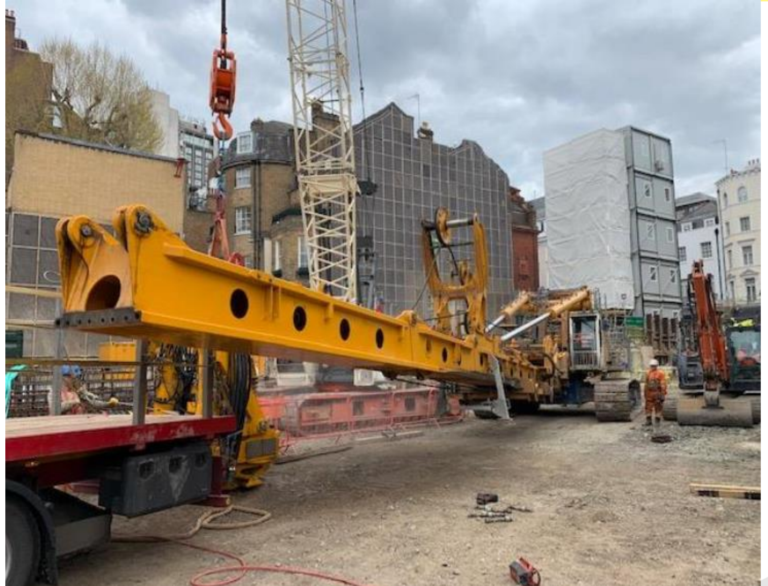
Demobilisation & Removal of Rigs /Cranes From Site
