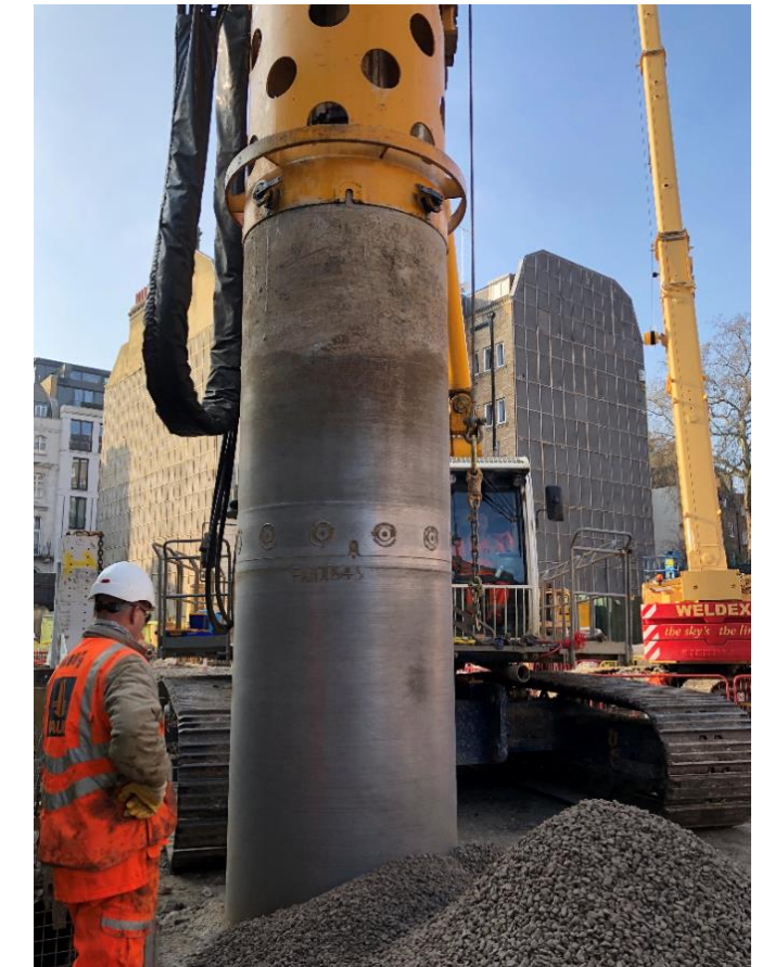
Extract Casing during concreting. Top up as required.
