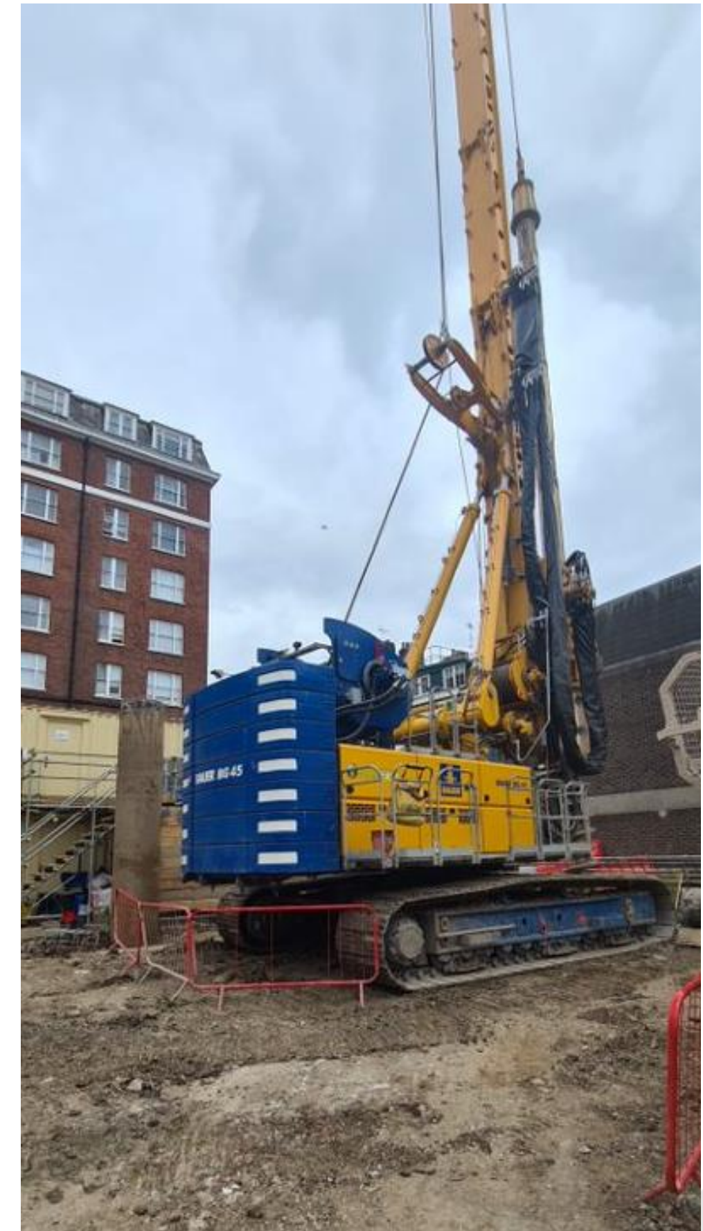
Rig Installing Secant Piles at Waverton Street
