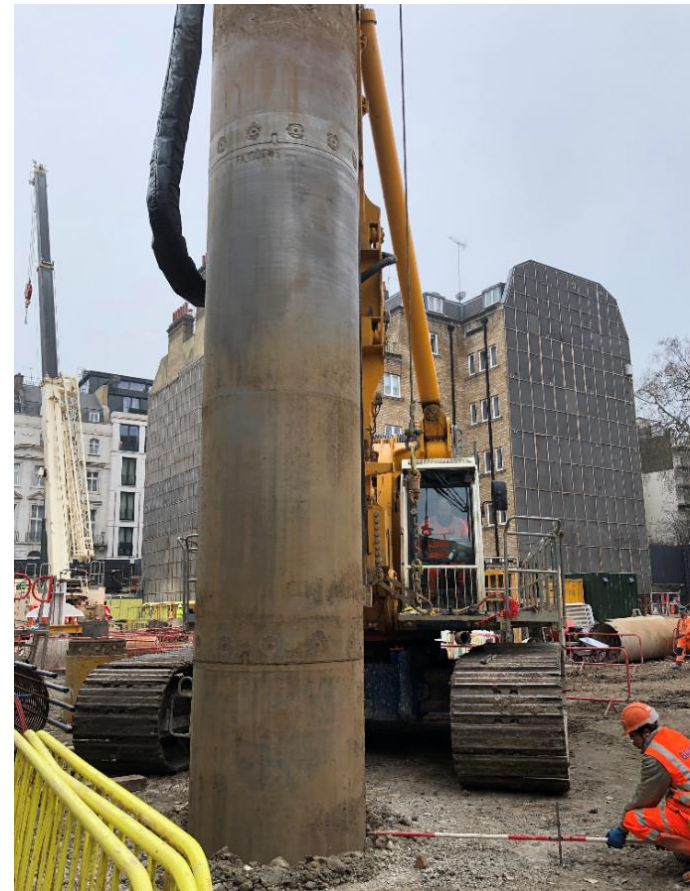
(1) Set Up at Pile Position
