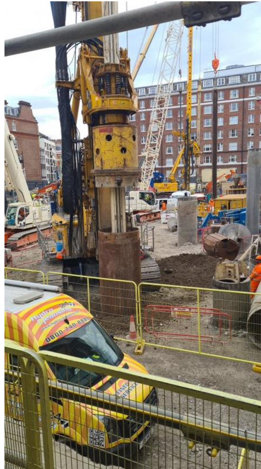
Rig – Installing New Internal Bearing Piles To West of Site
