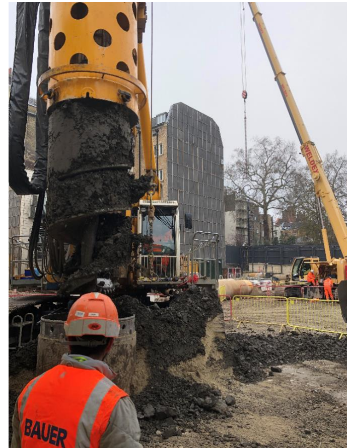
(2) Install Casing & Drilling to cut off level (2 hrs)
