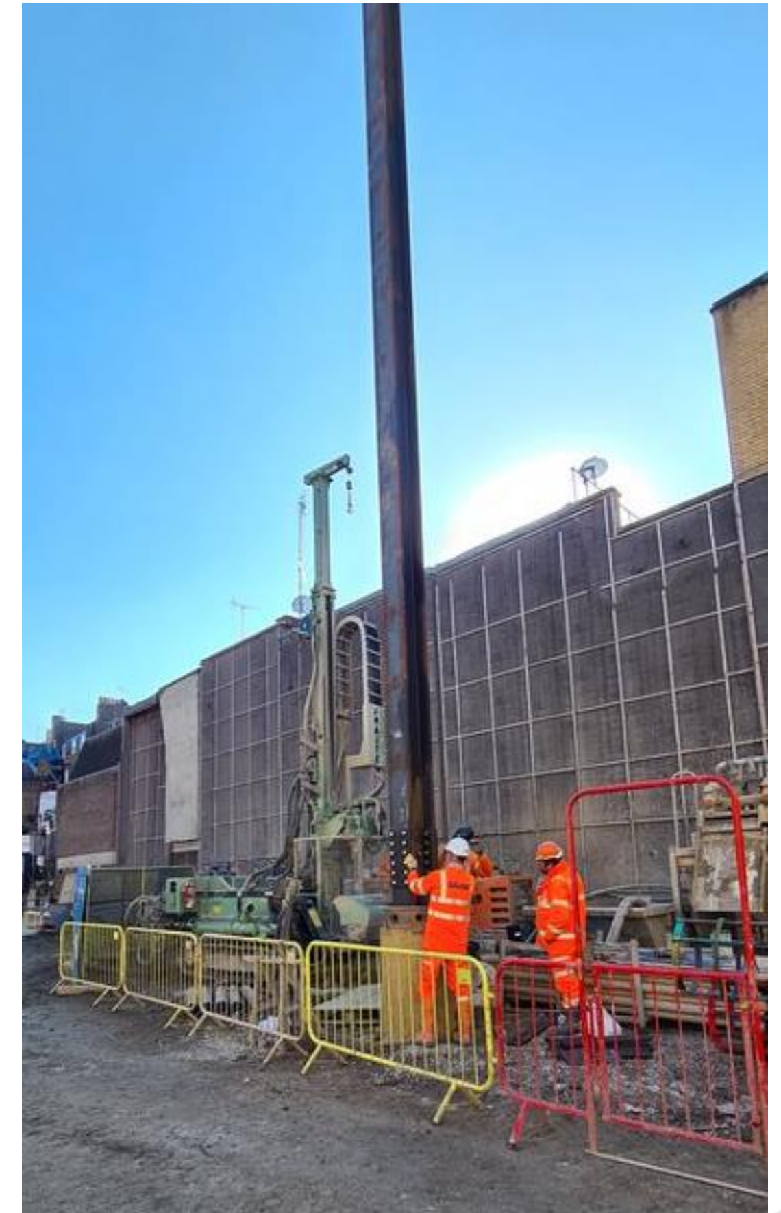
Installing plunge steel into Pile
