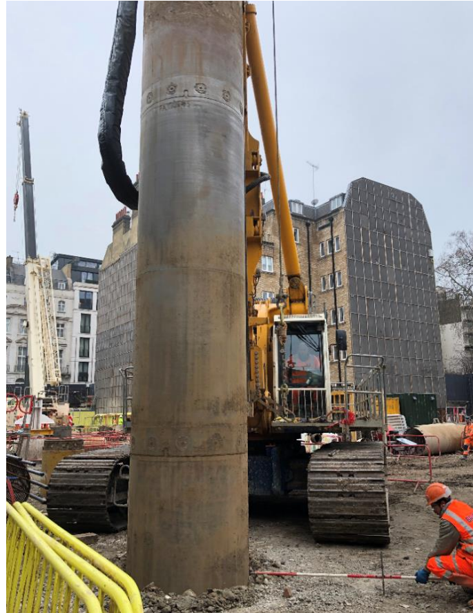
(1) Set Up at Pile Position
