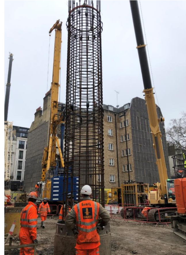
** (3) Progress to Pile Toe and clean base. Install reinforcement cage (4.5 hrs)
