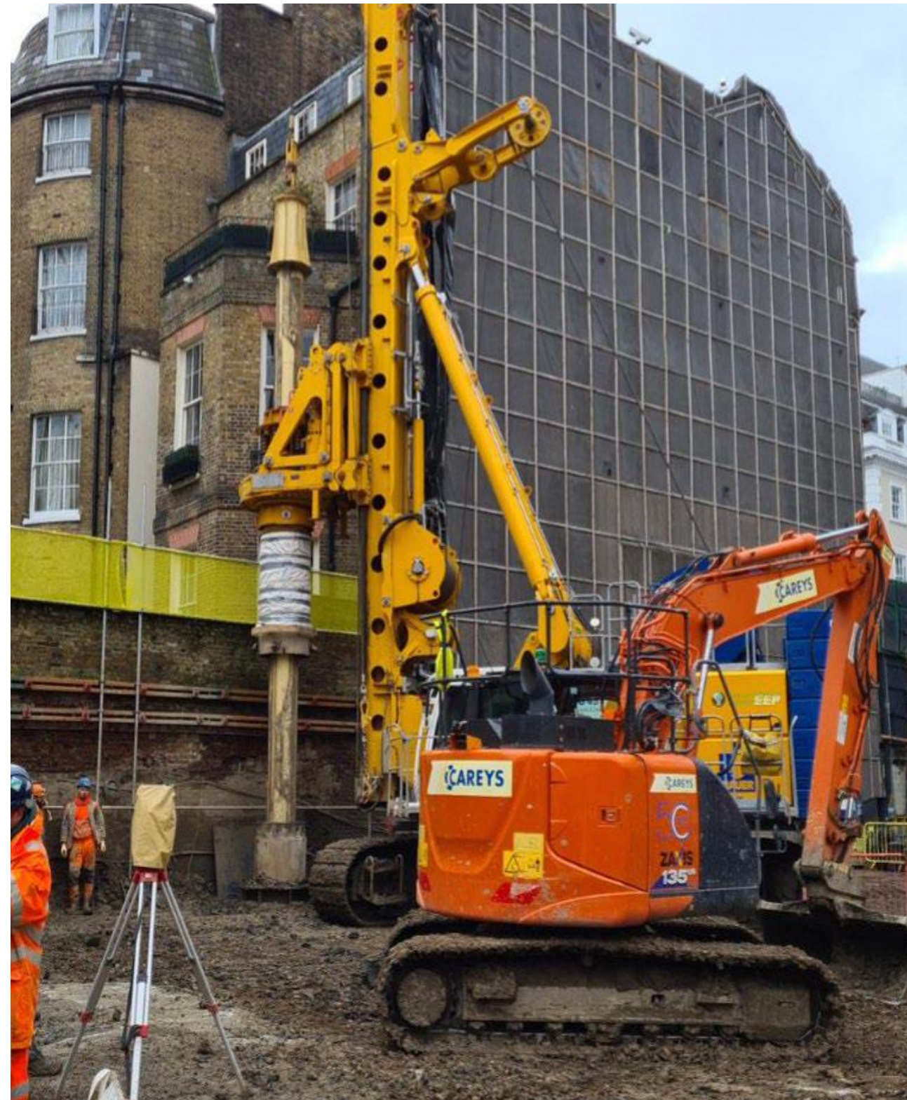
Rig – Installing New Perimeter Secant Piles To South of Site
