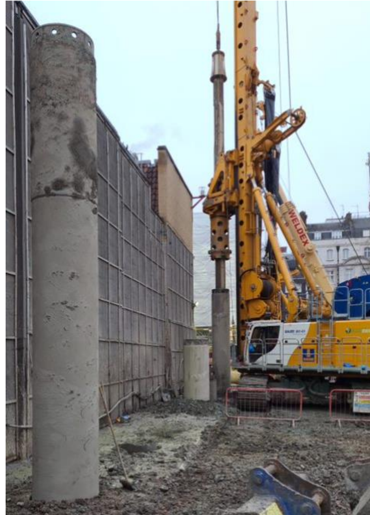
Rig – Installing New Perimeter Secant Piles To South of Site
