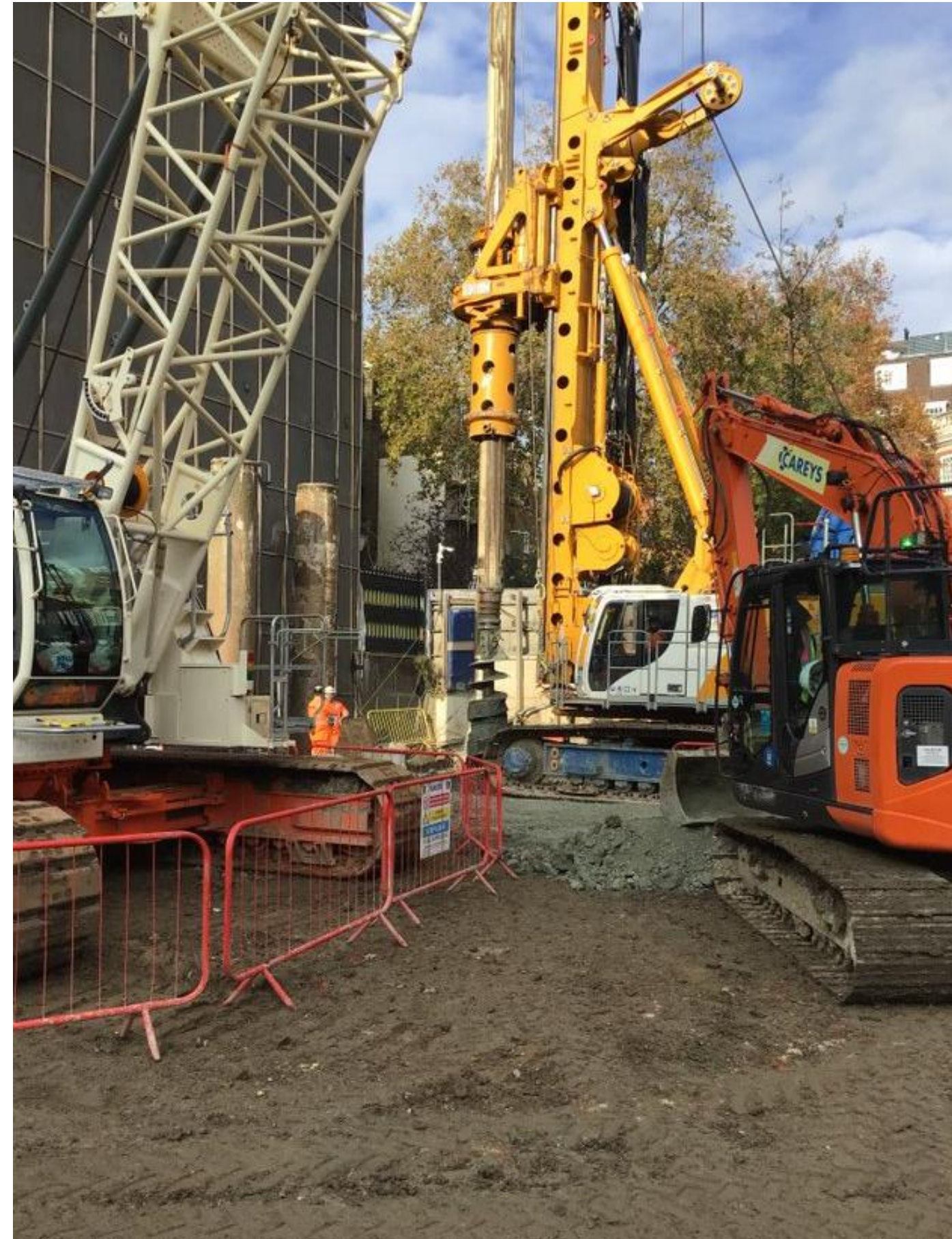
Rig 2 – Installing New Perimeter Secant Piles To East of Site
