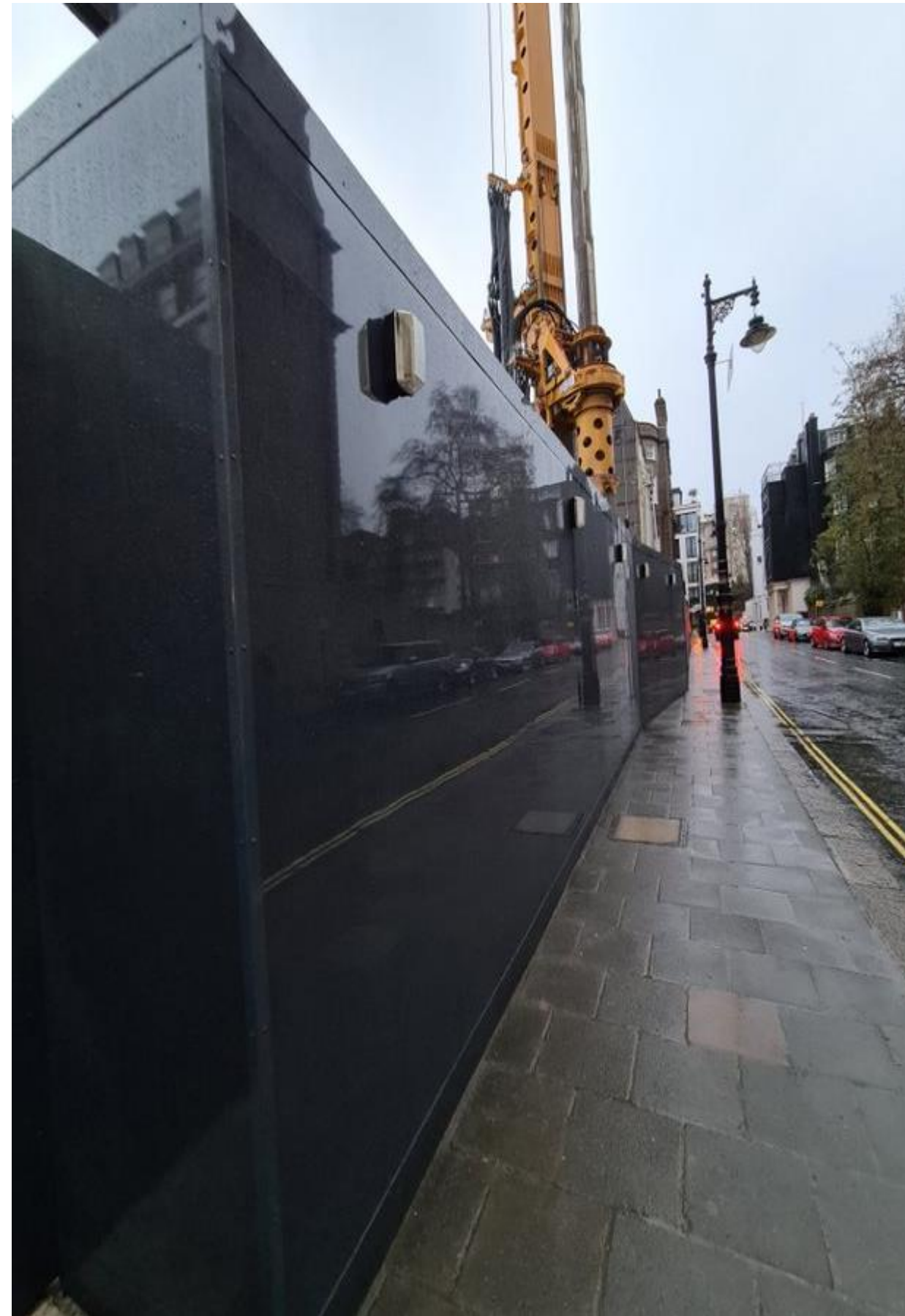
Dibond Sheetting Installed to Hoarding
