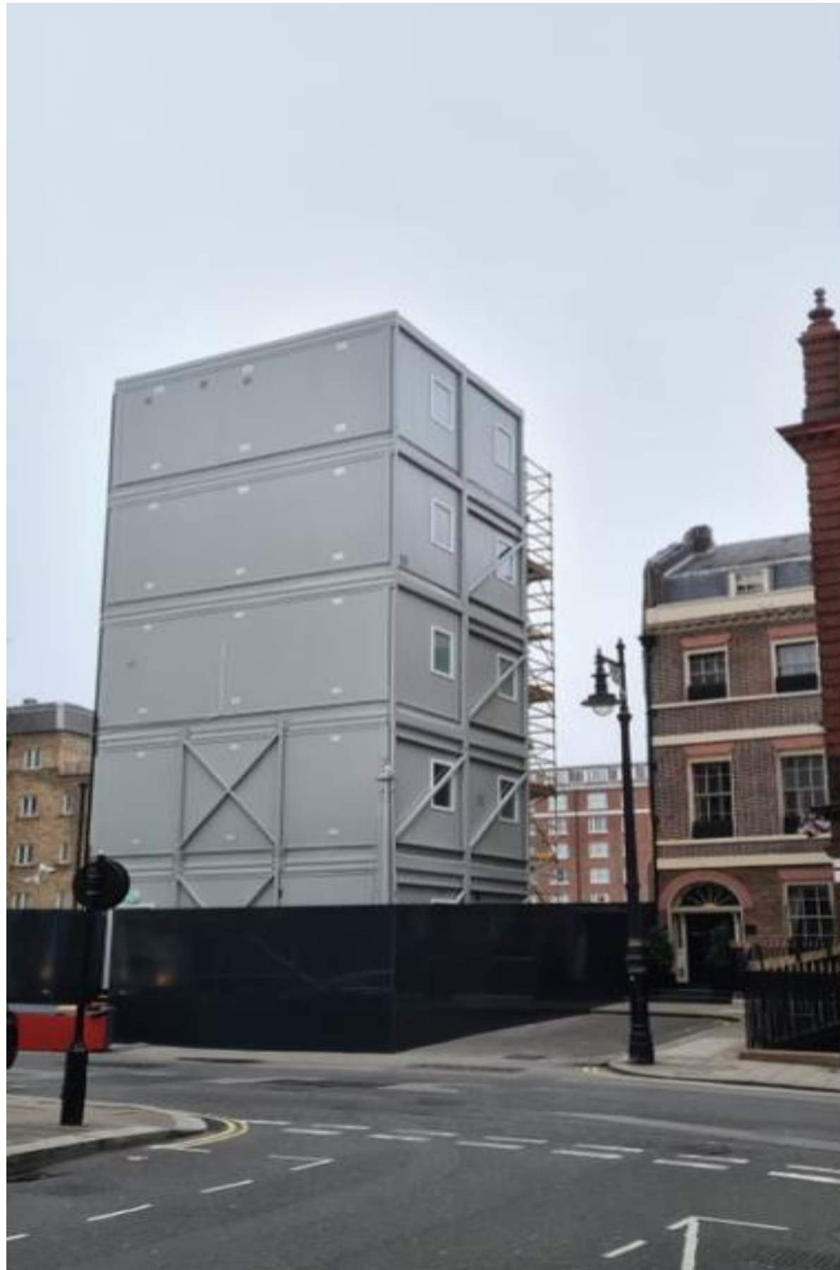
Modular Welfare Cabins on South Audley Street Installed
