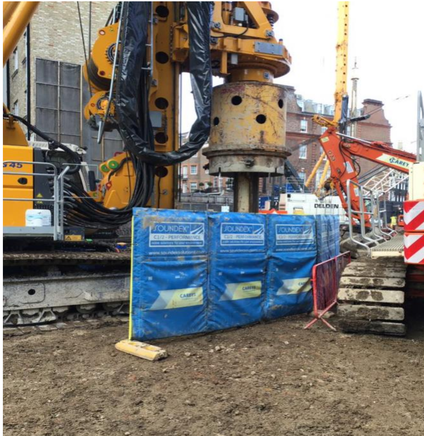
Slab Concrete Core Works In Action
