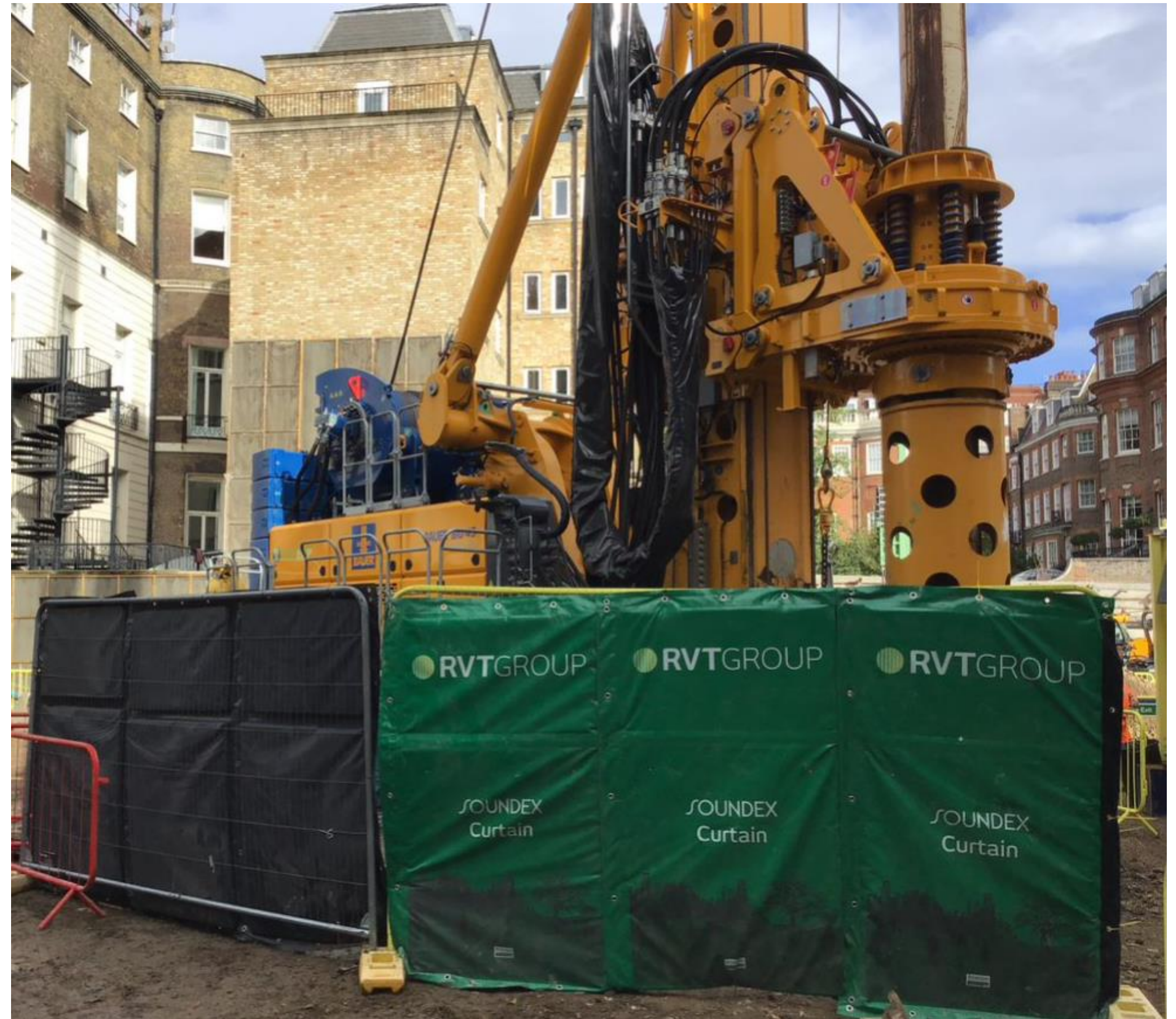
Existing Spine Beam Concrete Coring Works In Action (Inc Noise Barriers)
