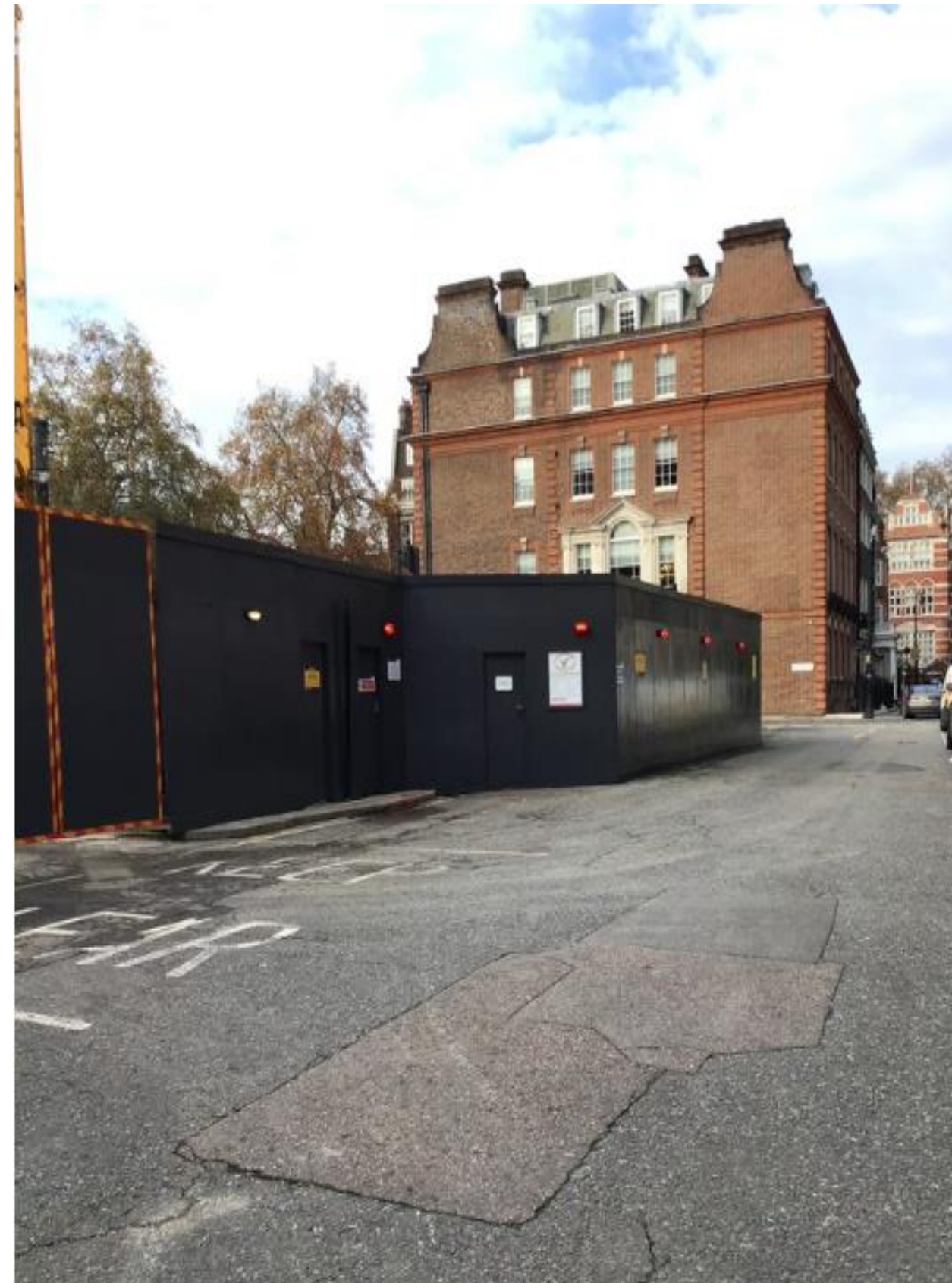
Perimeter Hoarding Increased to 3m in Height on Waverton Street, Hill Street & South Audley Street To Reduce Noise Output
