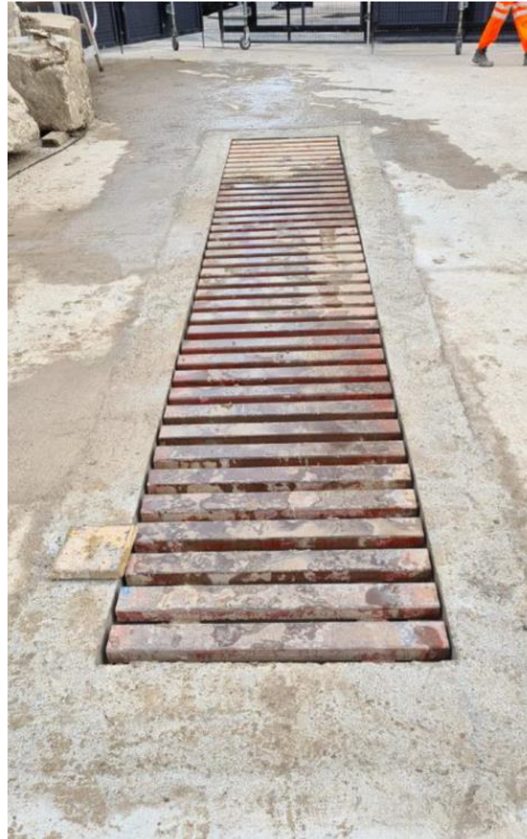
Installation of Wheel Wash Grillage at Gate 1 & 2 – Washing Area To keep Vehicle Wheels and Surrounding Roads Clean
