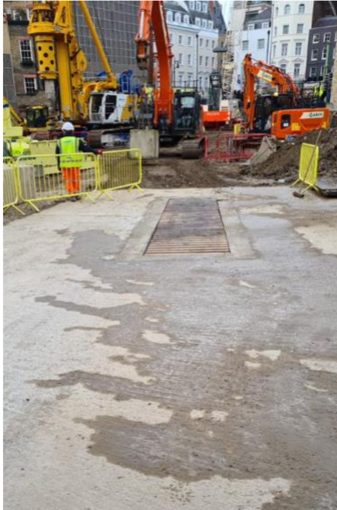
Installation of Wheel Wash Grillage – Washing Area To keep Vehicle Wheels and Surrounding Roads Clean
