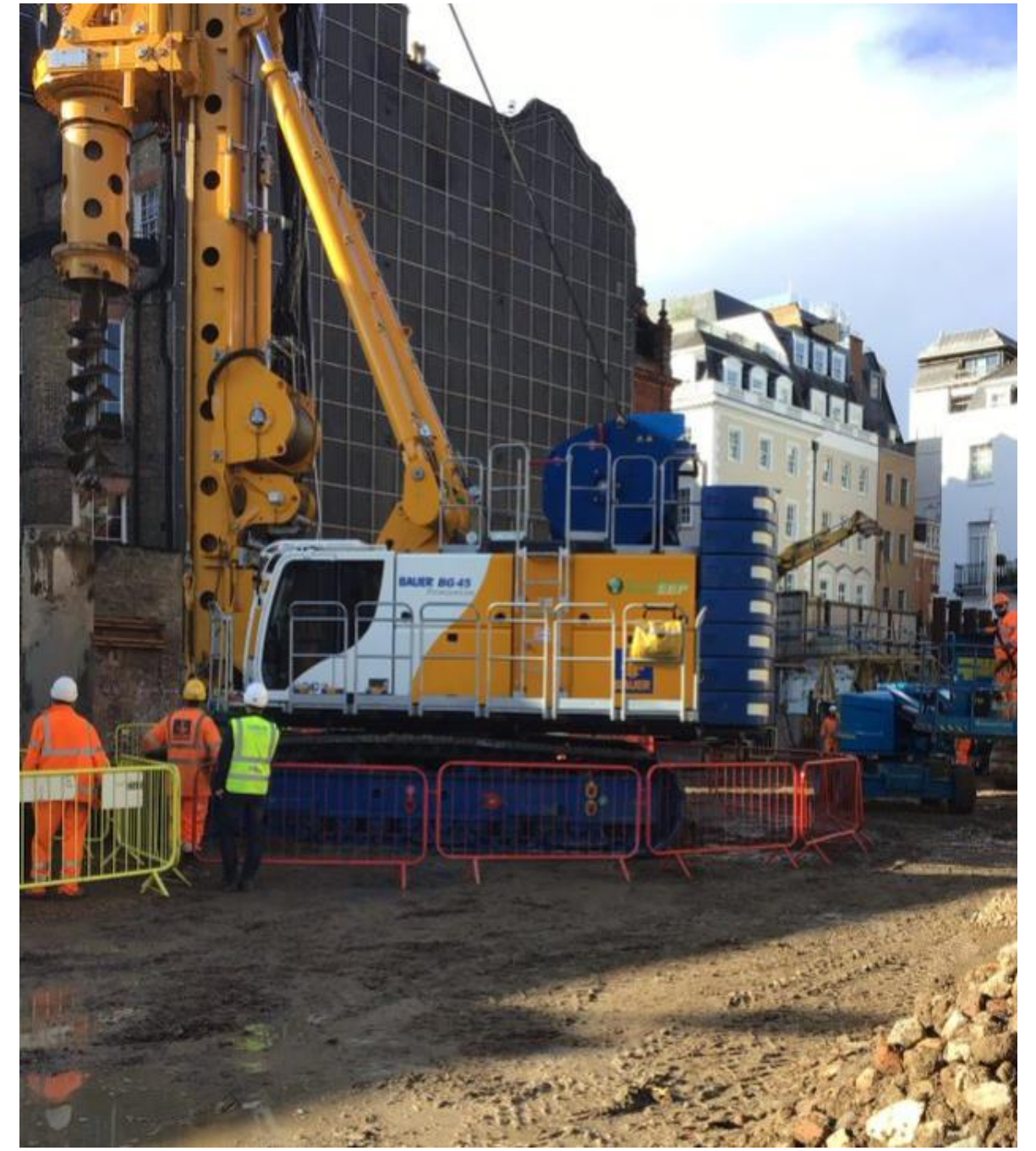
Pile Auguring In Action
