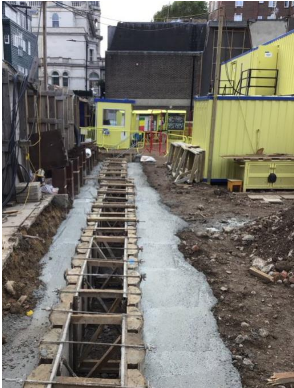
Guidewall Construction
