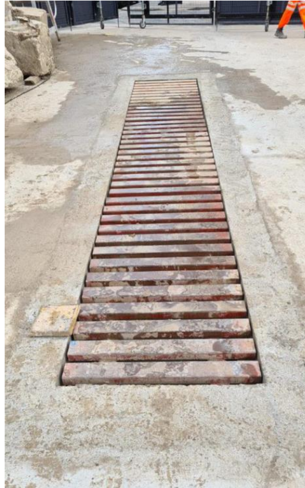
Installation of Wheel Wash Grillage – Washing Area To keep Vehicle Wheels and Surrounding Roads Clean
