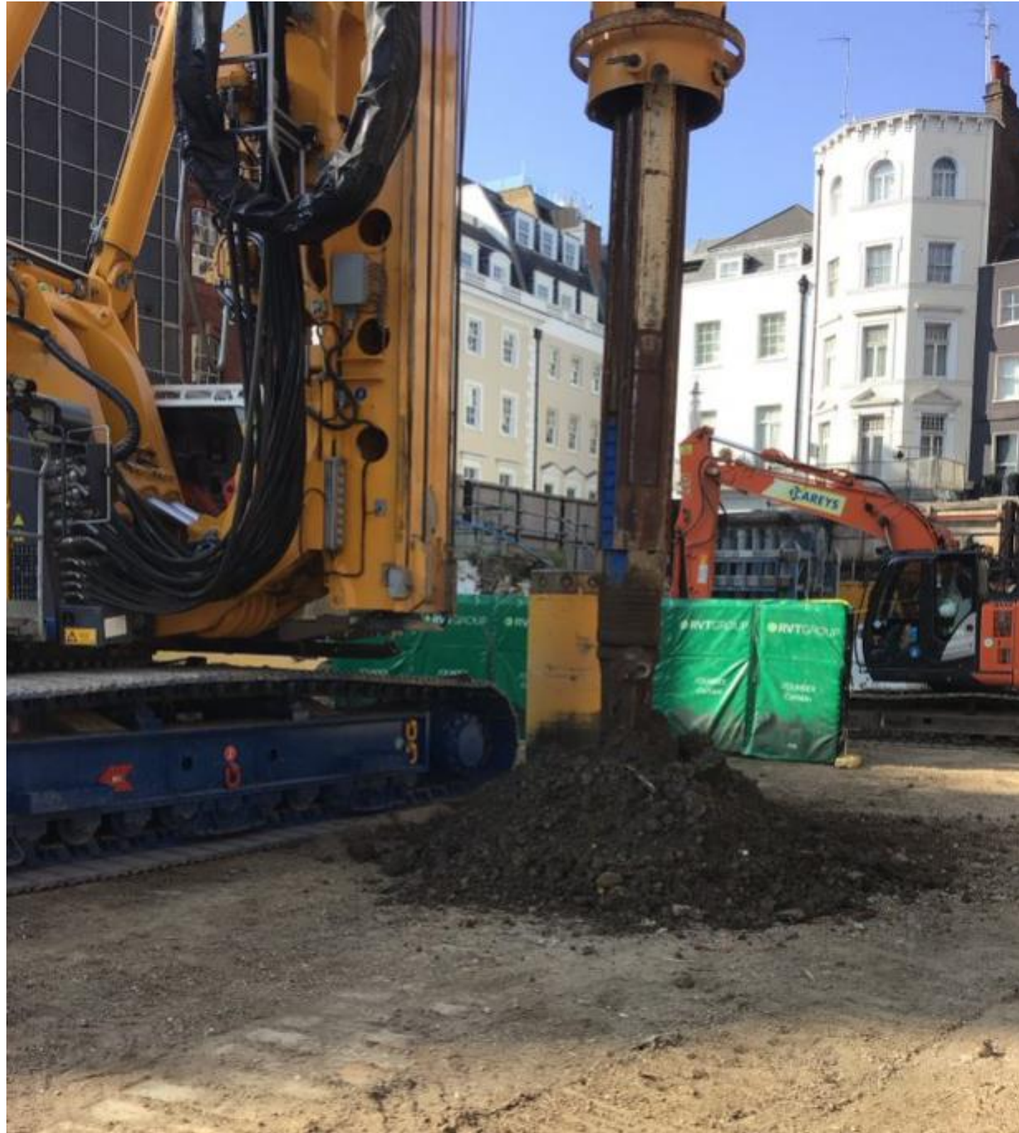
Slab Core Works In Action
