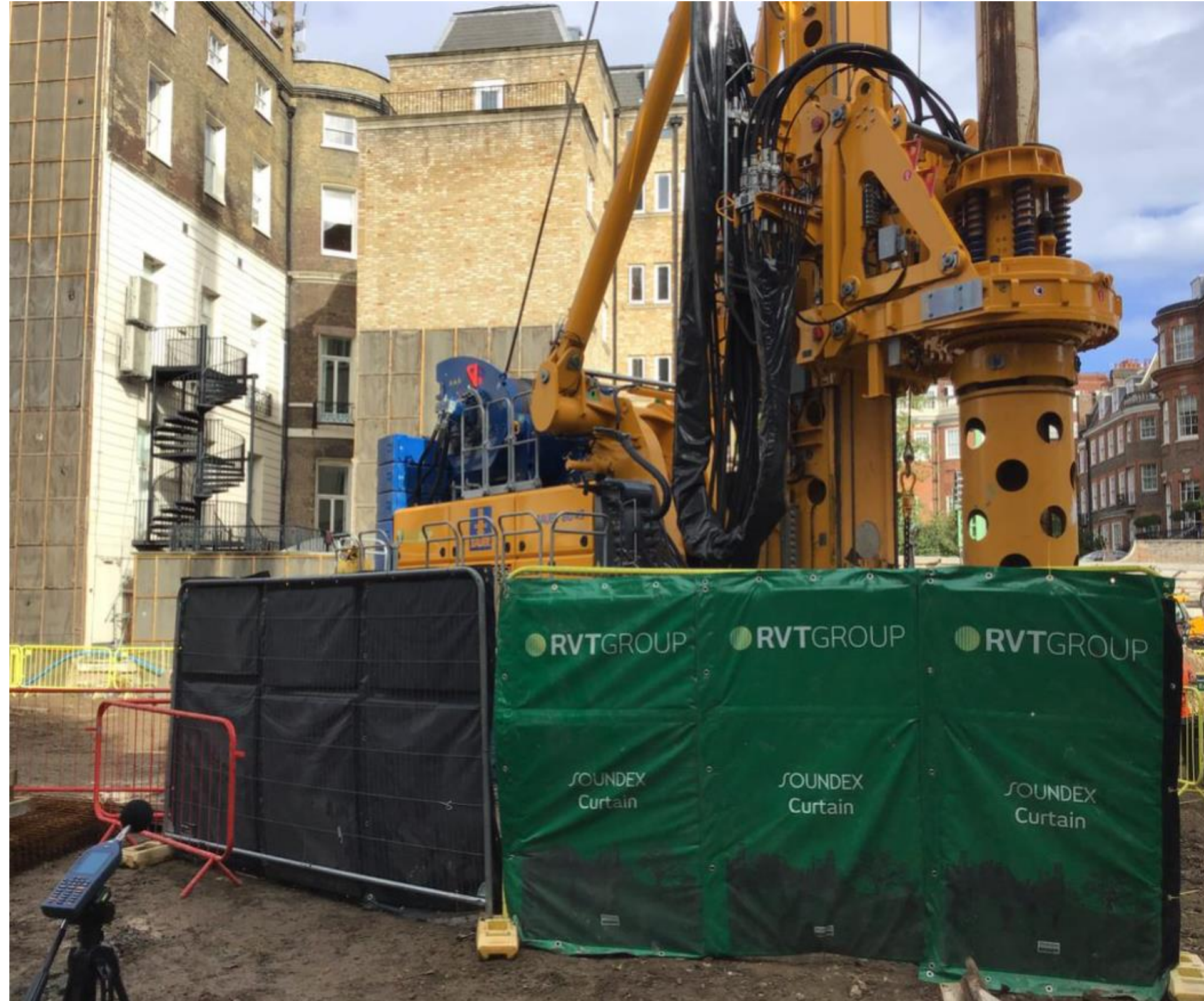
Existing Pile Coring Works In Action (Inc Noise Barriers)
