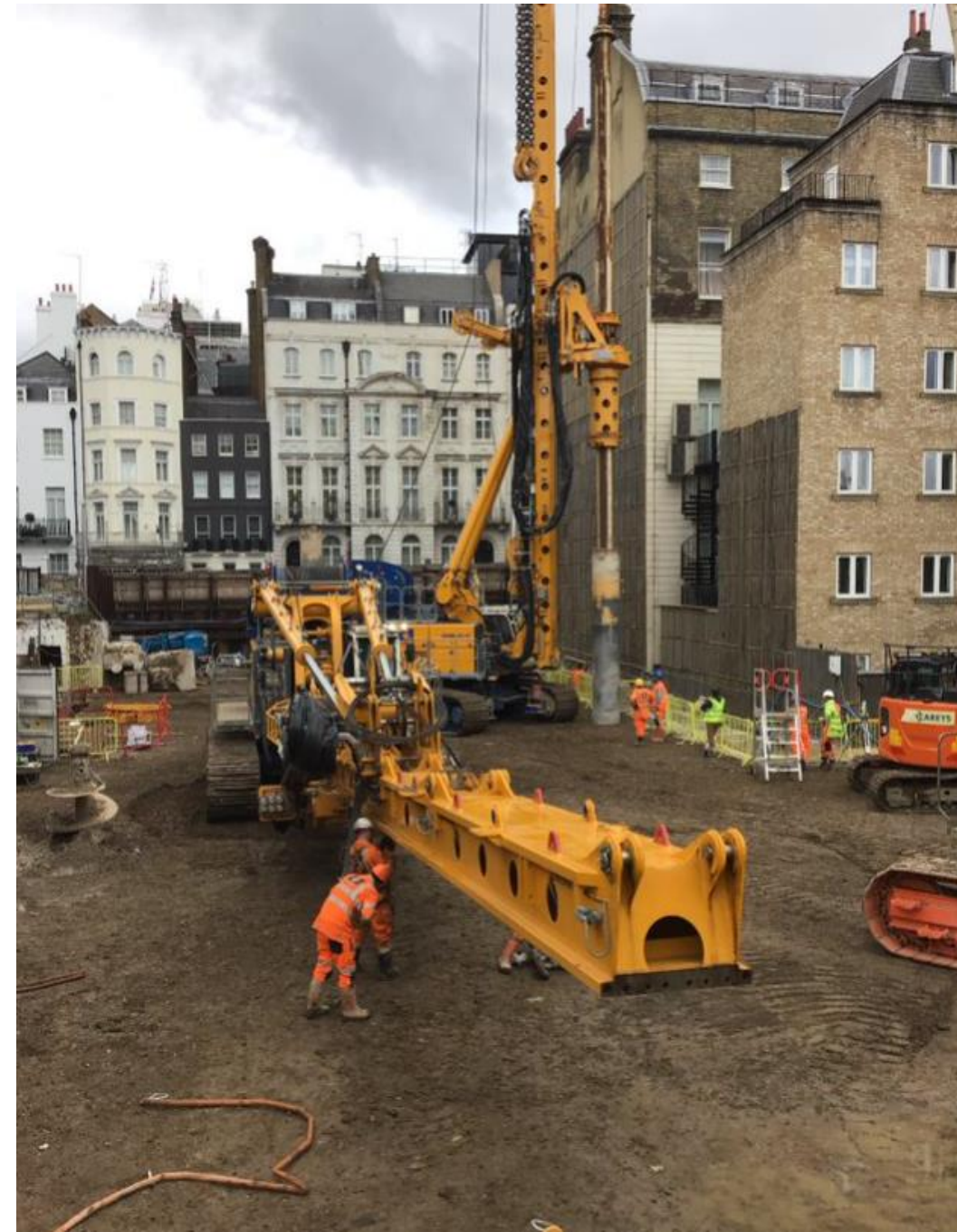
Building of Rig 2
