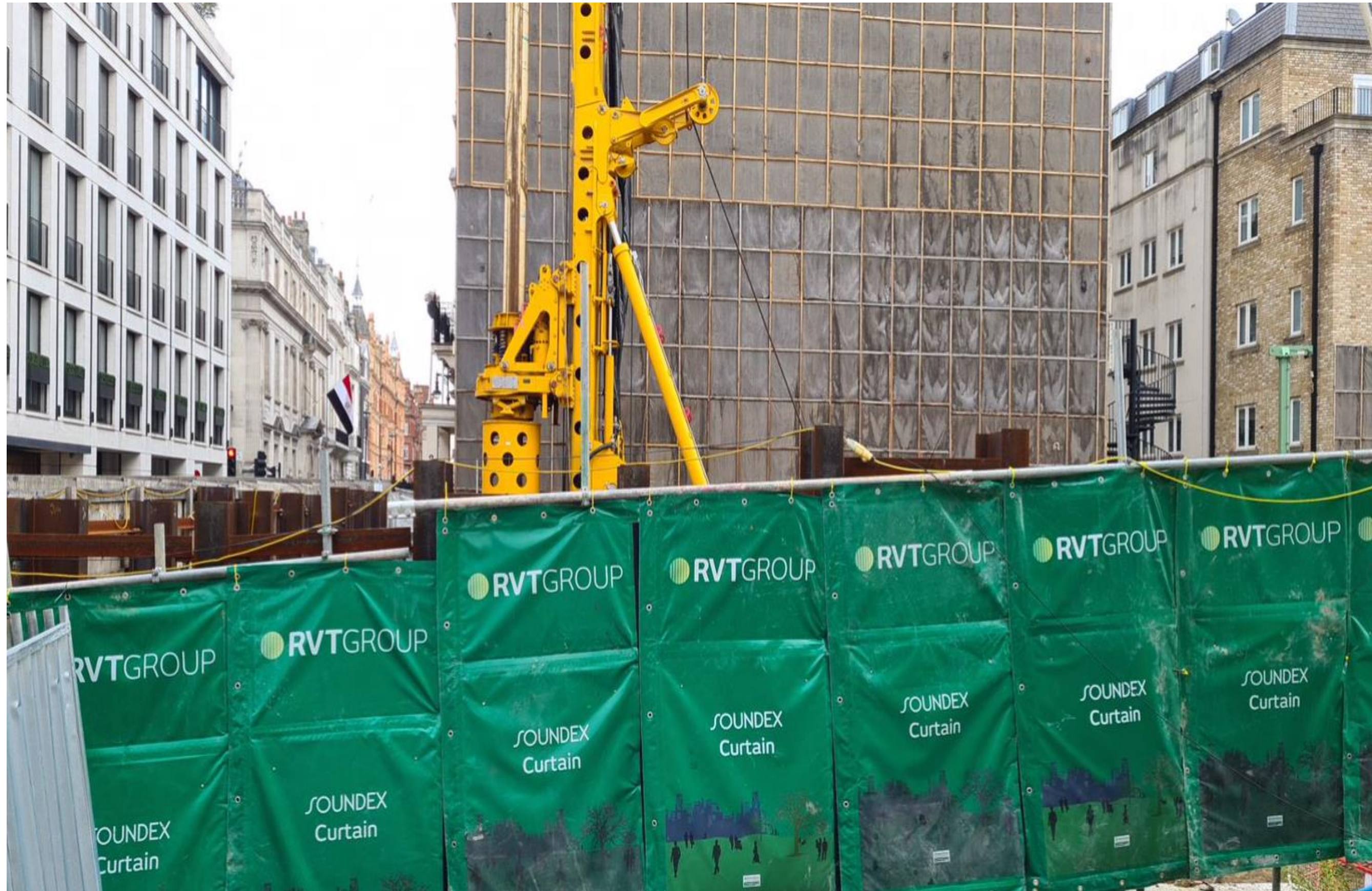
Existing Pile Coring Works In Action (Inc Noise Barriers)
